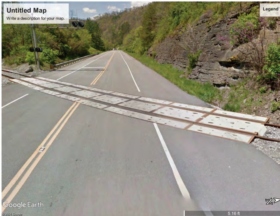
EXAMPLE OF NEW CROSSING WITH CONCRETE PANEL
