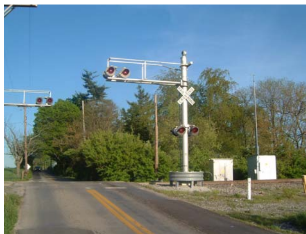
An example of an active warning system with flashing lights and bells along Brannon Road in rural Fayette County
