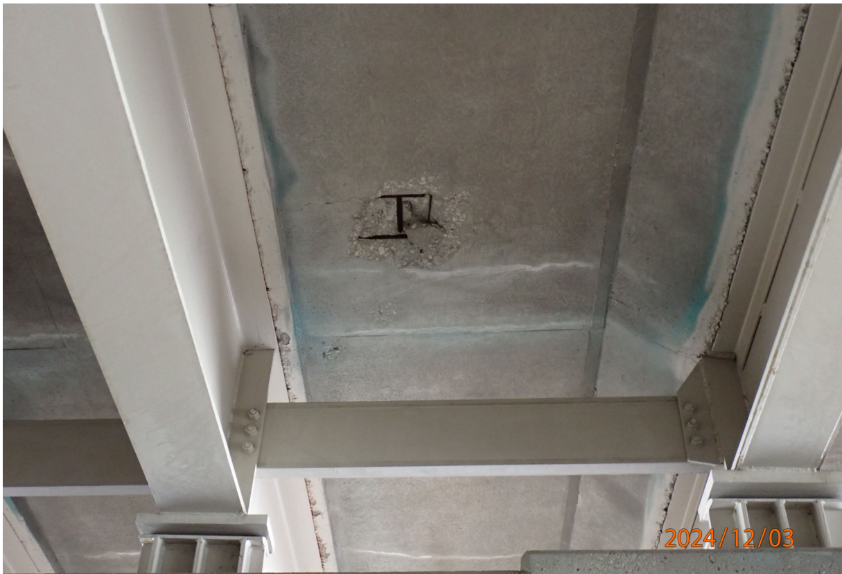
Large deck soffit spall with exposed rebar in Bay 13 of Span 1 near Pier 2.
