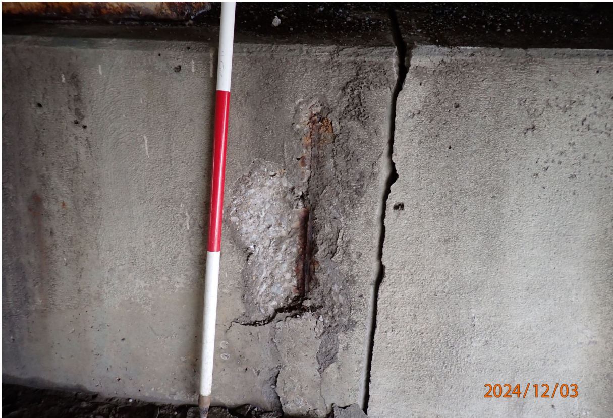
Abutment 1 spall with exposed rebar below Beam 3.
