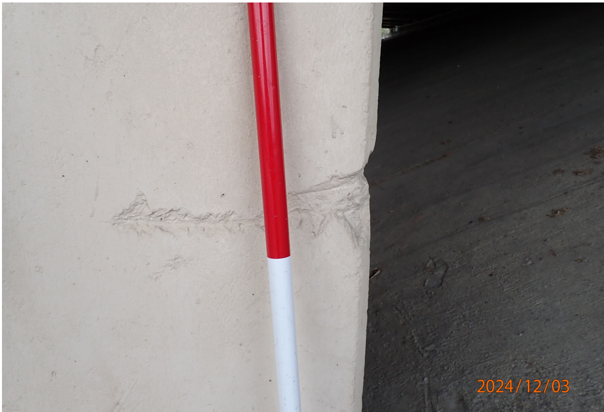
Pier 3-Column 9 spall.
