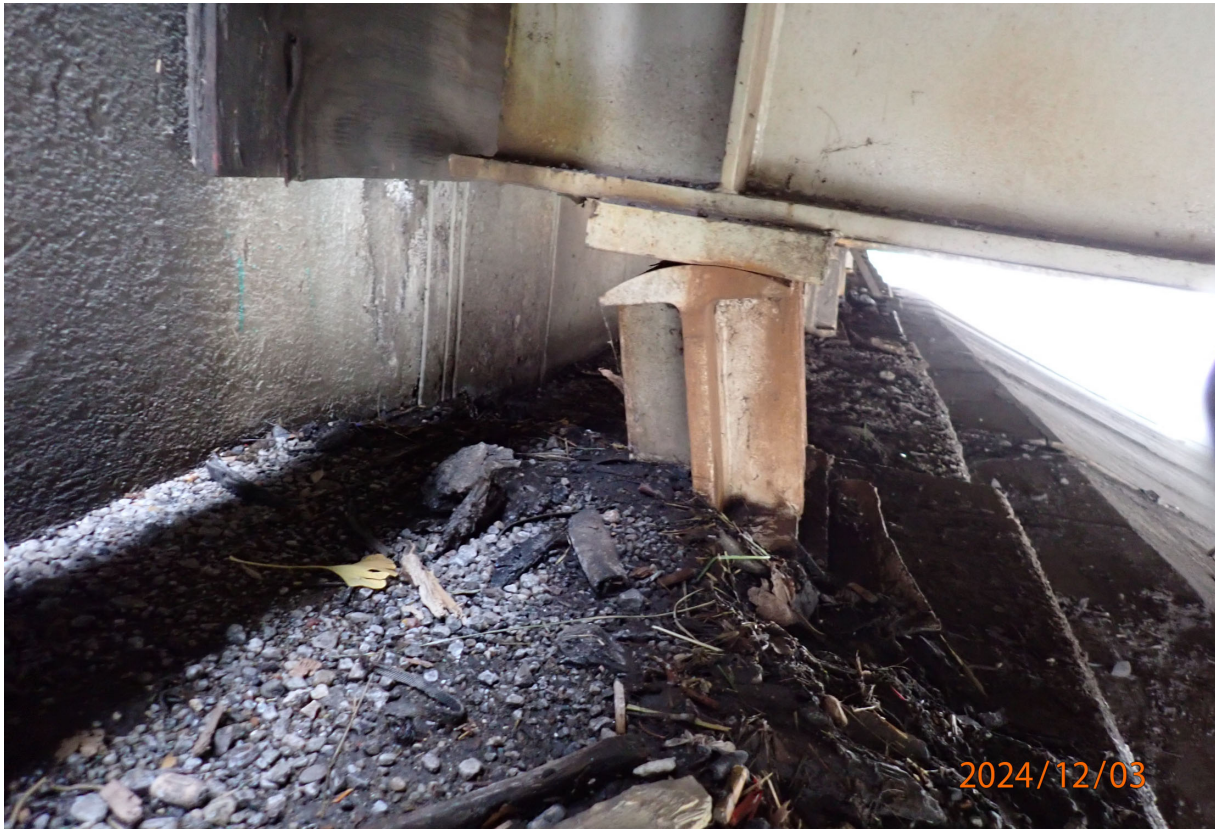
Abutment 1 bearings are over-expanded.
