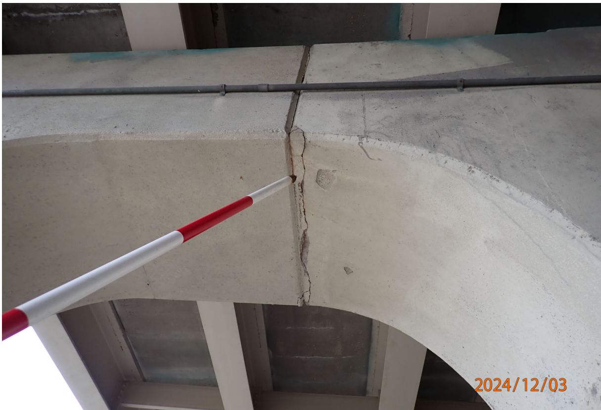
Pier 3 cap has a wide crack between Columns 1 and 2.
