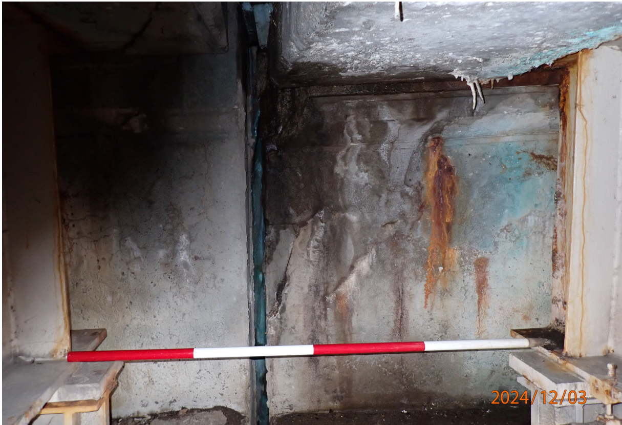
Abutment 4 moderate cracking with rust staining below the longitudinal joint.
