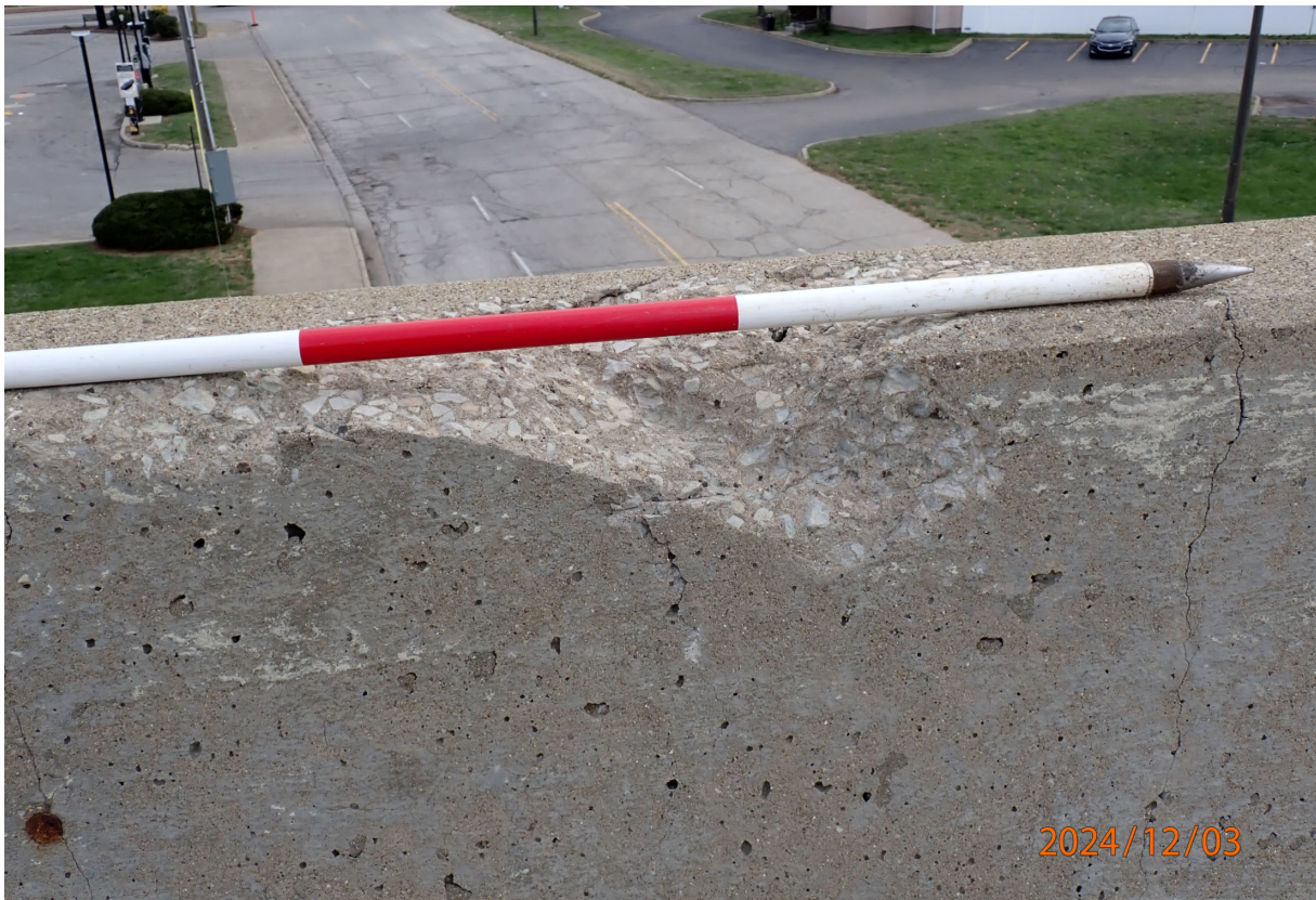
East barrier has a few impact spalls.
