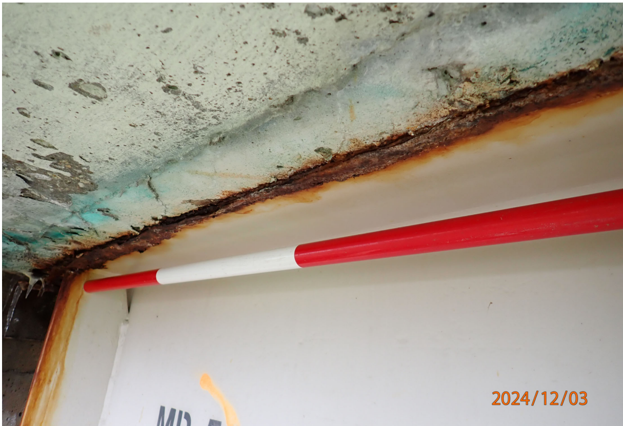
Beam 1 at Abutment 4 with corrosion along the top flange.
