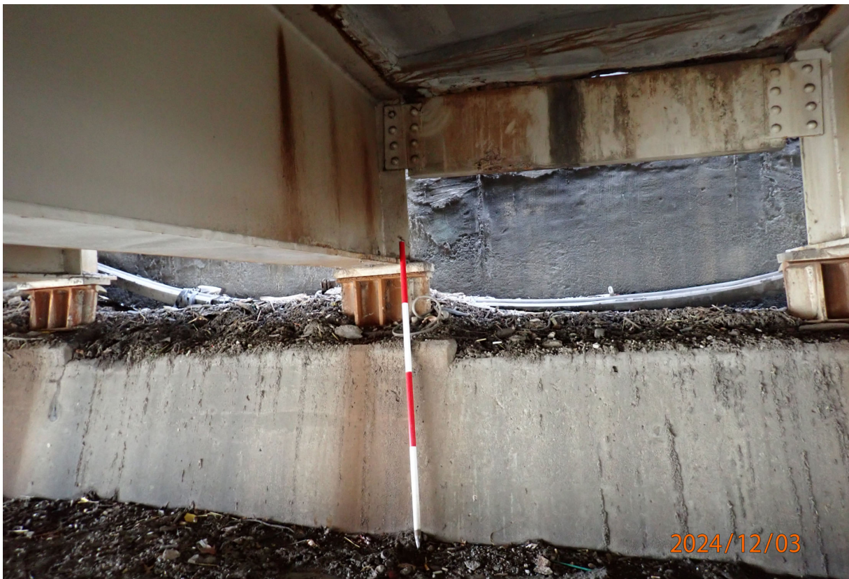
Abutment 1 has heavy debris on the cap, especially near the east end.
