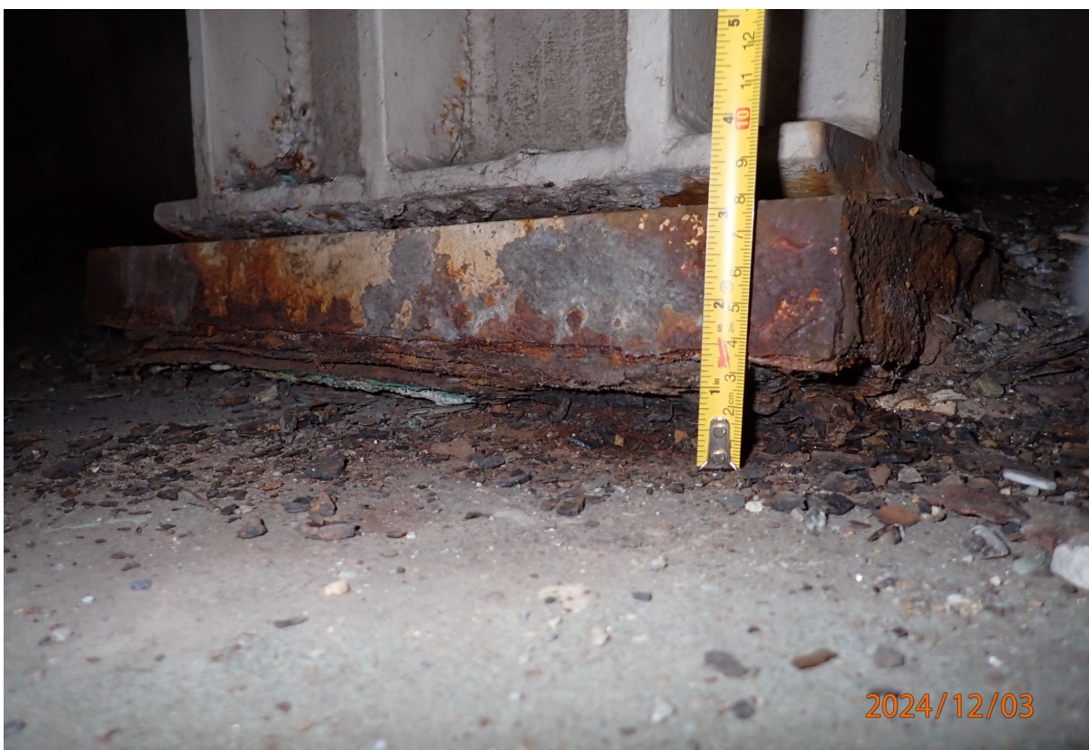
Some of the masonry plates at Abutment 1 no longer sit flush on the abutment seat due to extensive pack rust.
