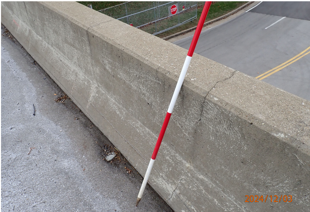
Typical barrier vertical cracking.
