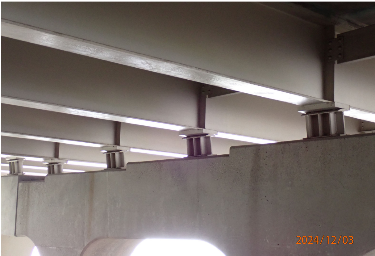
Typical expanded Pier 2 bearings.
