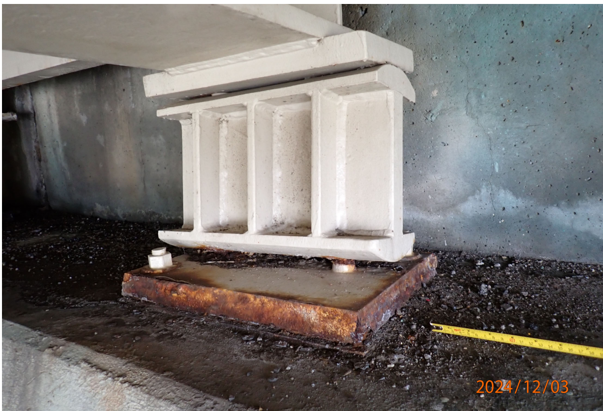
Abutment 1 bearings have corrosion, many with section loss.
