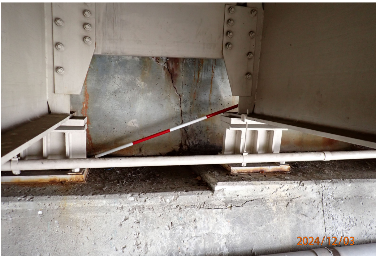
Abutment 4 backwall wide vertical crack in Bay 19.
