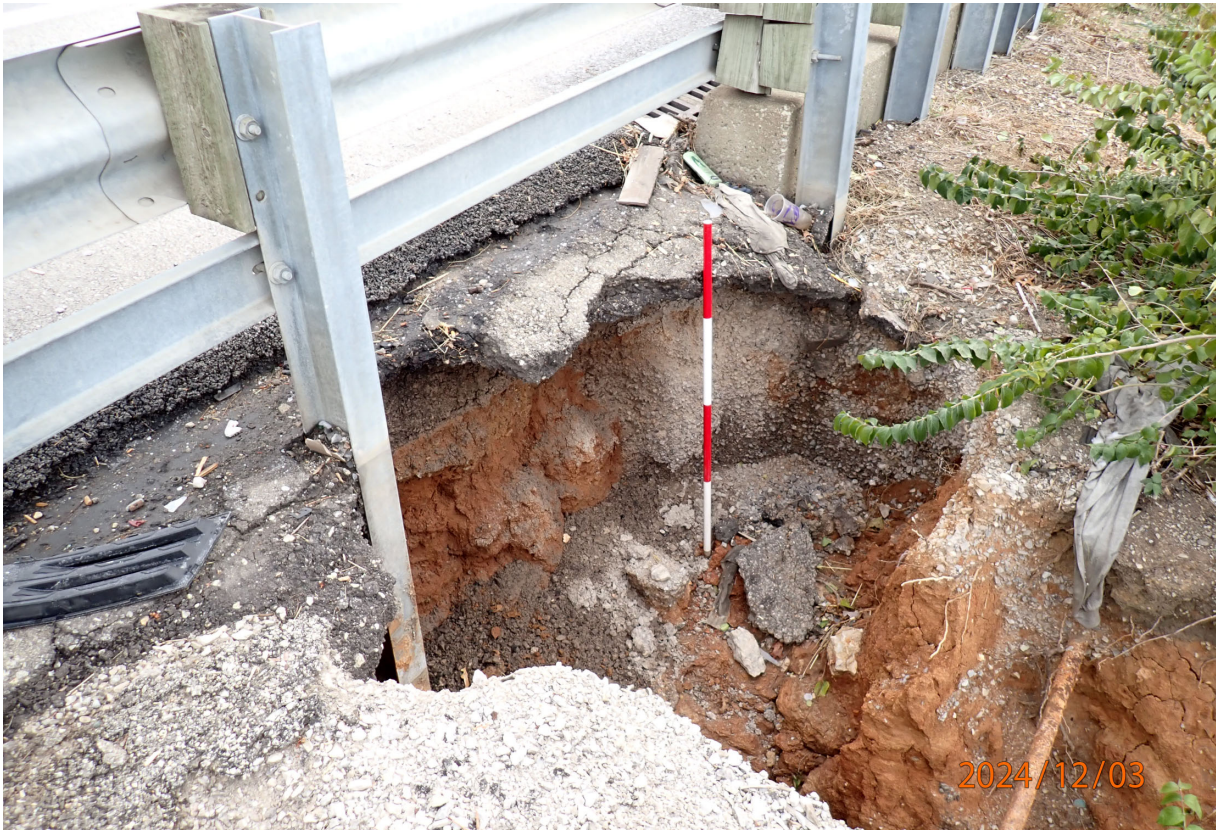
NW embankment has a large erosion hole along the roadway shoulder.
