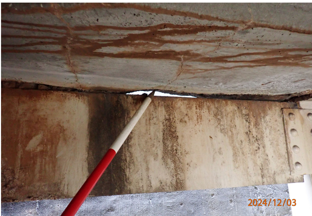
The underside of the deck adjacent to the Abutment 1 joint has spalling with exposed rebar, especially from Bays 15 through 17. Bay 15 shown.
