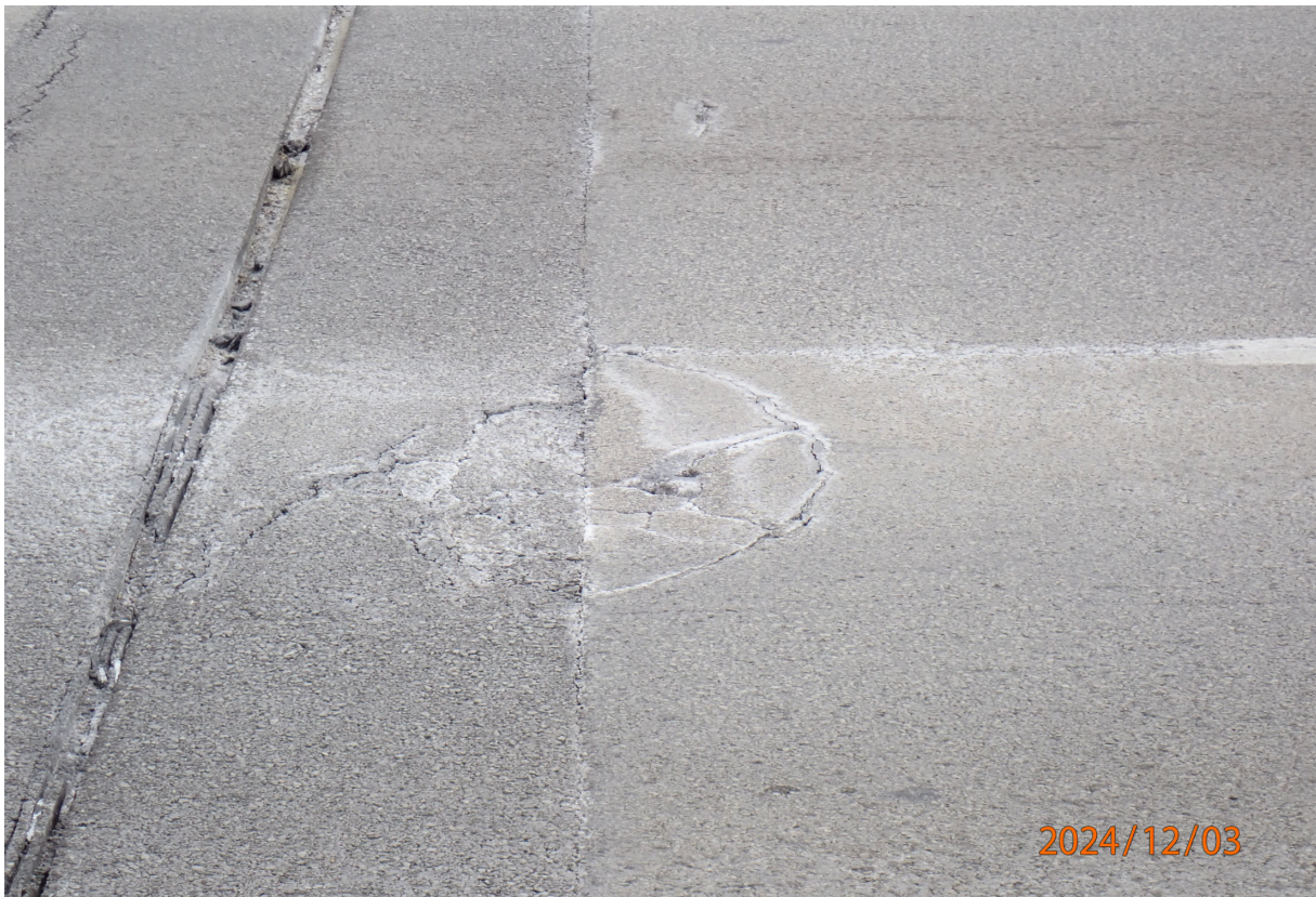
Asphalt overlay has cracking in the SB right lane at the north bridge end.
