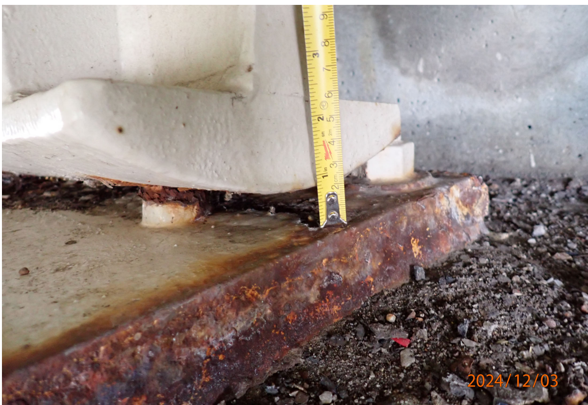
Several beam sole plates at Abutment 1 are not fully bearing on the rocker bearings and bang under live load. Beam 2 shown.
