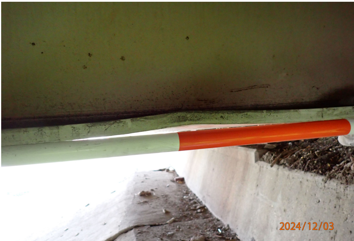
Beam 17 has distortion in the bottom flange near Abutment 1.
