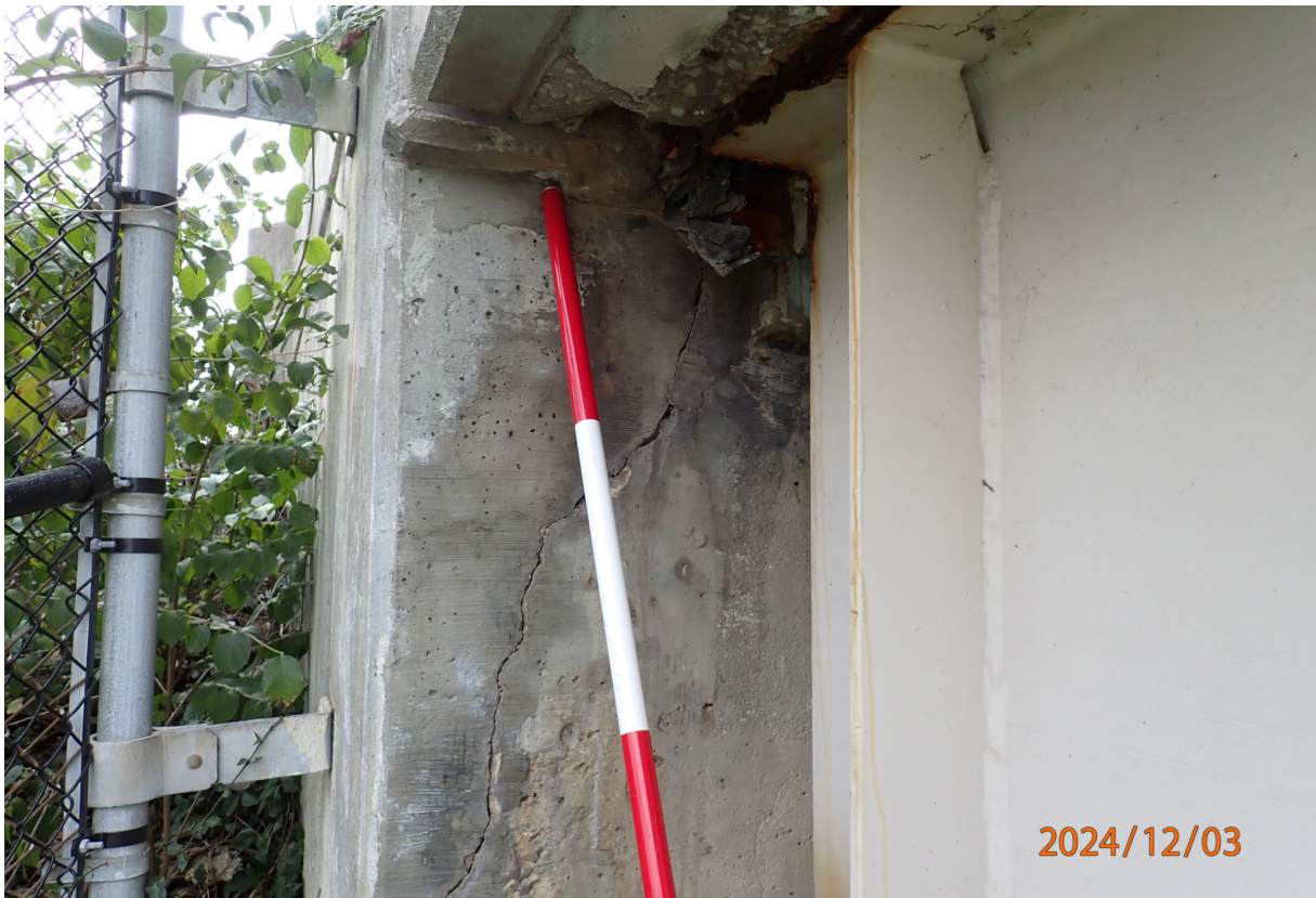
Abutment 1 backwall has moderate to wide diagonal cracks at the ends.
