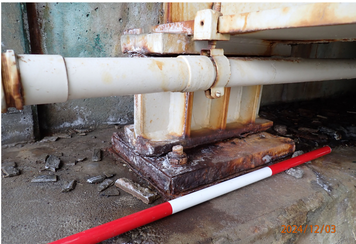
Typical Abutment 4 bearing with corrosion.
