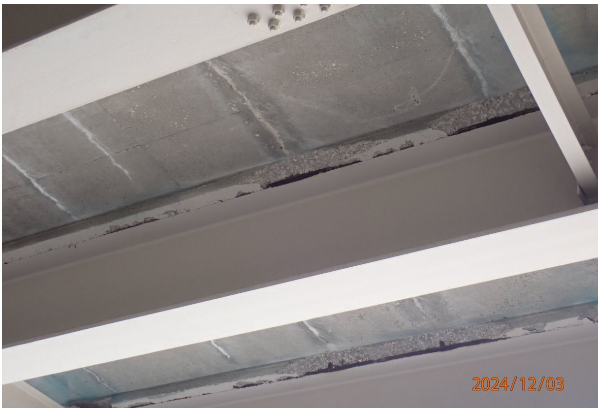
Underside of the deck has several haunch spalls along the beam top flanges.
