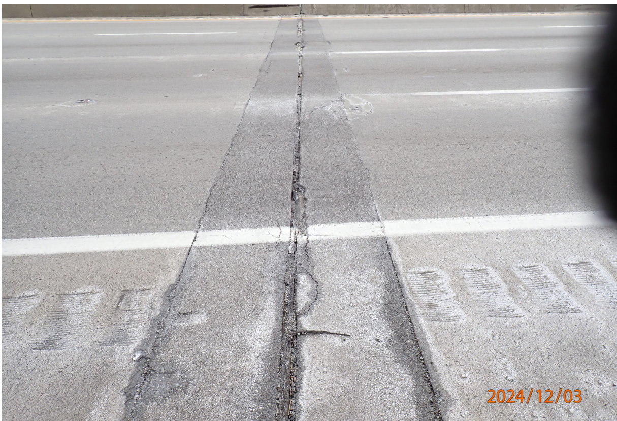
North bridge joint over Abutment 4 for SB traffic.
