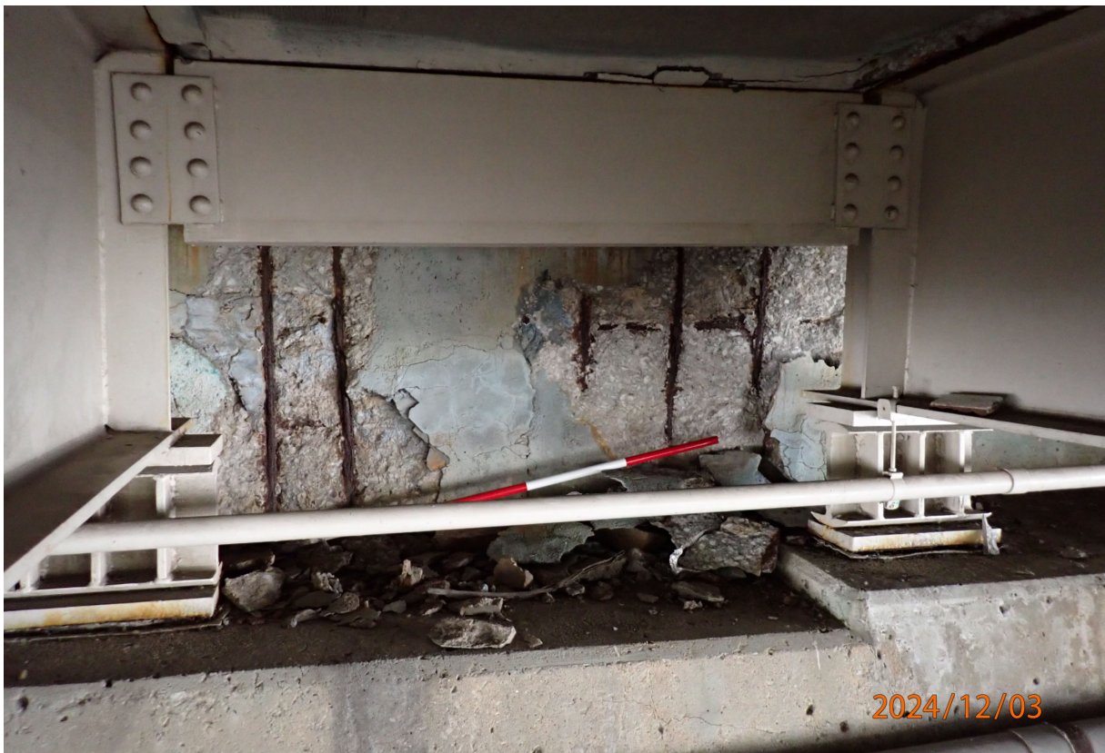
Large area of unsound patching and spalling with exposed rebar in Bay 14 of Abutment 4.
