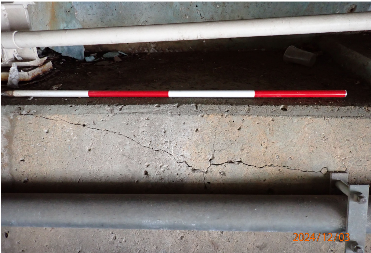
Abutment 4 cap has wide horizontal cracks in the front face. Bay 15 shown.
