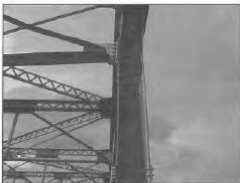
Figure B-15—Sway Bracing Impact Damage in Span 1
