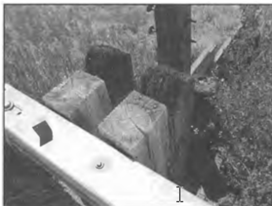
Figure B-5-Decay in Timber Rail Posts
