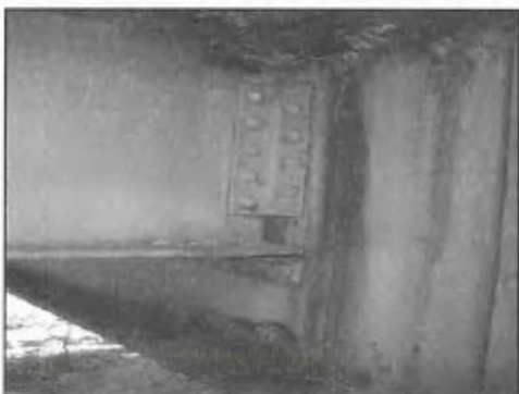
Figure B-17—Corrosion at Floor Beam Ends
