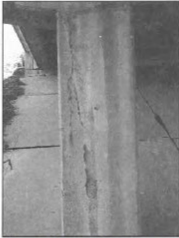
Figure B-12— \frac{2}{16} -in. Width Vertical Crack in Left Column of Pier 4
