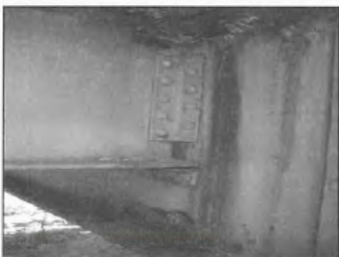
Figure B-17—Corrosion at Floor Beam Ends
