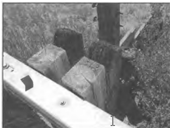
Figure B-5-Decay in Timber Rail Posts
