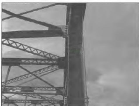
Figure B-15—Sway Bracing Impact Damage in Span 1
