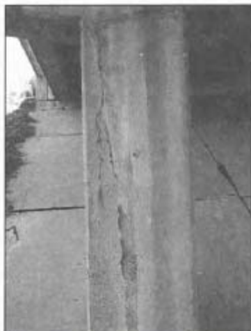
Figure B-12— \frac{3}{16} -in. Width Vertical Crack in Left Column of Pier 4
