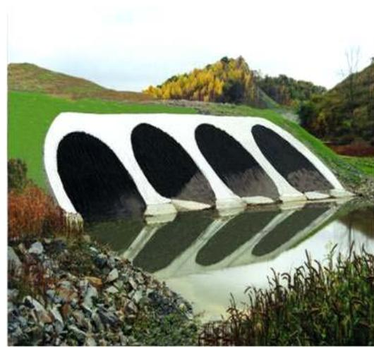
**Examples of mitered culvert design**
