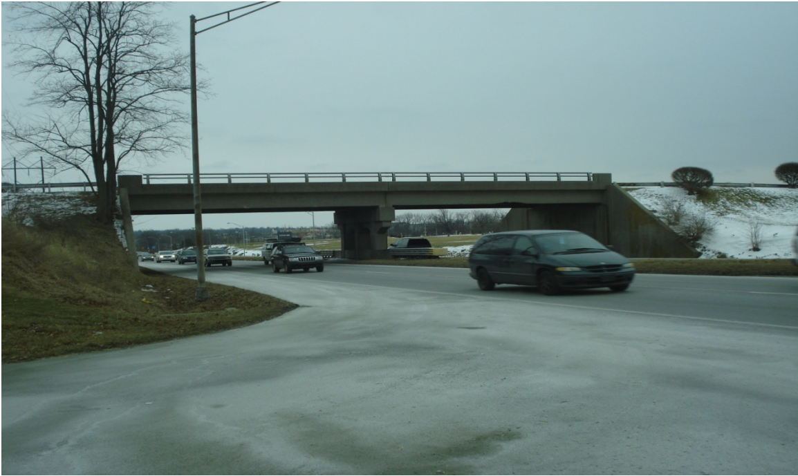
EXISTING LEXMARK BRIDGE SHOWING PIER AND VERTICAL ABUTMENTS
