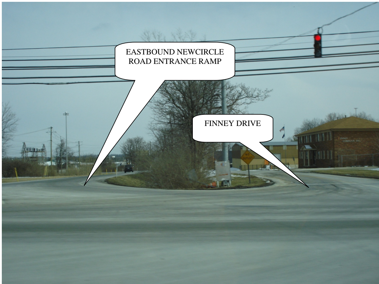
EXISTING CONDITIONS IN GEORGETOWN ROAD/ NEW CIRCLE ROAD INTERCHANGE
