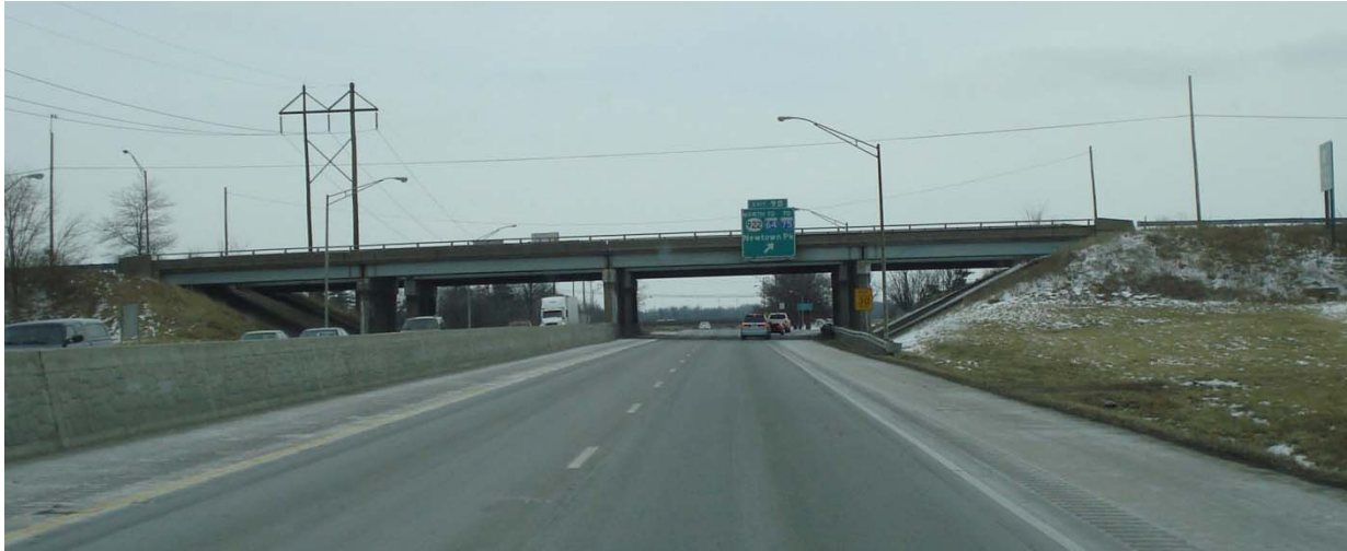
EXISTING TWIN STEEL BEAM BRIDGES OVER NEW CIRCLE ROAD
