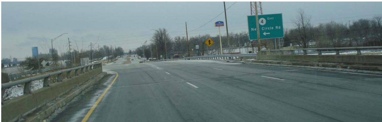
EXISTING SOUTHBOUND NEWTOWN PIKE BRIDGE OVER NEW CIRCLE ROAD
