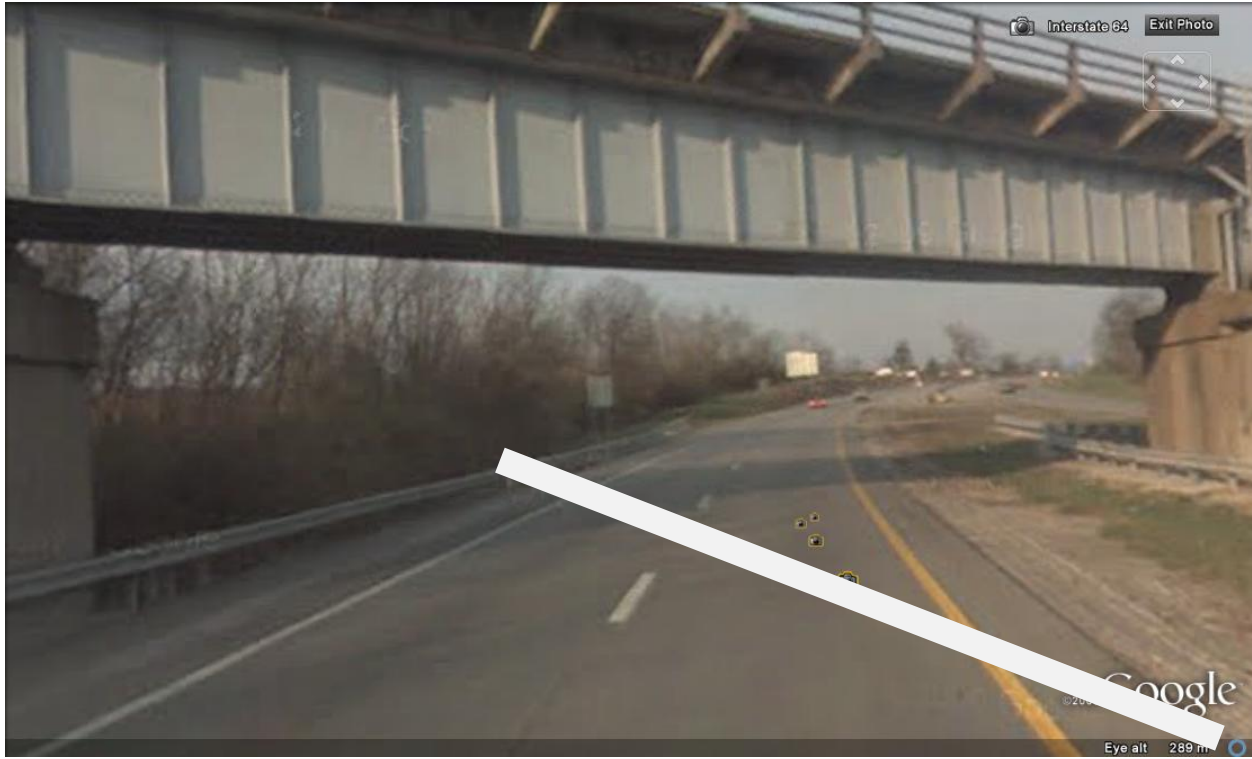
AS PROPOSED LOCATION OF 16' x 3' RCBC UNDER RJ CORMAN RR BRIDGE (Looking west)
