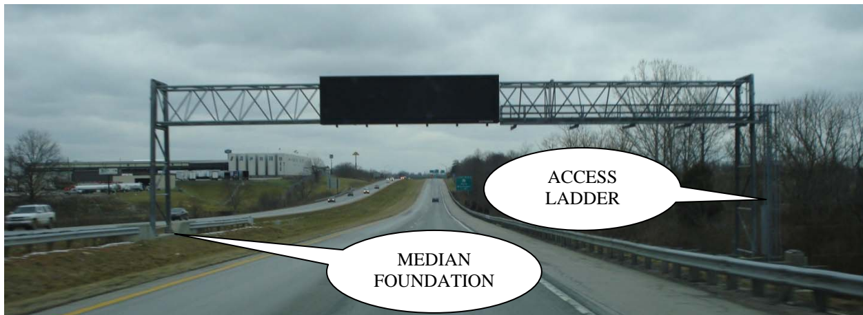
EXISTING ITS SIGN TRUSS SUPPORT
