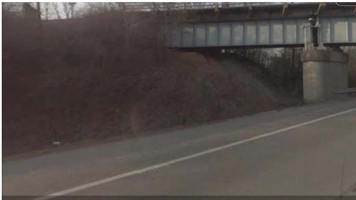
SOUTH SPAN OF RJ CORMAN RR BRIDGE STA 1315+50 (+/-)
