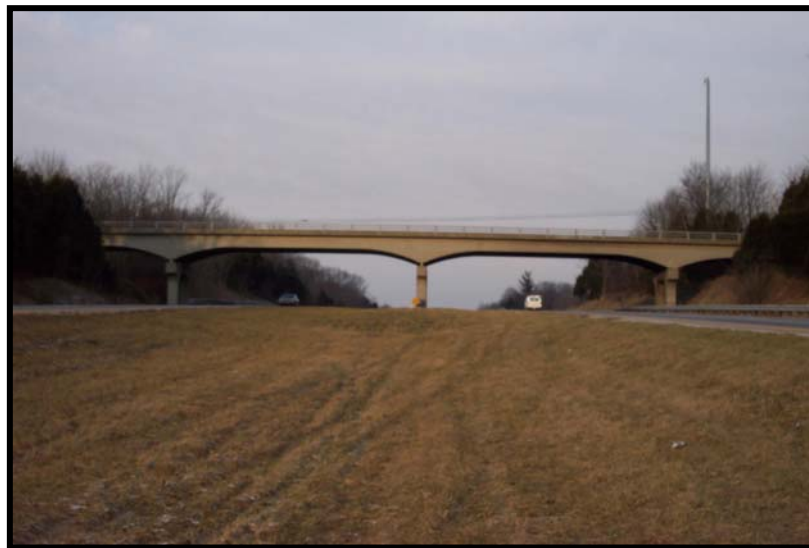
EXISTING CLARK STATION ROAD OVERPASS
