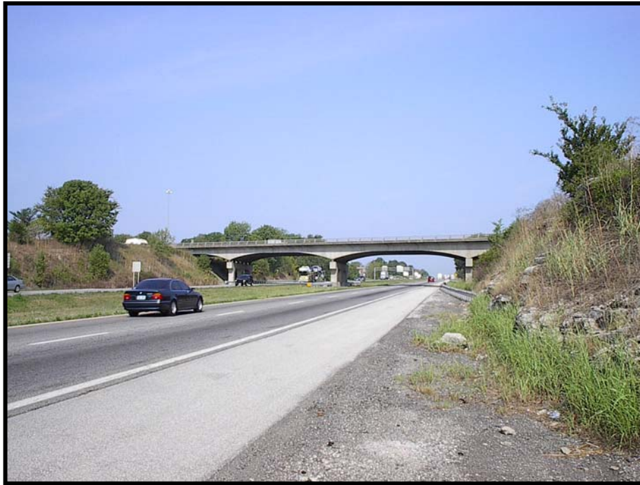
EXISTING KY 55 INTERCHANGE OVERPASS
