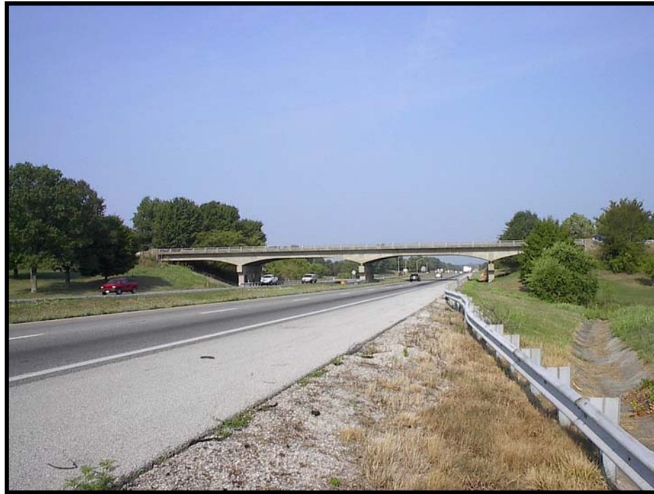
EXISTING KY 53 INTERCHANGE OVERPASS
