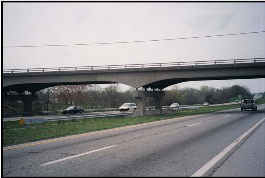
EXISTING JOYES ROAD OVERPASS
