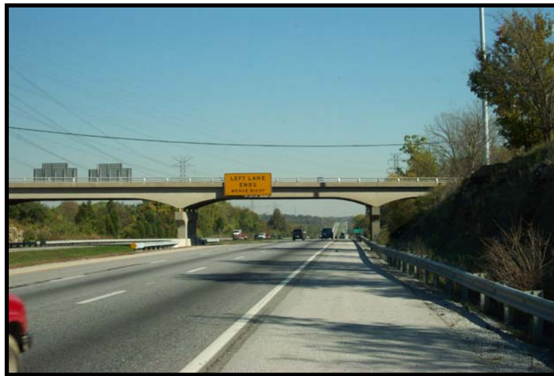
EXISTING ENGLISH STATION OVERPASS
