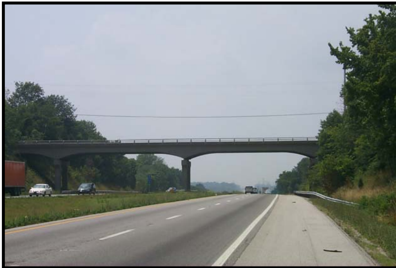
EXISTING GILLILAND OVERPASS
