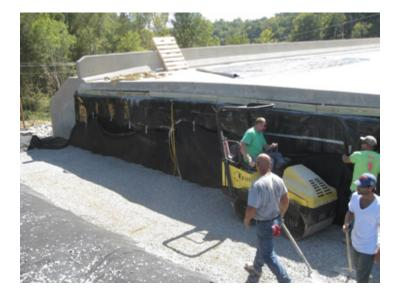
abutment and installed prior to placing the fabric and rock layers. The elasticity of the foam block allows for expansion and contraction, which creates a tight fit between the abutment and the road, thus preventing water from penetrating between the bridge and the road.
