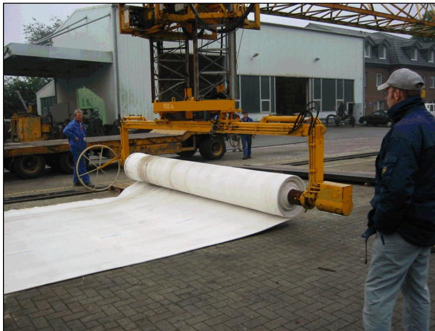
Figure 11.18. SandMat™ geocomposite blanket being unrolled.
