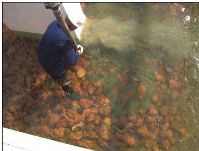
Figure 12.11. Underwater partial grouting of riprap.
