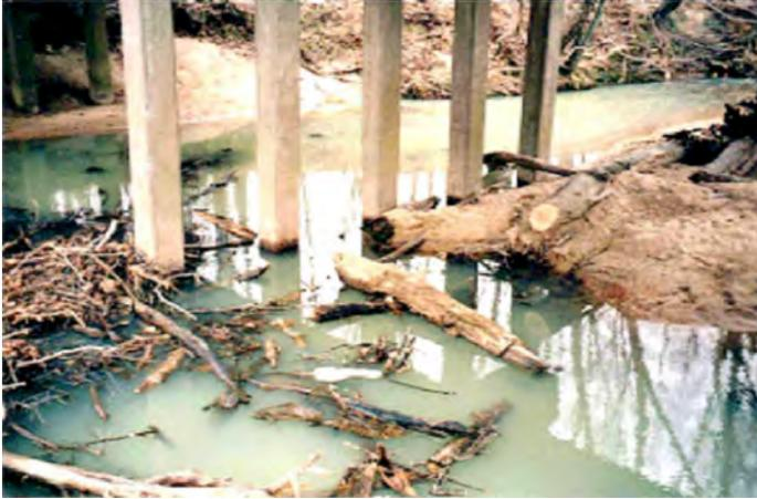
Figure 19.5a. Scour hole debris at Bridge 133, Graves County, KY
