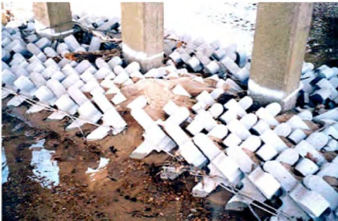
Figure 19.5c. Close-up of armor units after several flow events at Bridge 133, Graves County, KY
