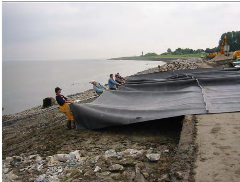
Figure 12.17. Hand placing geotextile prior to placing partially grouted riprap.
