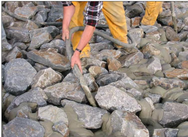
Figure 12.20. Grout placement by hand.
