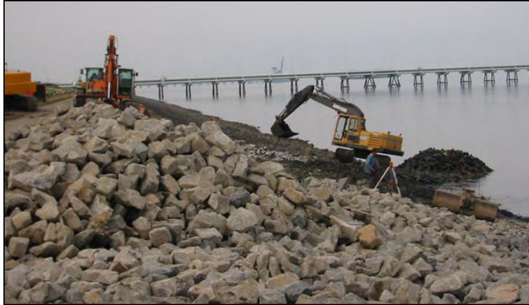
Figure 12.18. Placing riprap with hydraulic excavators.
