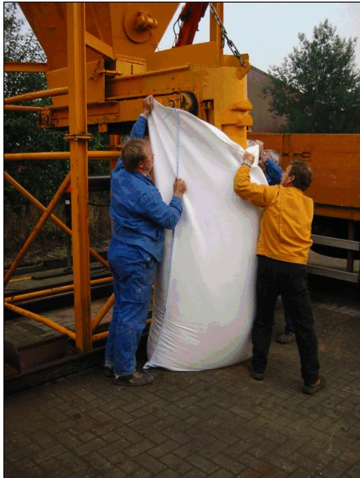
Figure 11.19. Filling geotextile container with sand.
