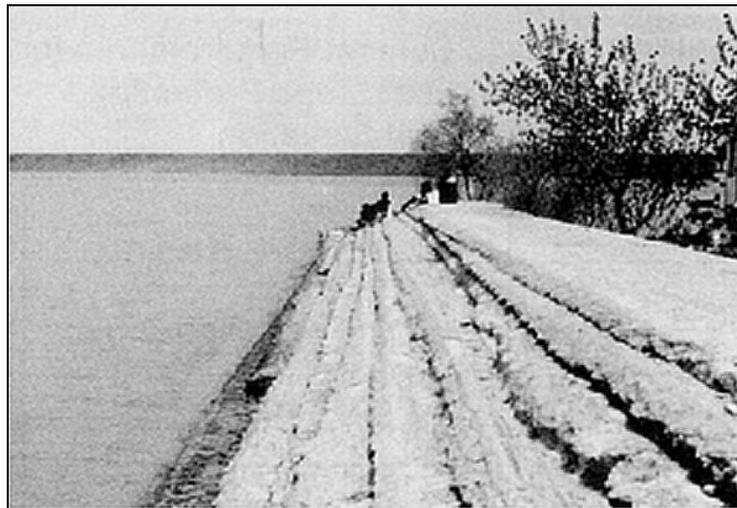
Figure 7.1. Stair step facing on Bonny Reservoir, Colorado after 30 years (PCA).
