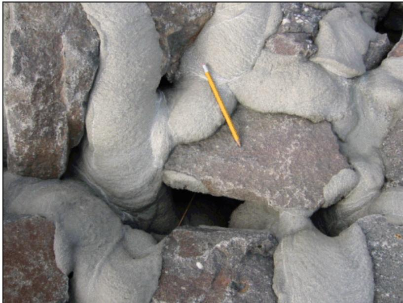
Figure 12.1. Close-up view of partially grouted riprap.
