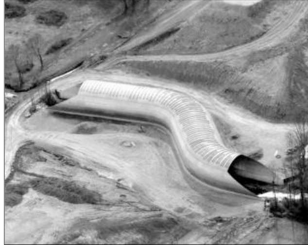
Figure 5.3. Culvert with a horizontal bend (Contech).
