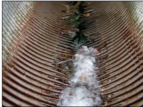
Figure 2.12b. Corrosion issues in a culvert.
