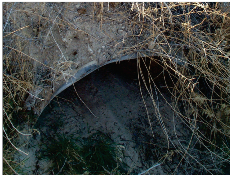
Figure 5.12. Excessive sediment deposition in culvert.
