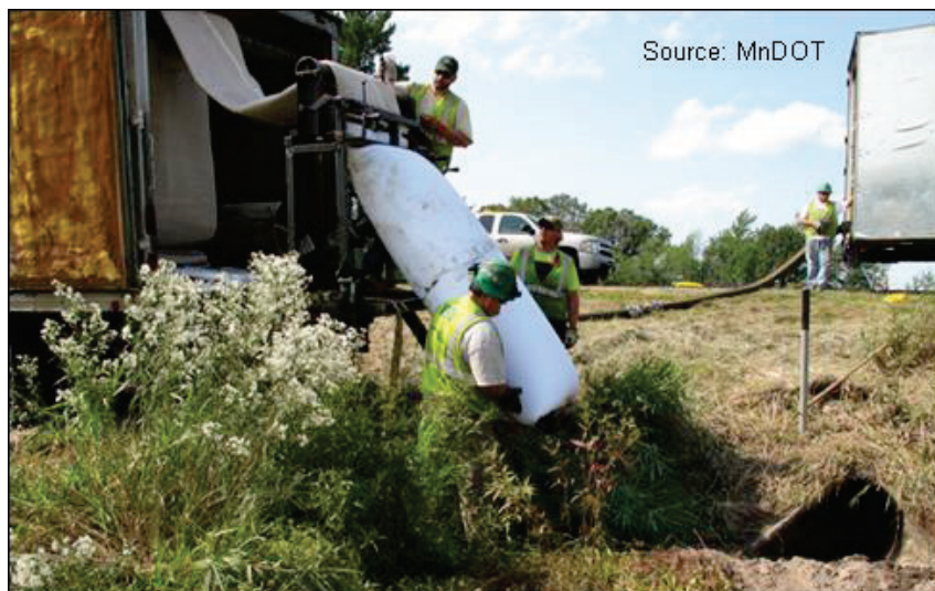
Figure 6.14. Cured-in-place liner installation.
