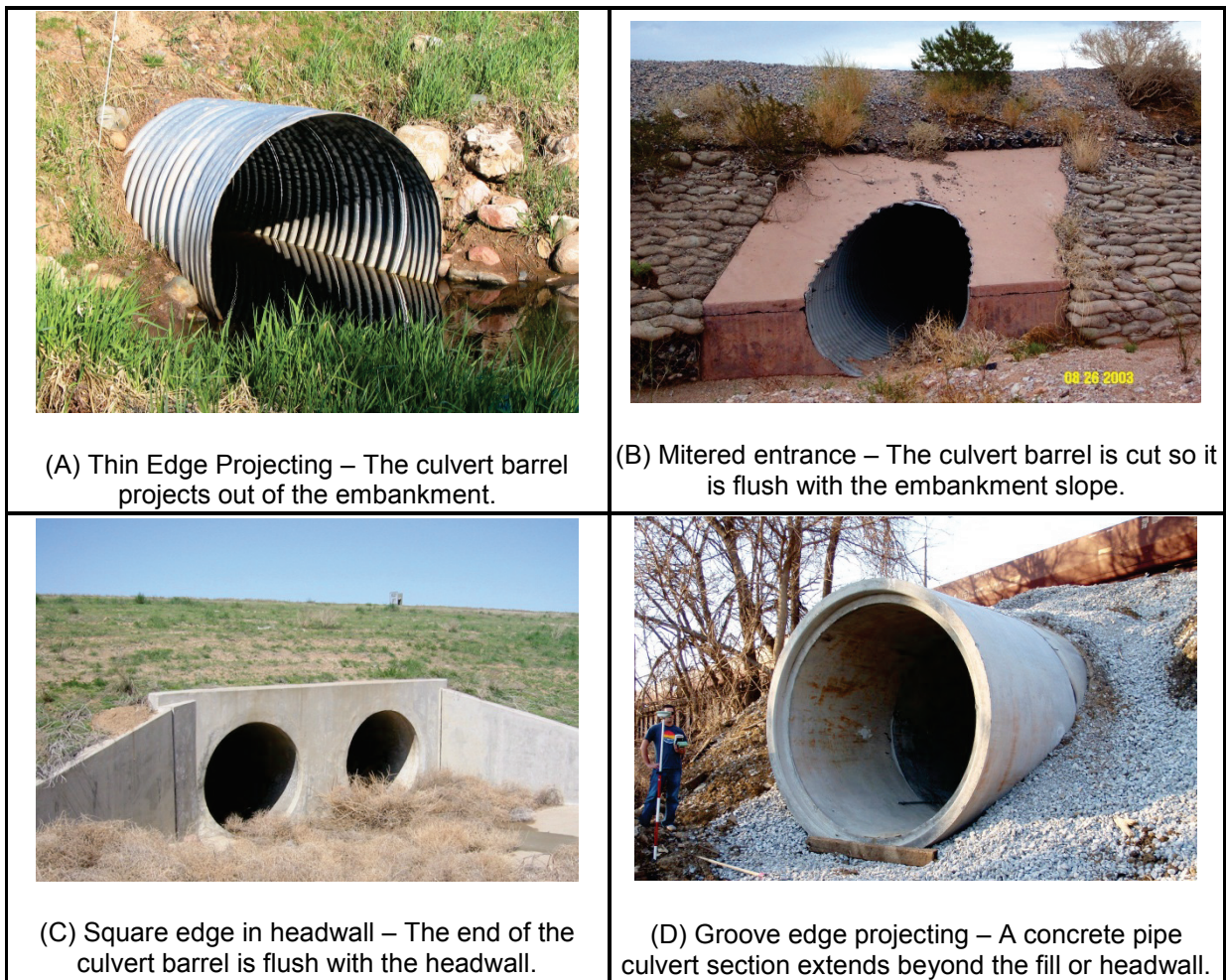
Figure 3.2. Typical inlet configurations.
