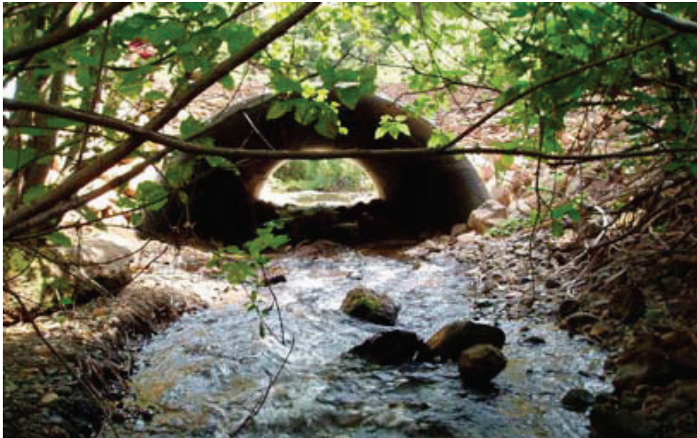
Figure 4.4. Completed open-bottom installation (from USFS 2008).
