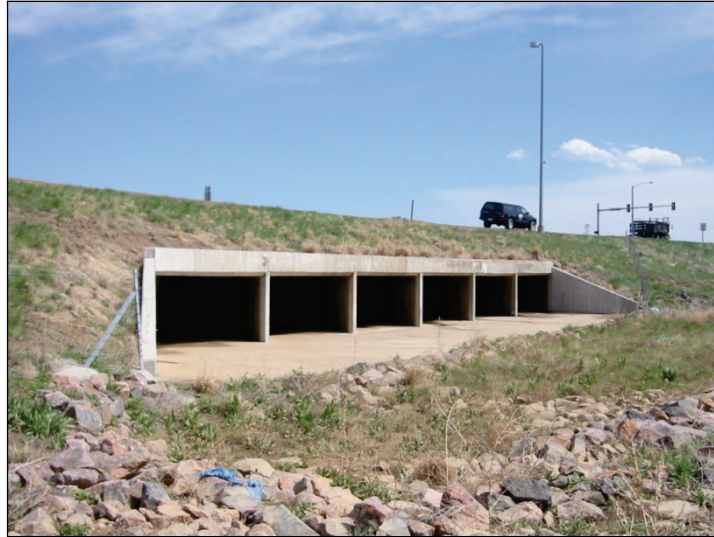
Figure 5.17. Multiple barrel box culvert.
