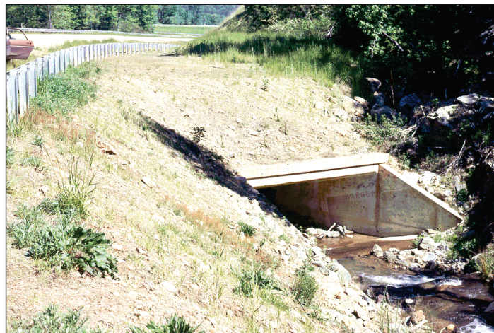
Figure 5.16. Fill warped to avoid inlet skew.
