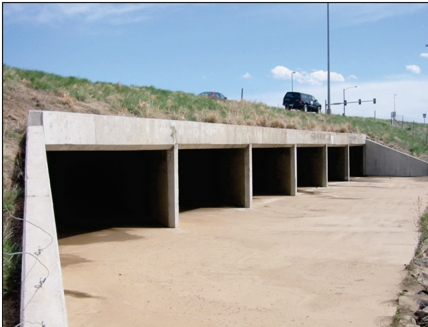
Figure 1.21. Multi-cell box culvert.
