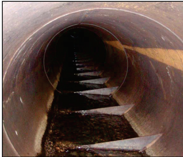
Figure 5.7. Angled baffles (from FishXing Users Manual).
