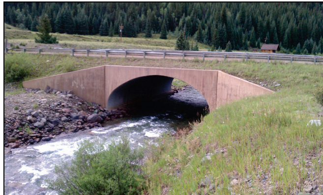
Figure 1.11. Open-bottom culvert.
