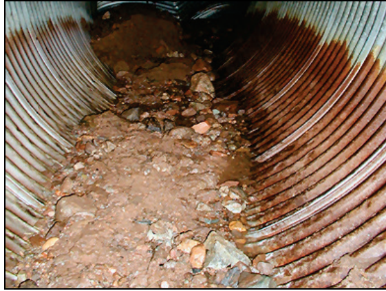
Figure 2.12a. Abrasion issues in a culvert.
