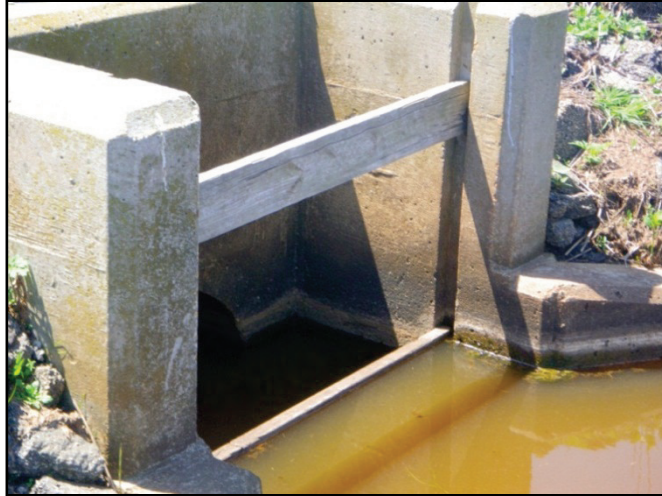
Figure 5.1. Culvert as outflow control device.
