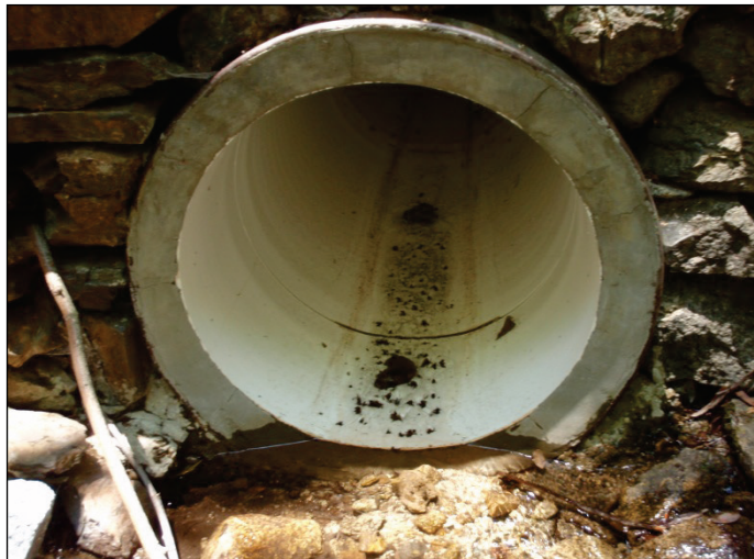
Figure 6.12. Slip lining a 30 inch (750 mm) CMP with a 24 inch (600 mm) PVC pipe.
