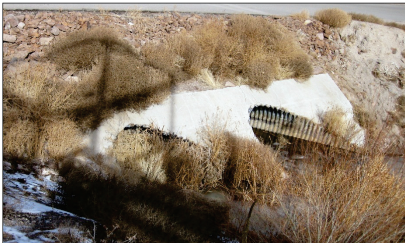
Figure 5.20. Slope paving around a mitered inlet.
