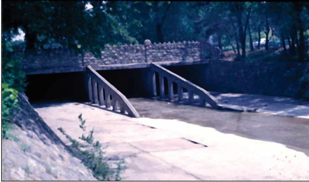
Figure 2.8. Concrete debris fins with sloping leading edge as extension of culvert walls.
