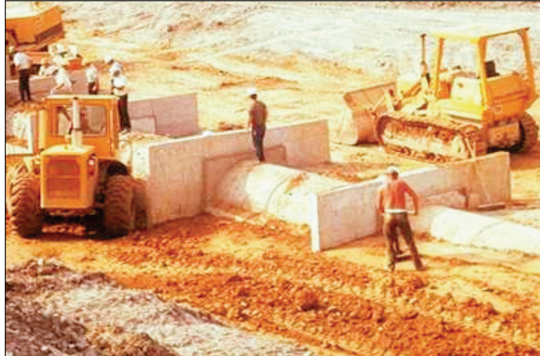
Figure 5.21. Anti-seep collars (FEMA 2005).
