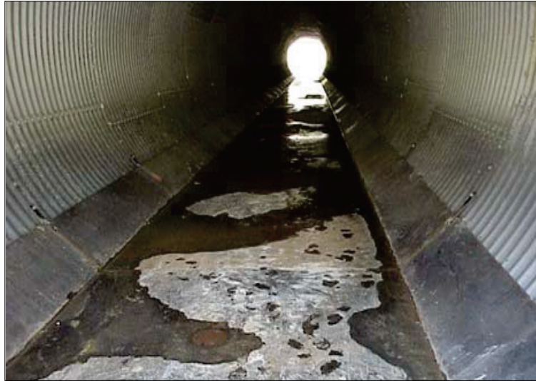
Figure 6.18. Invert repair of CMP using steel plating.
