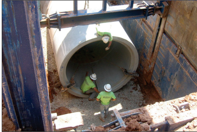
Figure 6.10. Open-trench excavation with shoring.
