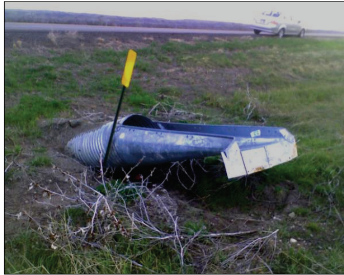
Figure 6.5. Buoyancy uplift.
