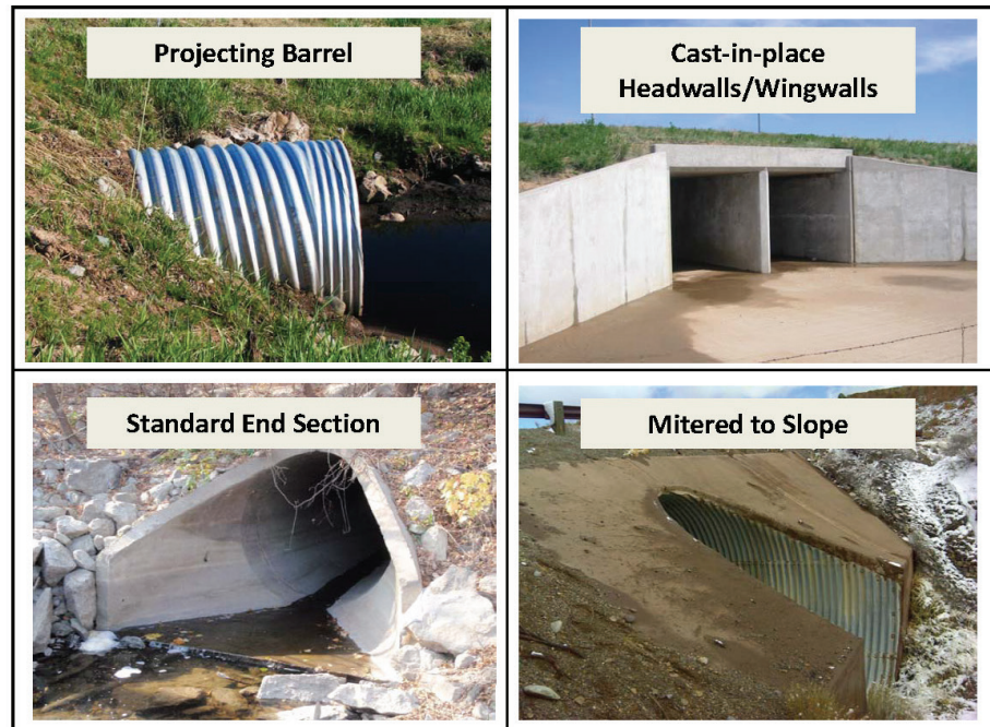
Figure 1.8. Four standard inlet types.
