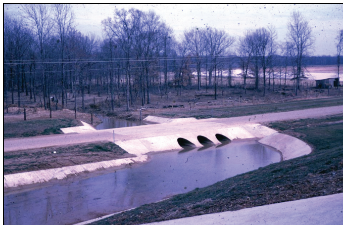
Figure 1.14. Vented low-water crossing.
