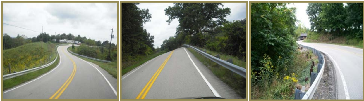
Figure 4: Alignment Deficiencies
