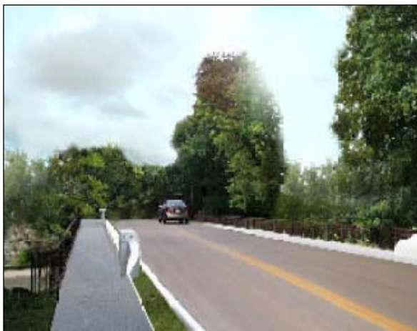
H. "After" Wolf Pen Branch Road bridge near Springdale Road, Prospect, KY (FEIS Selected and Modified Selected Alternatives).
