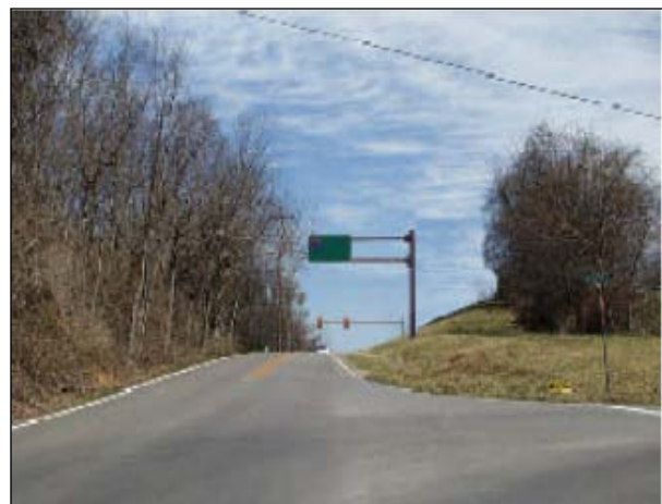
I. "After" Wolf Pen Branch Road bridge near Springdale Road with signalized intersection (FEIS Selected and Modified Selected)
