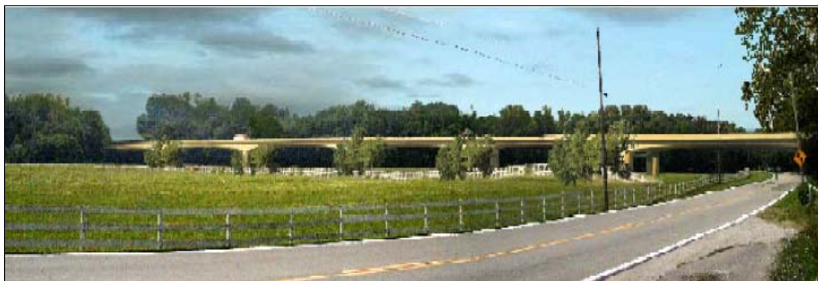
D. Prototypical view of approach on structure (FEIS Selected and Modified Selected Alternatives).
