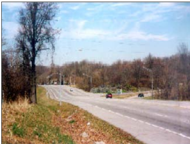
F. Modified Ramp Terminus at US 42 (FEIS Selected and Modified Selected Alternatives).
