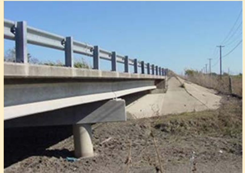
Type T6 Tubular W Beam
