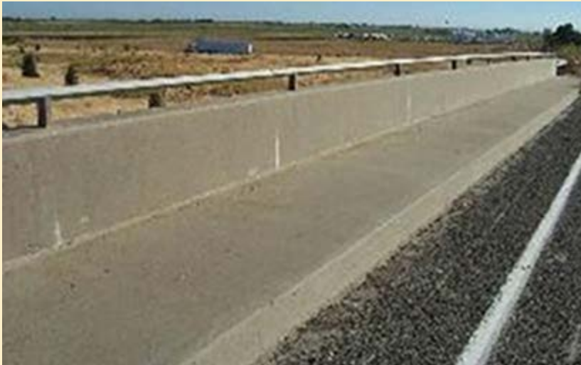
Type 26 Concrete Barrier with Sidewalk
