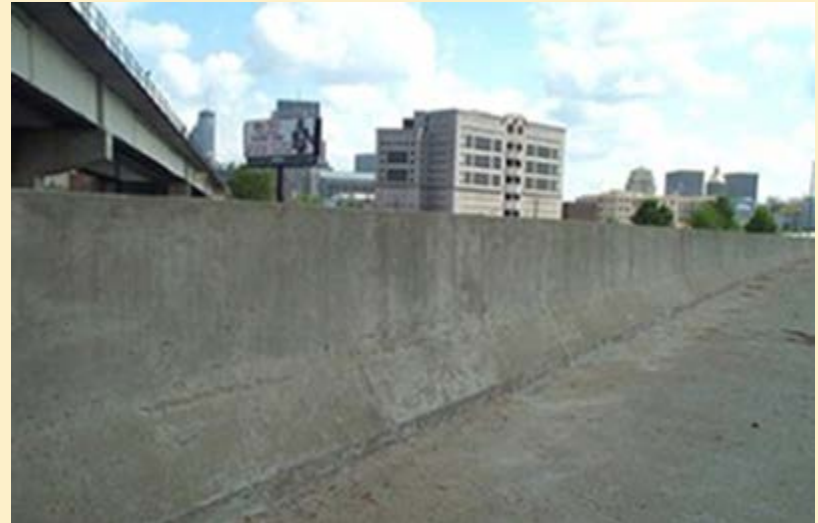
New Jersey Concrete Barrier
