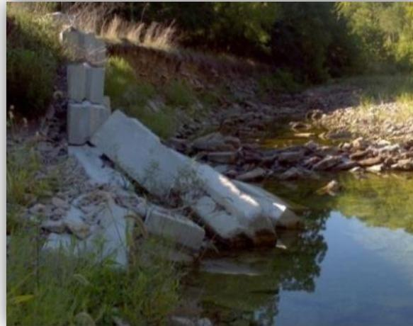
***Concrete blocks installed in an attempt to stabilize the stream bank near Duke Energy gas main***
