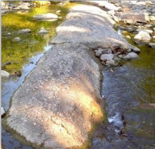
***Exposed sanitary sewer crossing upstream of Dry Creek WWTP***
