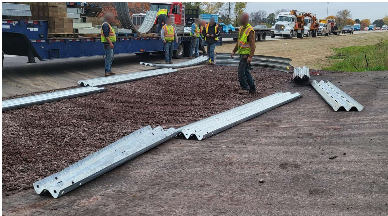
Figure 40 Beams Laid Out (Unassembled)
