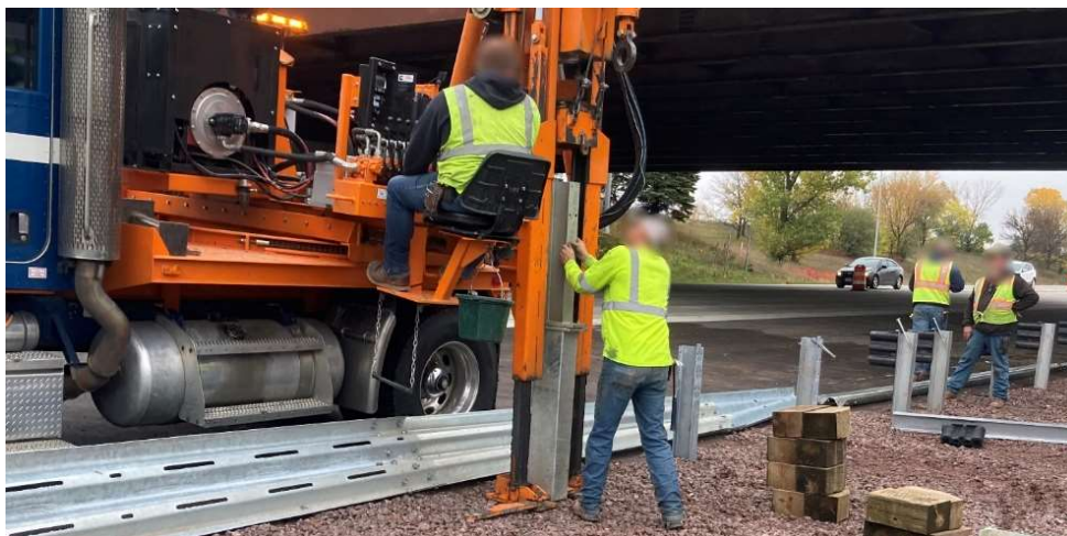
Figure 50 Driving UBSPs
