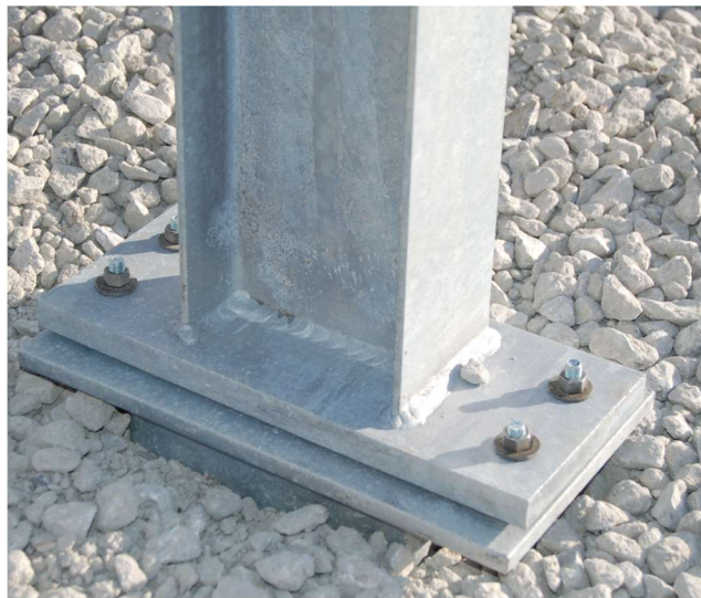
Figure 10 Assembled (Top) and Installed (Middle, Bottom) UBSPs
