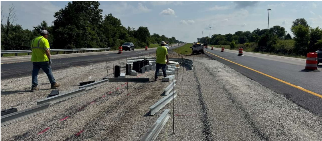
Figure 42 Beams E1, E2A, and E2B Connected to the System Layout The line string marks the back of posts for installation.
