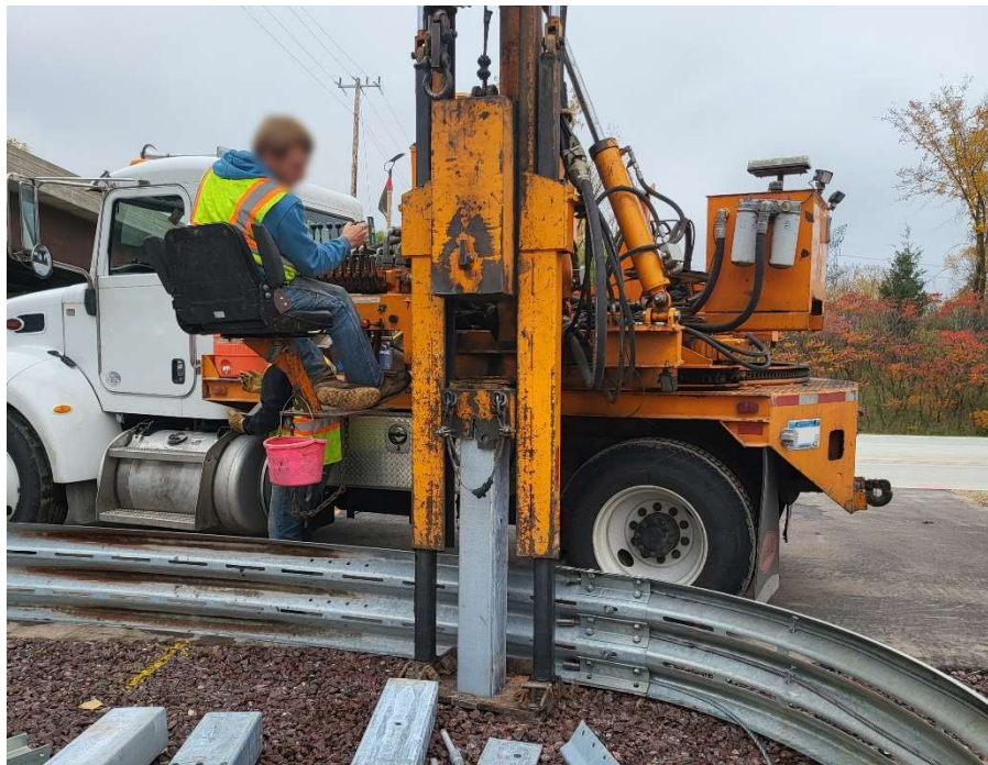
Figure 48 Driving BCT Foundation Tubes
