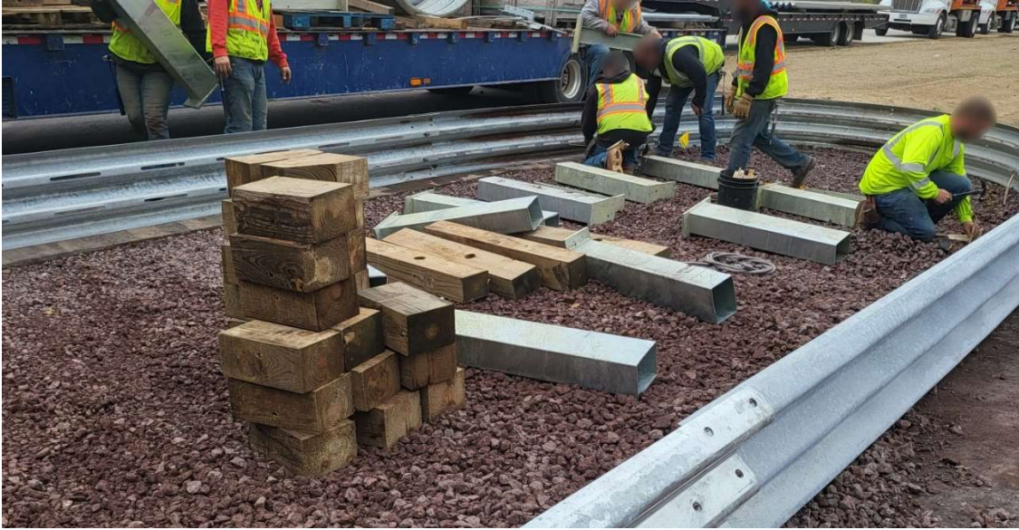
Figure 41 Beams Loosely Connected as a System Template
