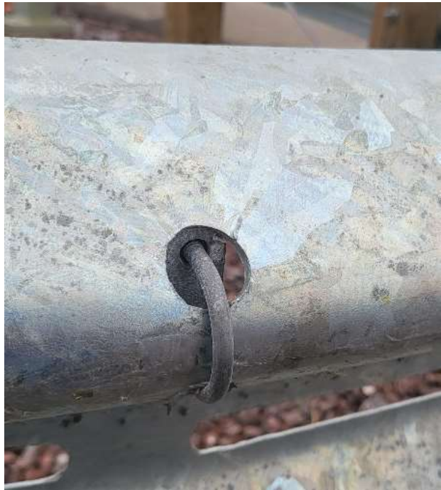
Figure 47 Nose Cable U-Bolt Orientation
