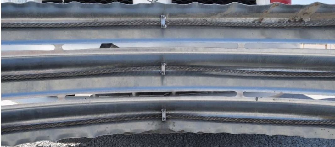
Figure 29 Cables Lining System Nose (Back View)
