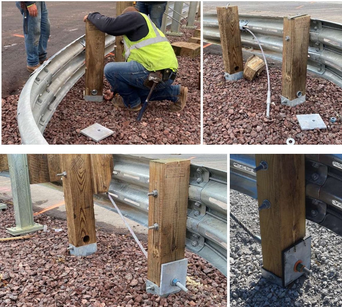
Figure 53 Cable Anchorage Installation
