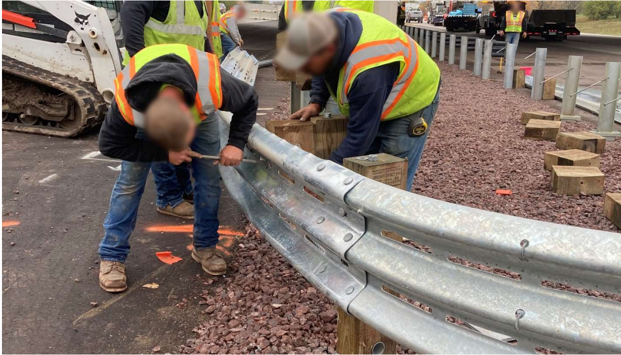
Figure 52 Attaching Blockouts and Installing Guardrail
