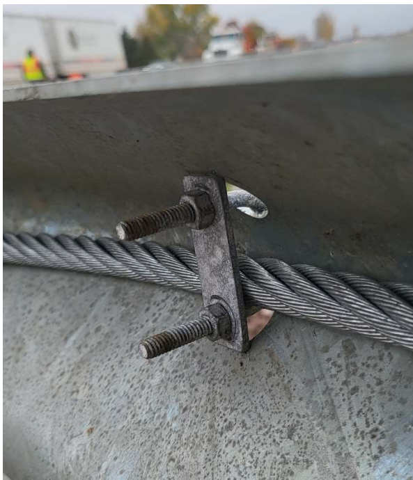
Figure 47 Nose Cable U-Bolt Orientation
