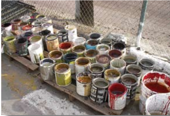
Hazardous materials—such as paint, fuel, oil, fertilizers, and such—should be managed to prevent spills or runoff into storm drains and waterways.
