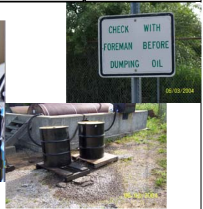
Bulk liquid storage drums are stored on pallets to protect the bottom from rust.
