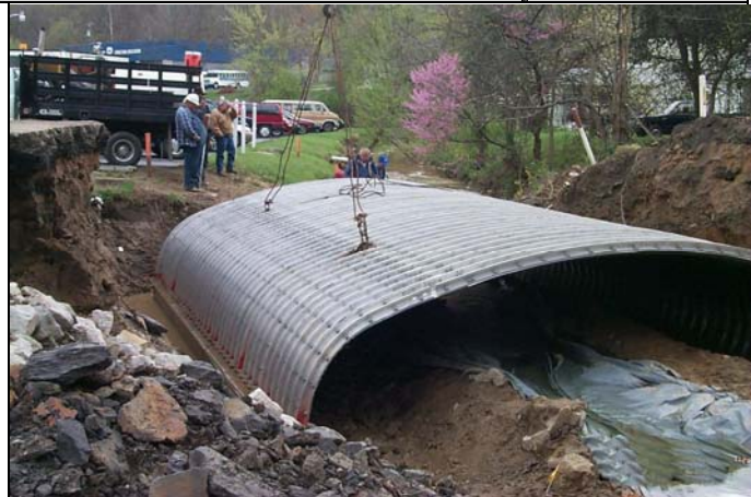
This bridge replacement includes stream isolation to minimize sediment discharge to the stream.
