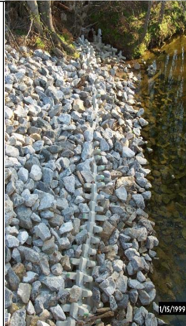
◀ A-Jacks were used to stabilize the foot of this embankment
