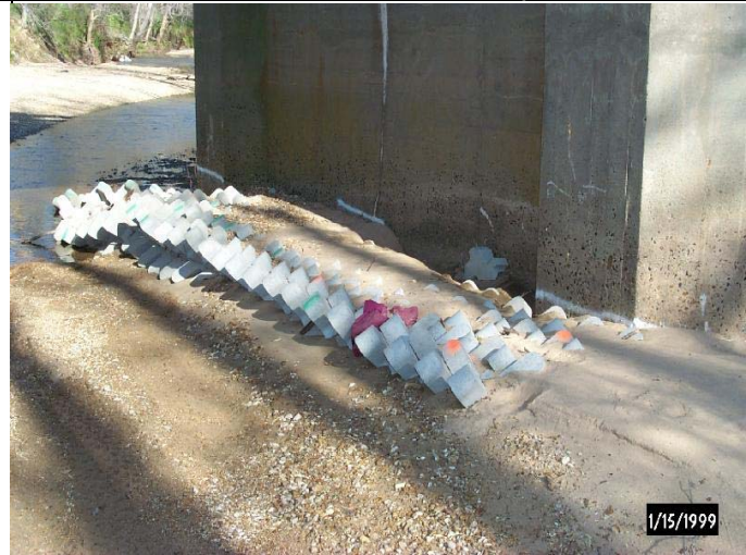
A-Jacks were used to encourage sediment deposits to fill in scour holes.
