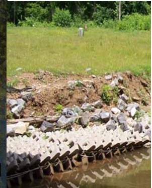
◀ A-Jacks were used to stabilize the foot of this embankment
