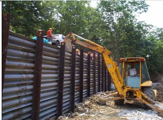
Railroad T- rails and cribs can be used to repair roadway slips adjacent to streams.
