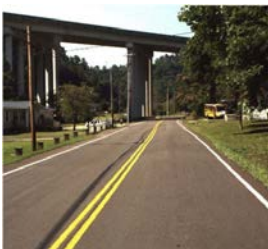
Typical MP Pavement
