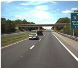
Typical Parkway Pavement
