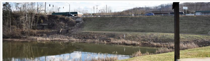
The west embankment separates the river from Panbowl Lake. Like the east embankment, there are different slope measurements on either side of the road. Fill material in the embankments includes topsoil, asphalt, rock, coarse grained alluvium, bedrock, shale/sandstone and groundwater.
