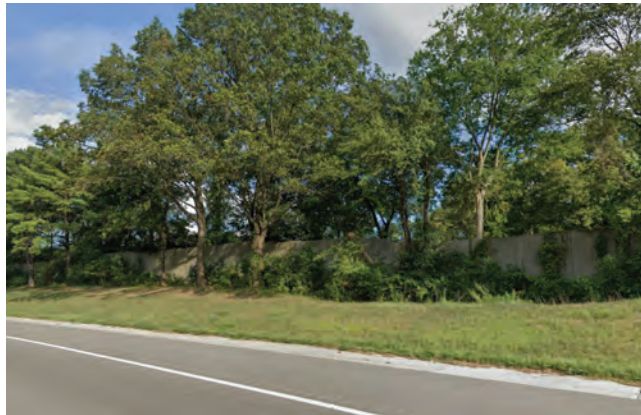
When warranted, barriers are a common method for reducing traffic noise along busy roadways.
