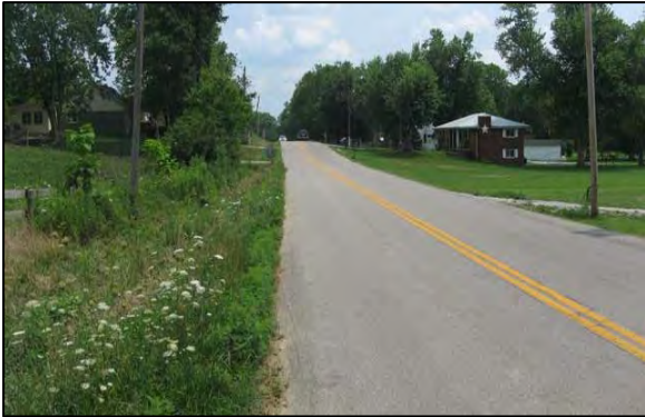
Two Lane Road Typical of Project Corridor Roads
