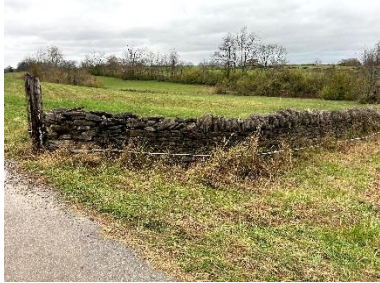
Roadside G north of entrance, view from road side.
