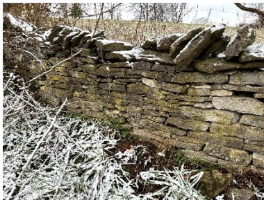
Roadside G south of entrance, section with covers and single copes.
