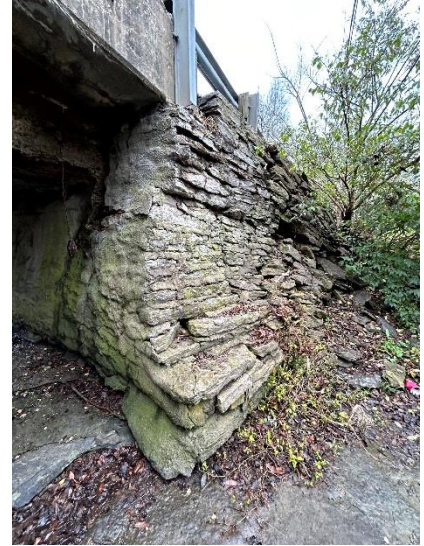
North roadside G, showing seamless transition into sw bridge wingwall
