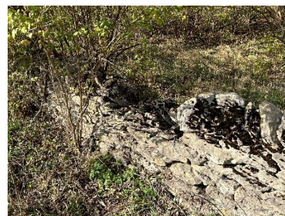
Resource D, detail showing single copes and rougher stone.
