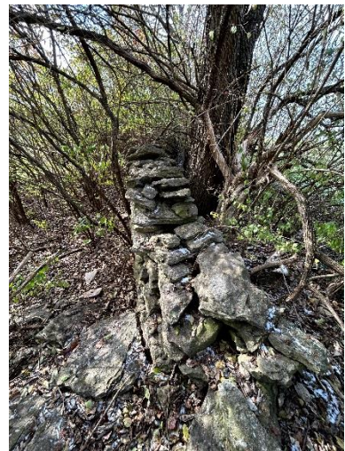
North F perpendicular fence, showing profile and batter.
