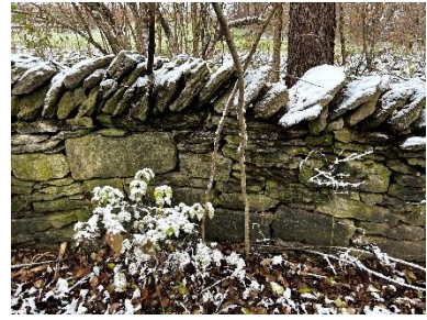
North F perpendicular fence, showing single copes and unusual thick stone near top of build.
