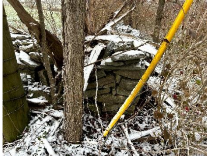
South roadside G, showing corner at junction with south perpendicular F.
