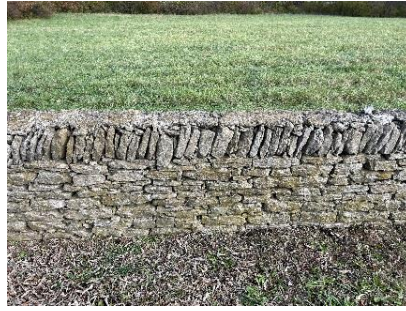
Groverland roadside fence, close up of repaired section with concrete cap, coursed stonework, and face chinking.
