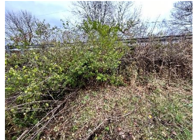
Roadside G north of entrance, view from field side at transition to bridge.
