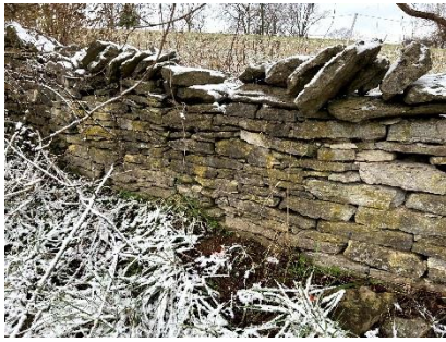
North roadside G, showing a section with covers and single copes.
