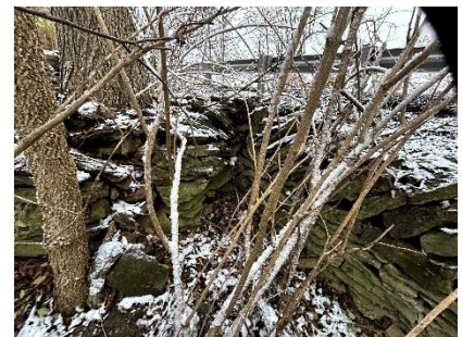
North roadside G, closeup showing integrated stonework, inside corner.
