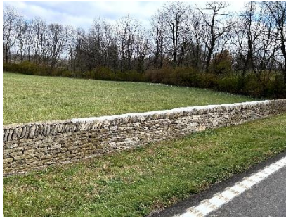
Groverland Farm Resource W roadside fence showing recent repair with concrete cap over double copes.
