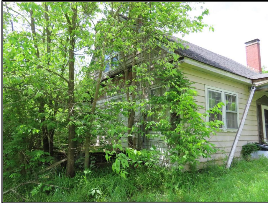
Figure 98. Site 8 (SC 174): Façade and south elevation of the residence (Resource B) looking northwest.
