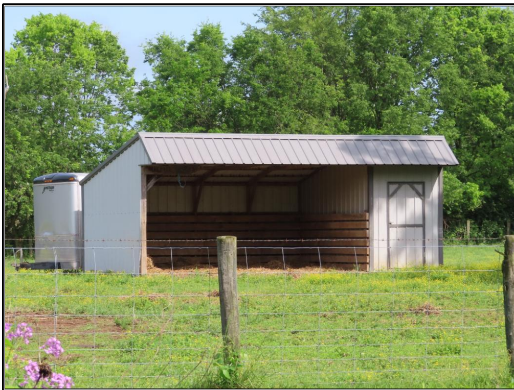
Figure 33. Site 2 (SC 813): Southeast and southwest elevations of the livestock shelter (Resource B), looking north.
