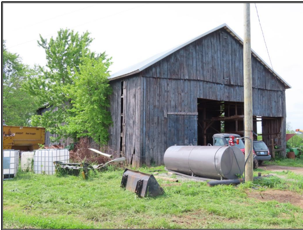
Figure 47. Site 3 (SC 173): East and south elevations of the barn (Resource E), looking northwest.
