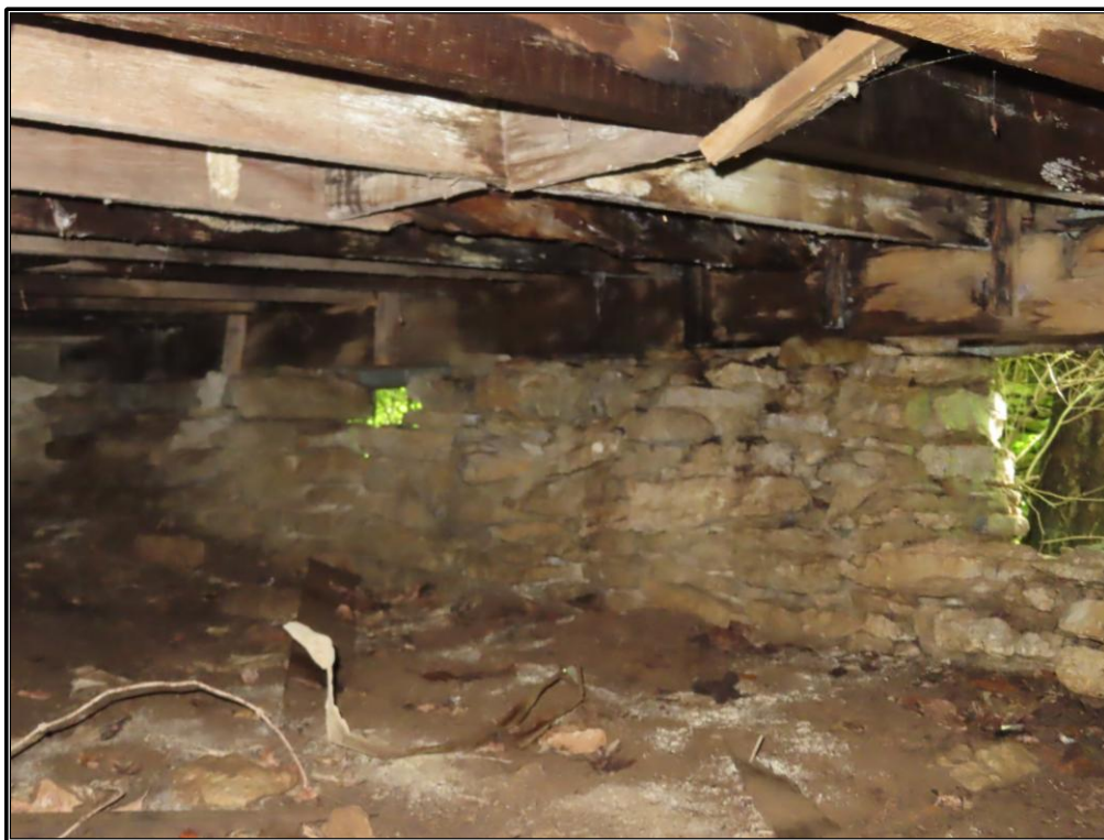
Figure 117. Site 8 (SC 174): Detail of the continuous stone foundation (Resource H).
