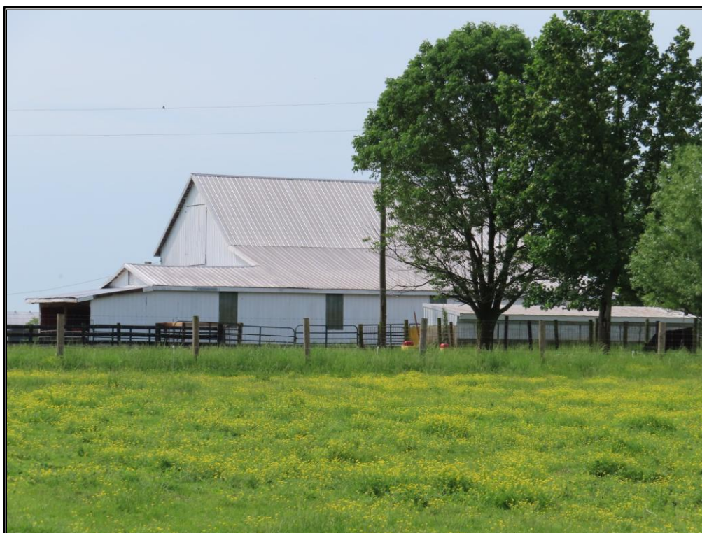
Figure 22. Site 1 (SC 808): Northwest and northeast elevations of the barn (Resource E) and shelter (Resource F), looking south.
