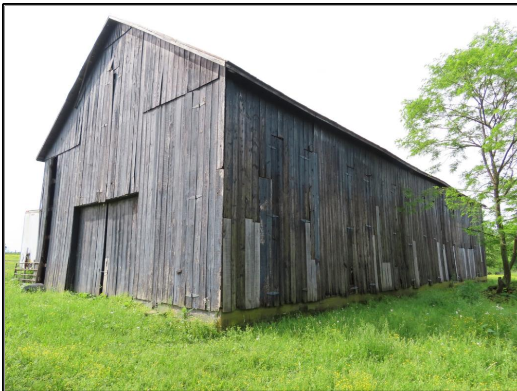
Figure 30. Site 2 (SC 813): Northwest and northeast elevations of the tobacco barn, looking south.
