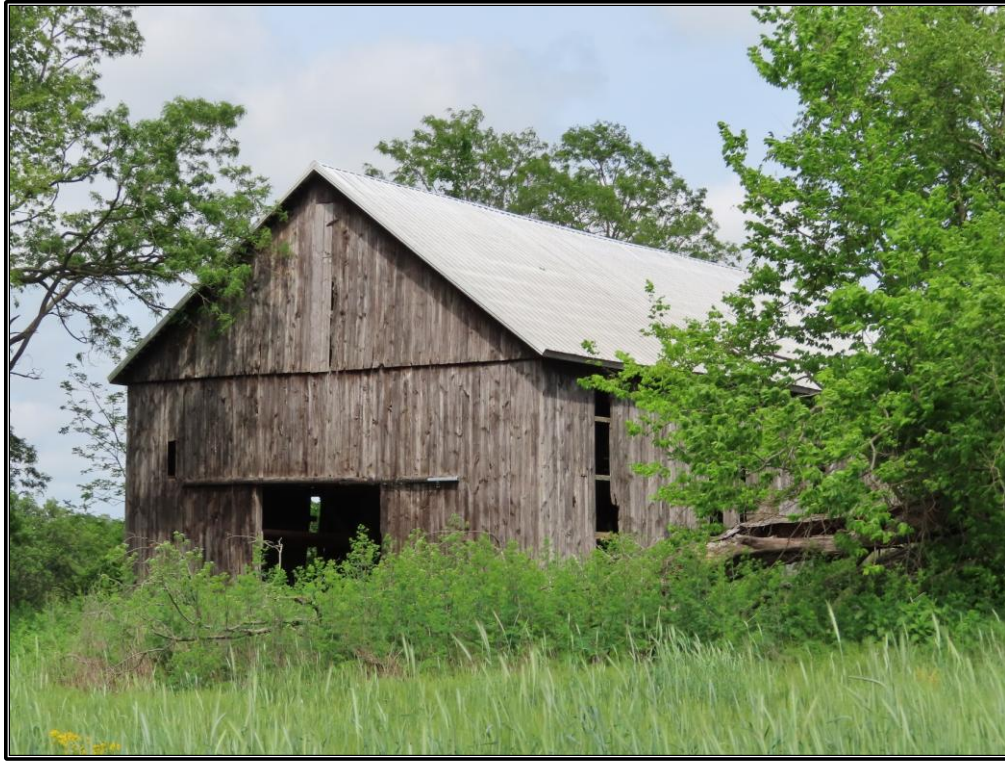
Figure 40. Site 3 (SC 173): West and south elevations of the barn (Resource C), looking northeast.
