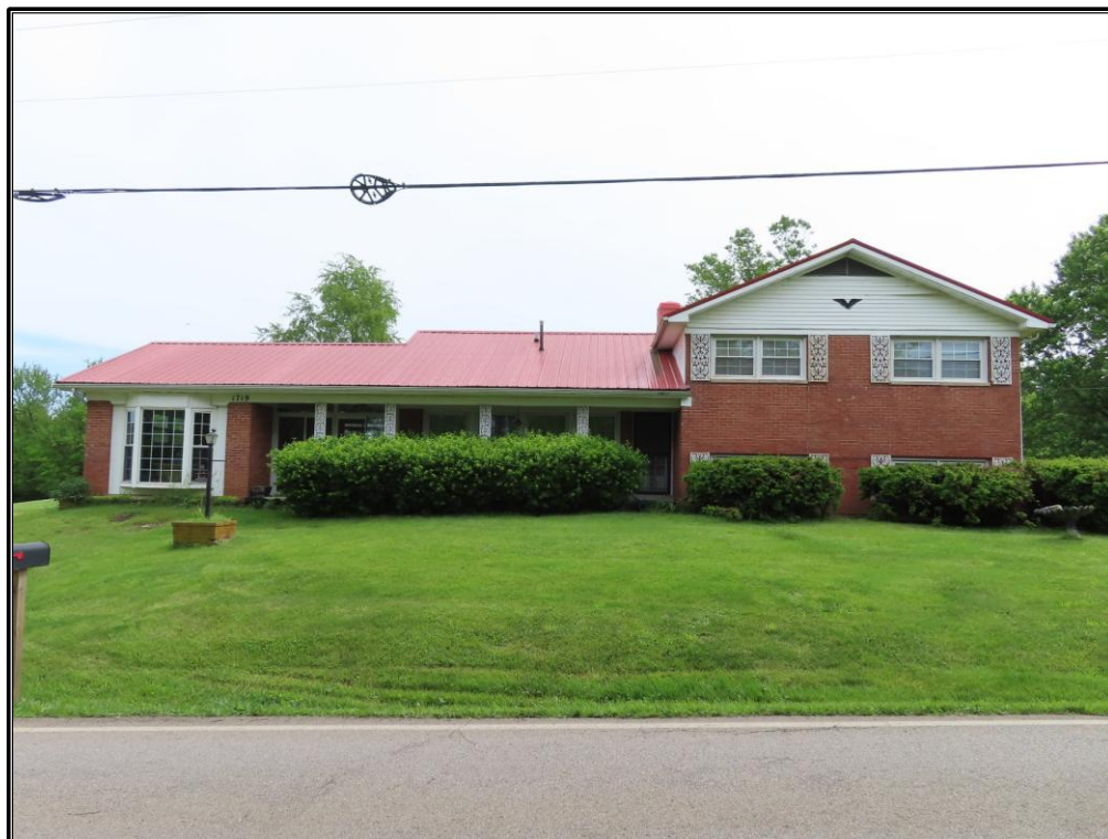
Figure 82. Site 7 (SC 813): Façade of the residence, looking northeast.
