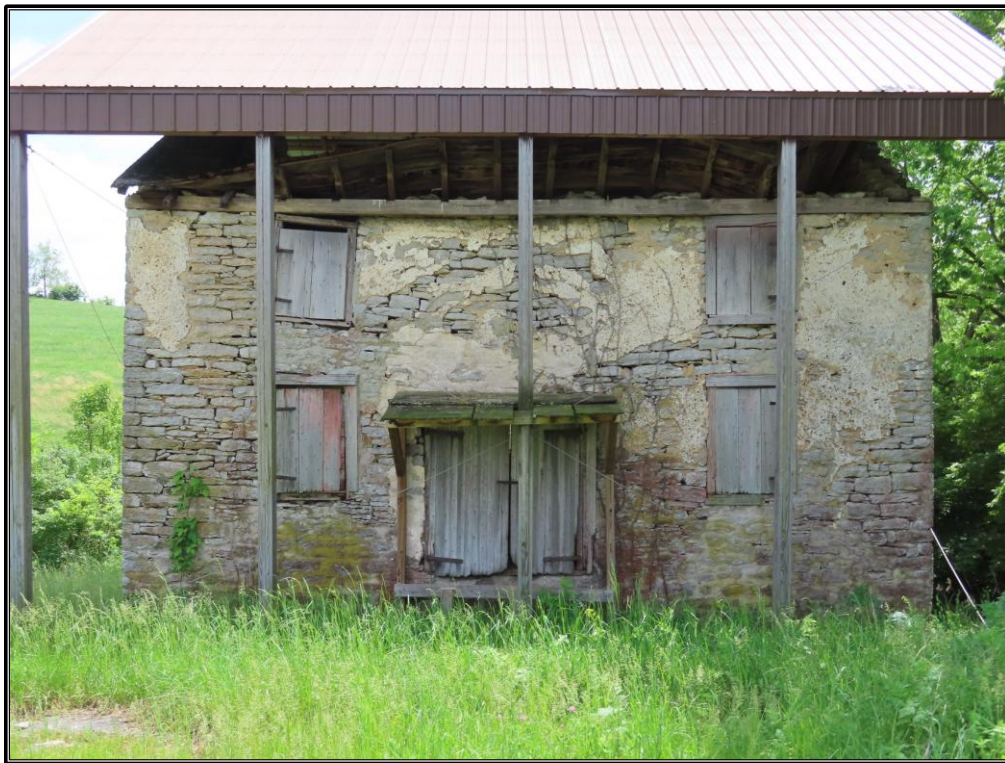
Figure 86. Site 8 (SC 174): Façade of the Choctaw Indian Academy, looking south.
