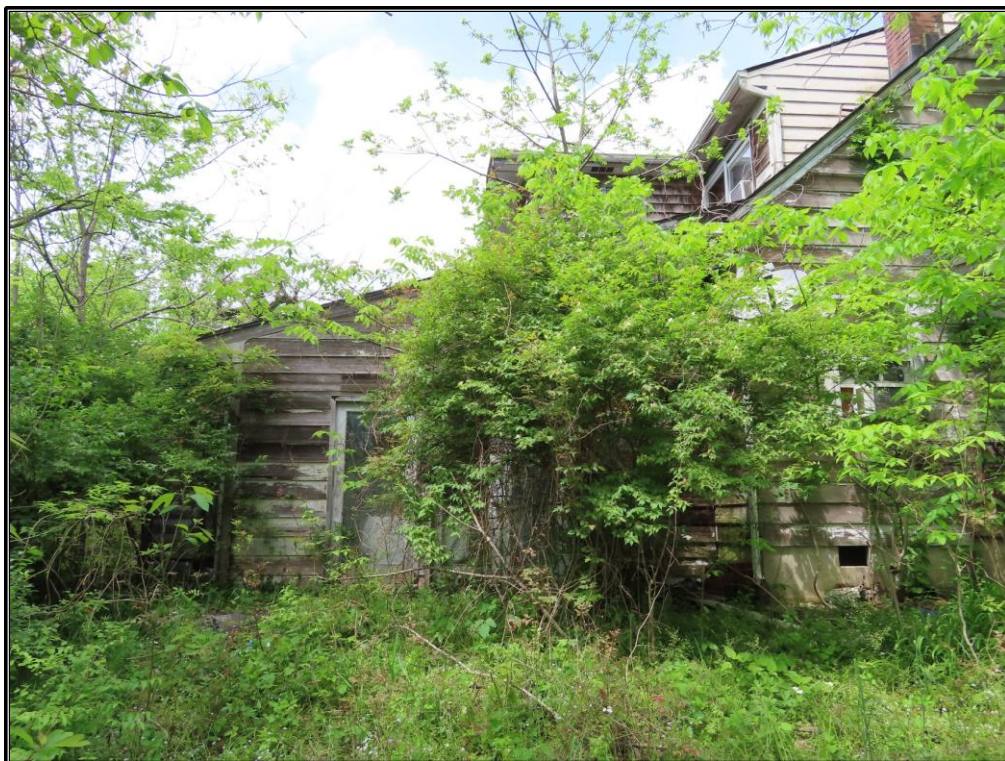
Figure 97. Site 8 (SC 174): South elevation of the residence (Resource B), looking north.
