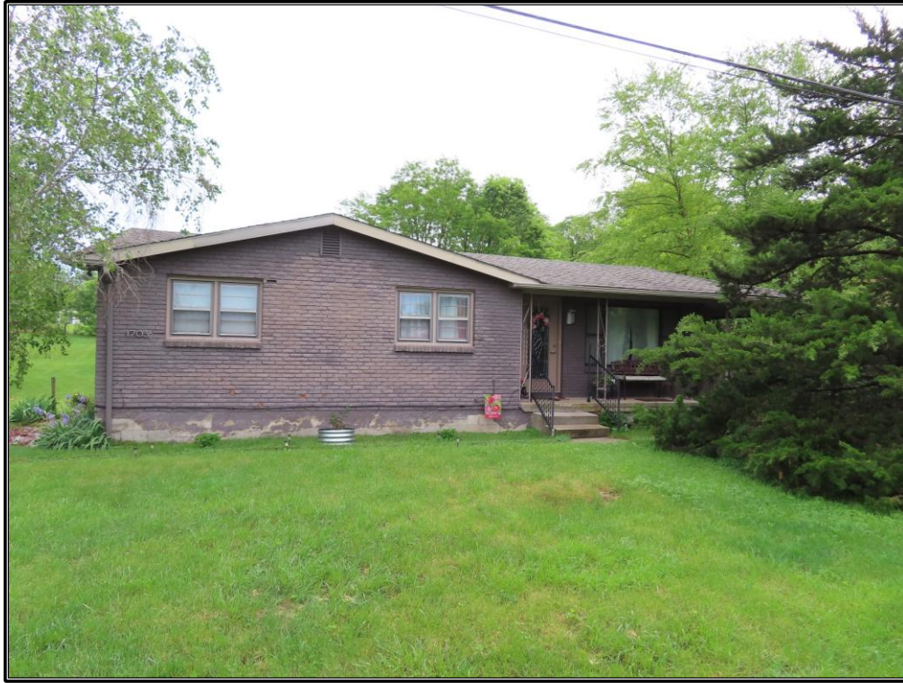
Figure 81. Site 6 (SC 812): Façade of the residence, looking northeast.
