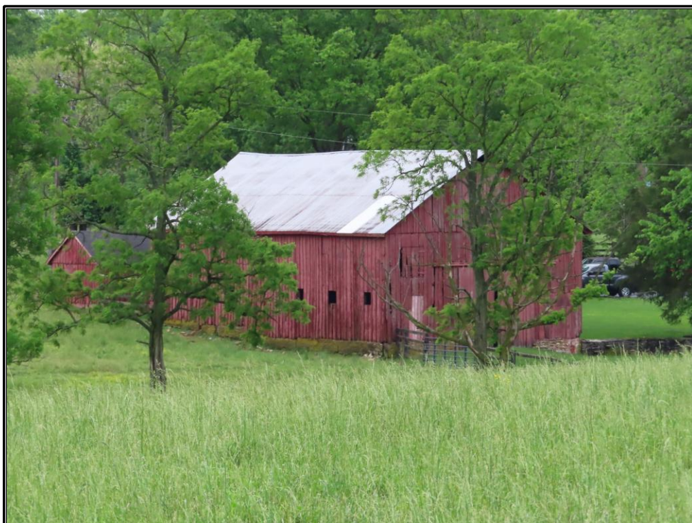
Figure 135. Site 10 (SC 150): Northwest and southwest elevations of the barn (Resource H), looking east-southeast.
