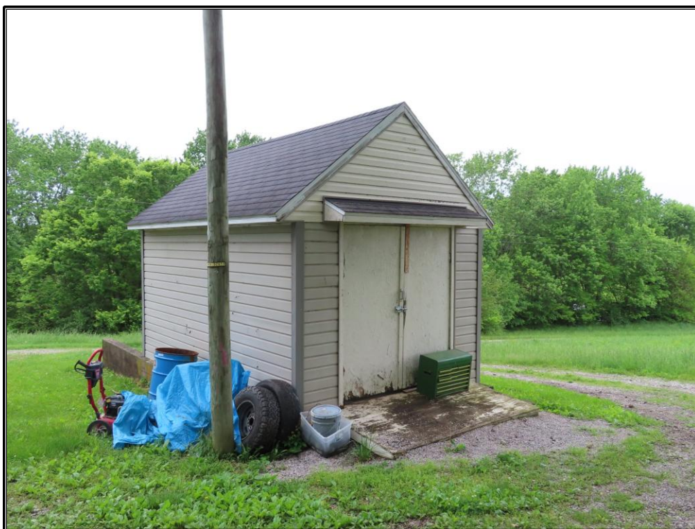
Figure 159. Site 10 (SC 150): East and south elevations of the shed (Resource Z), looking northwest.
