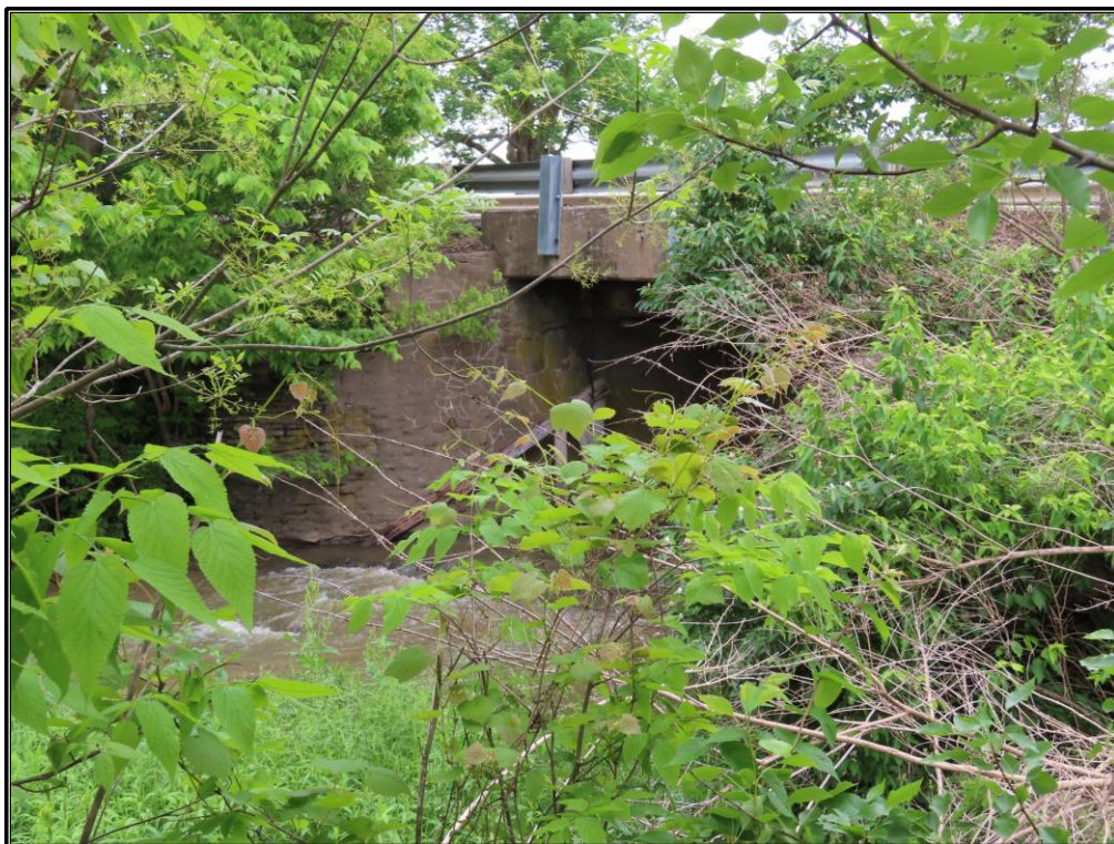
Figure 171. Site 11 (SC 817): View of the substructure and abutments, looking northeast.
