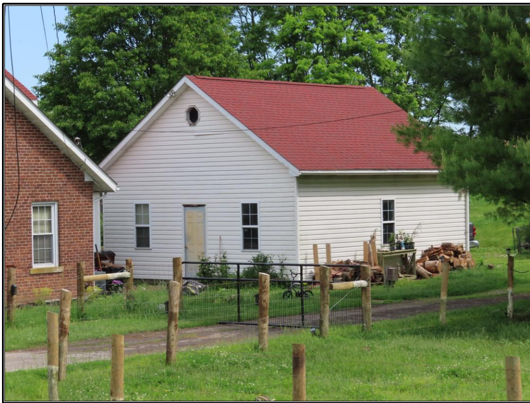
Figure 77. Site 5 (SC 811): Southeast and southwest elevations of the garage (Resource A), looking north.
