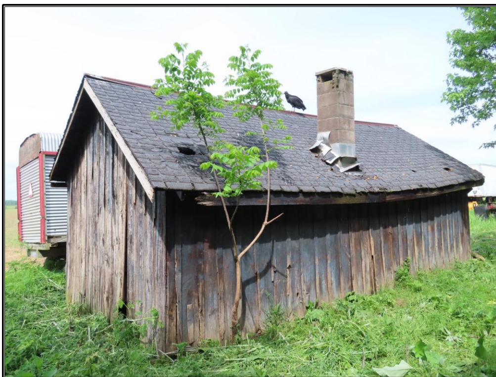
Figure 52. Site 3 (SC 173): West and south elevations of the shed (Resource F), looking northeast.
