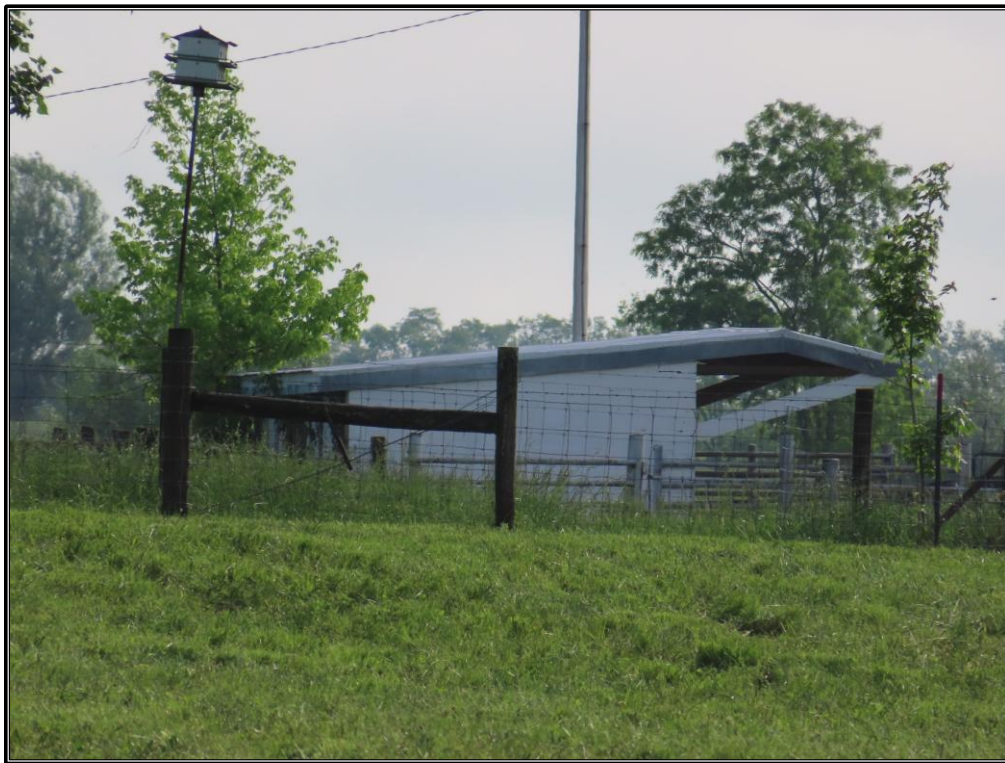
Figure 27. Site 1 (SC 808): Southwest elevation of the shelter (Resource J), looking northeast.
