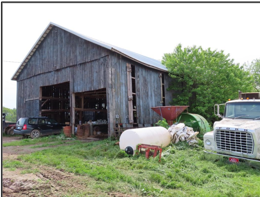
Figure 48. Site 3 (SC 173): East and north elevations of the barn (Resource E), looking southwest.
