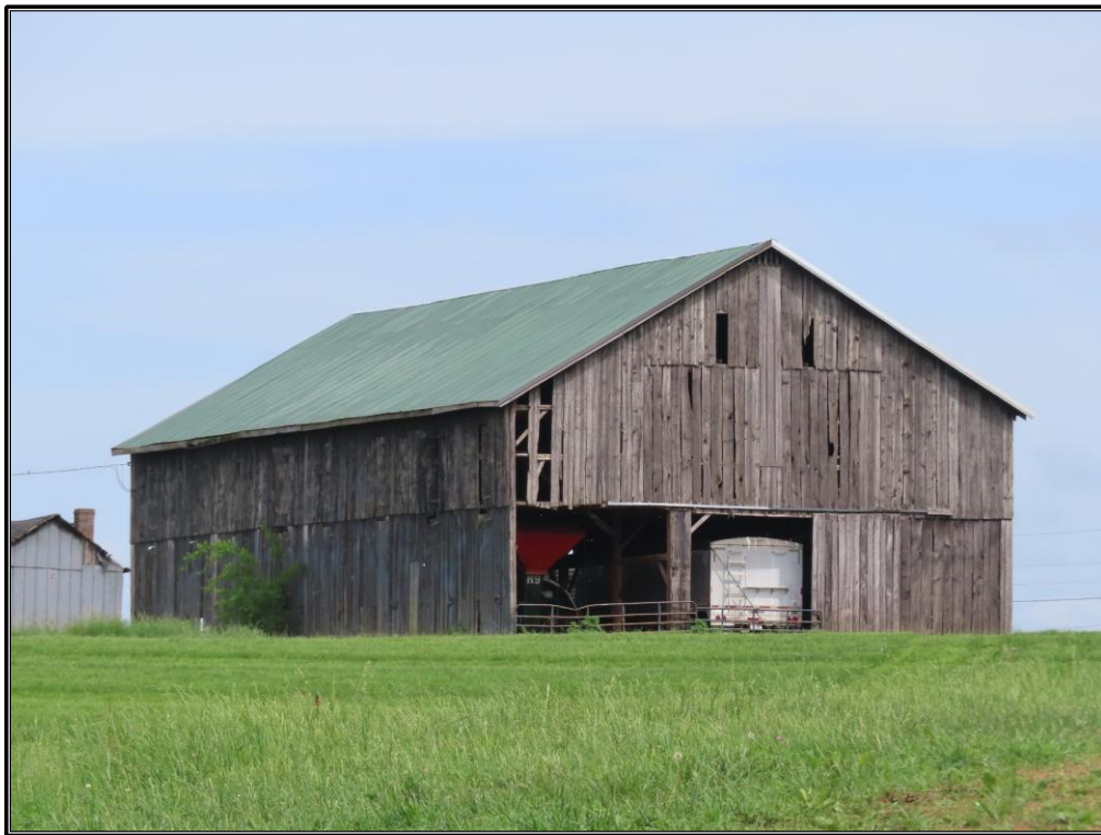
Figure 60. Site 3 (SC 173): North and west elevations of the barn (Resource M), looking southeast.
