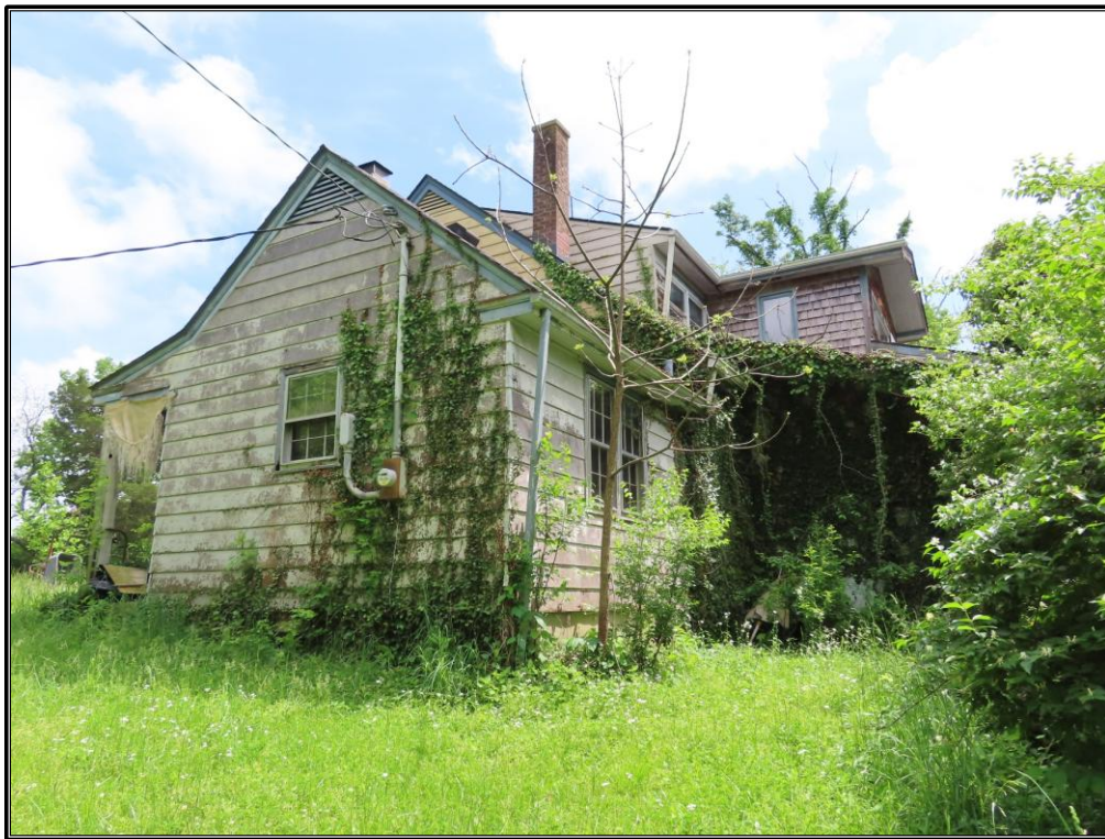
Figure 96. Site 8 (SC 174): North and west (rear) elevations of the residence (Resource B), looking east.
