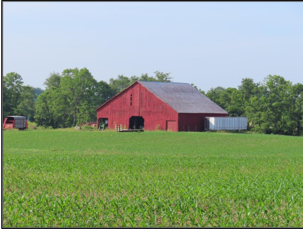
Figure 144. Site 10 (SC 150): Northeast and northwest elevations of the barn (Resource N), looking south-southeast.
