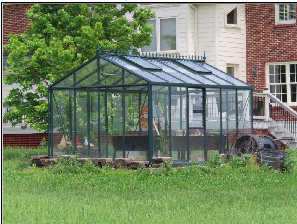
Figure 131. Site 9 (SC 814): Southeast and southwest elevations of the greenhouse (Resource C), looking north-northeast.
