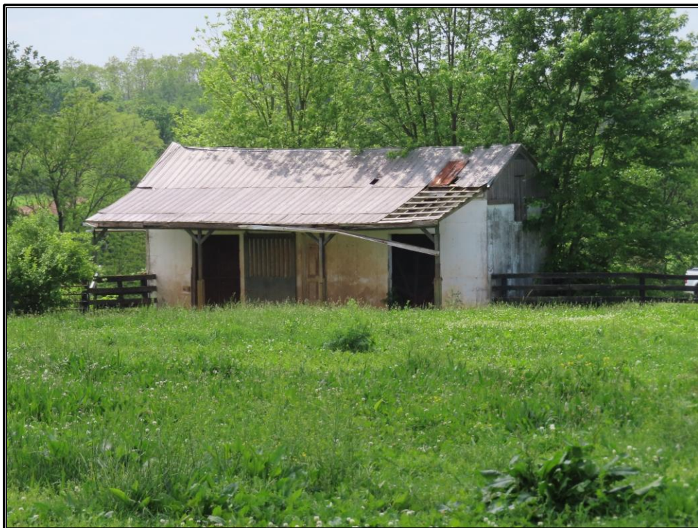
Figure 132. Site 9(SC 814): North and east elevations of the stable (Resource D), looking southwest.
