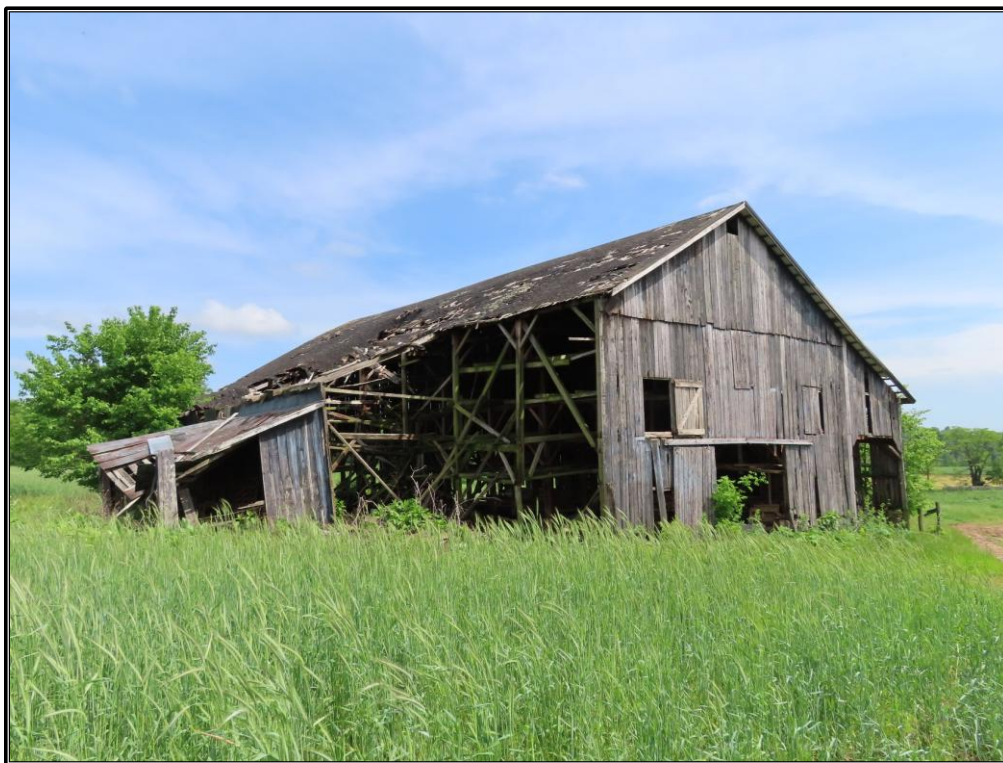
Figure 43. Site 3 (SC 173): East and south elevations of the barn (Resource D), looking west-northwest.
