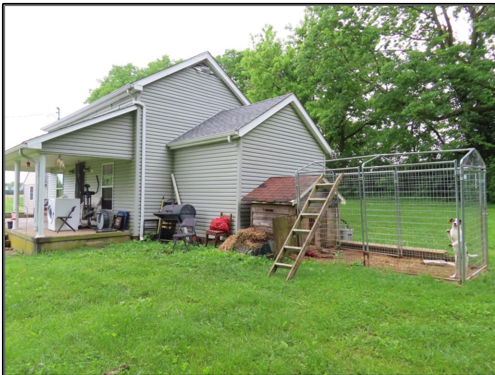
Figure 157. Site 10 (SC 150): Façade and south elevation of the residence (Resource Y), looking northeast.
