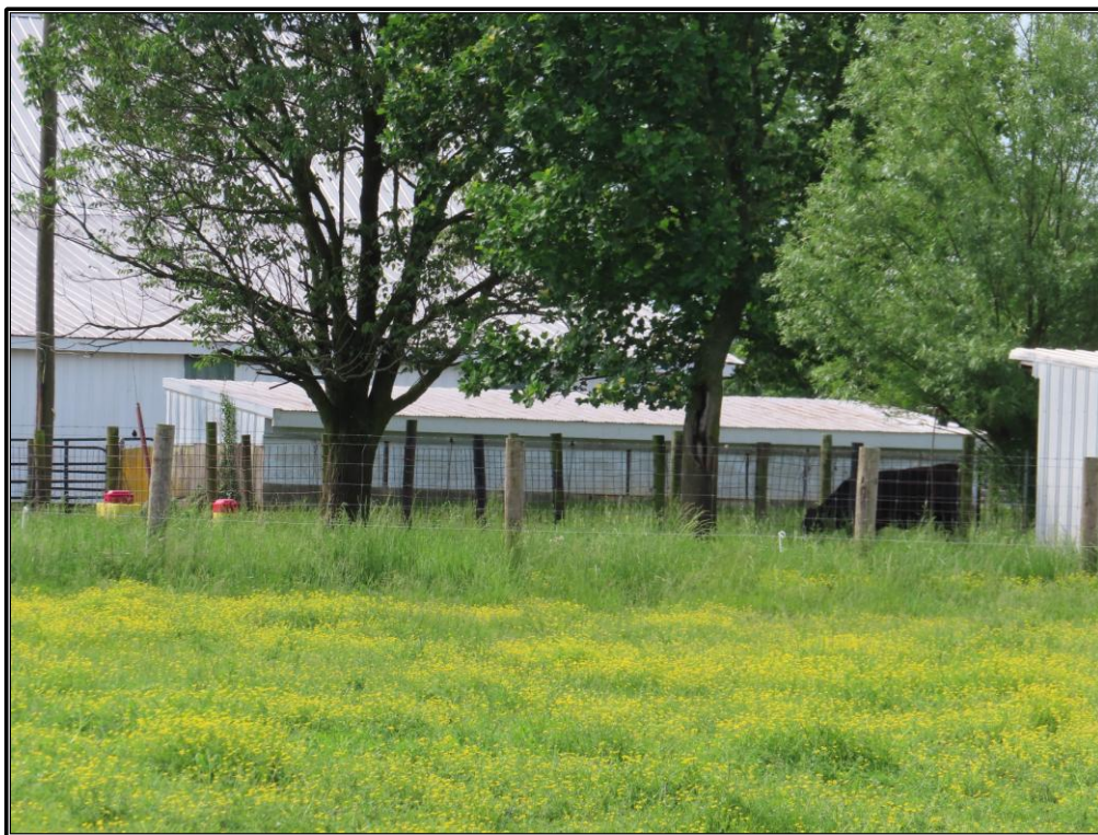
Figure 23. Site 1 (SC 808): Northwest and northeast elevations of the shelter (Resource F), looking south.
