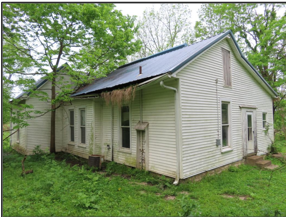
Figure 64. Site 3 (SC 173): West and south (rear) elevations of the residence (Resource O), looking northeast.
