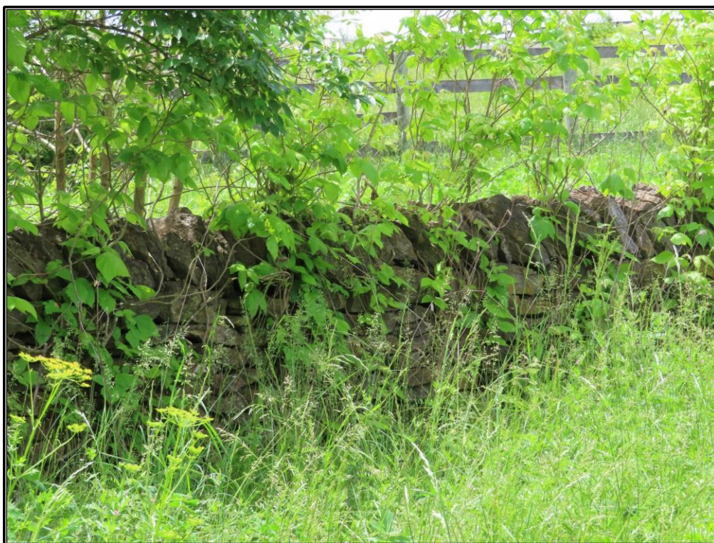
Figure 127. Site 9 (SC 814): Detail of the fence.
