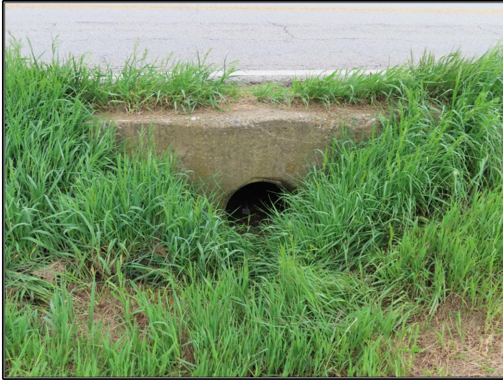
Figure 177. Site B (SC 816): Northeast elevation of Site B, looking southwest.
