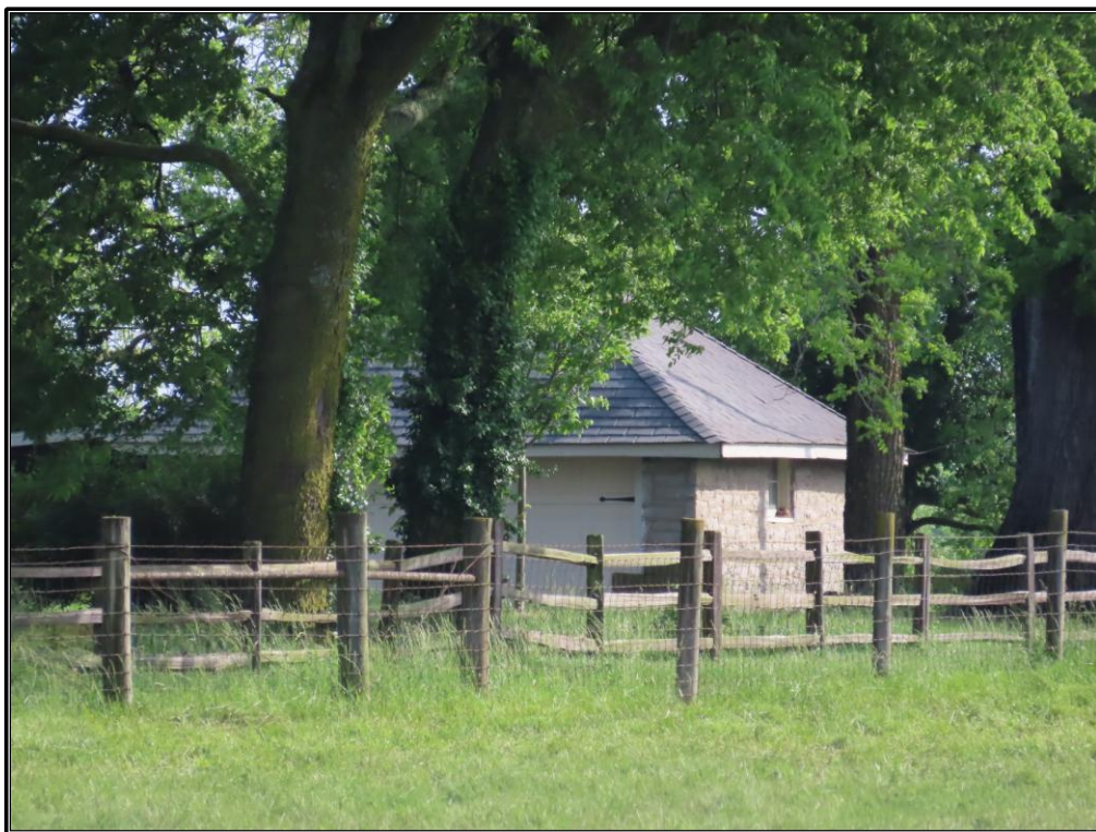
Figure 17. Site 1 (SC 808): Southwest and southeast elevations of the garage (Resource A), looking north.
