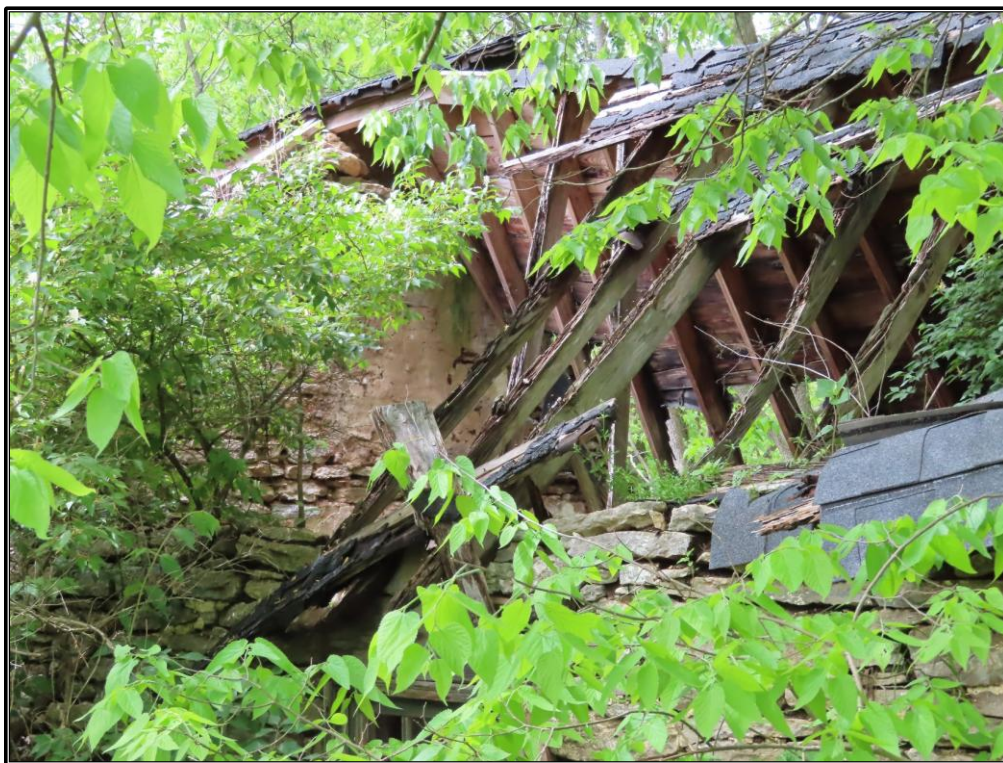
Figure 92. Site 8 (SC 174): Detail of the roof (Resource A), looking northeast.
