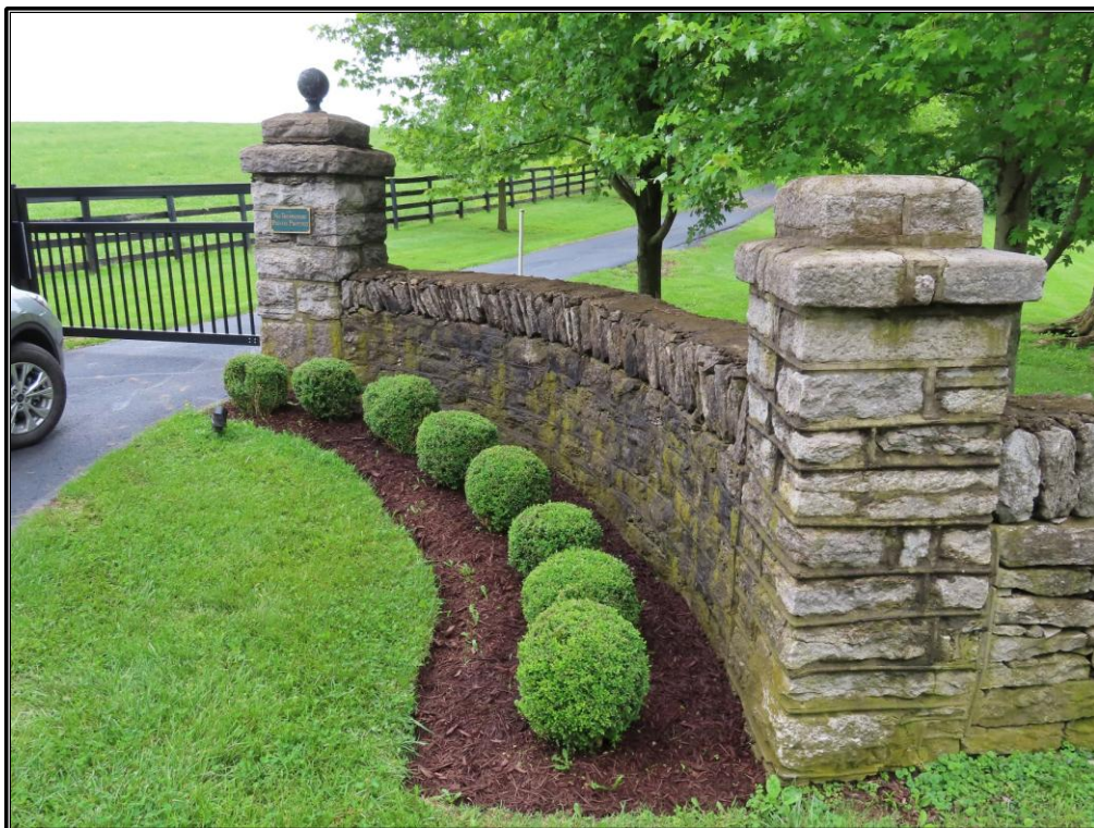
Figure 154. Site 10 (SC 150): View of the entry (Resource W), looking east-northeast.
