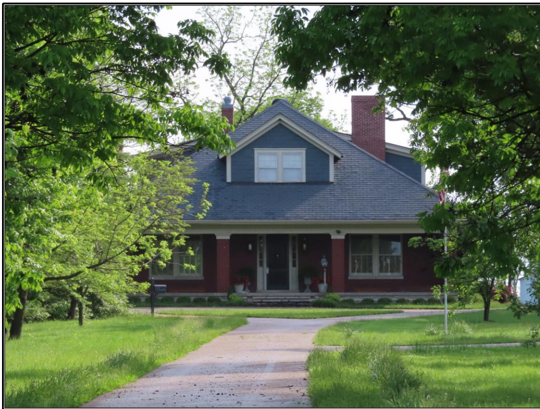
Figure 14. Site 1 (SC 808): Façade of the residence, looking northeast.
