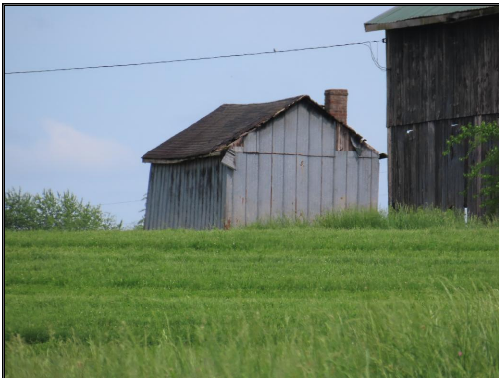
Figure 61. Site 3 (SC 173): North and west elevations of the shed (Resource N), looking southeast.
