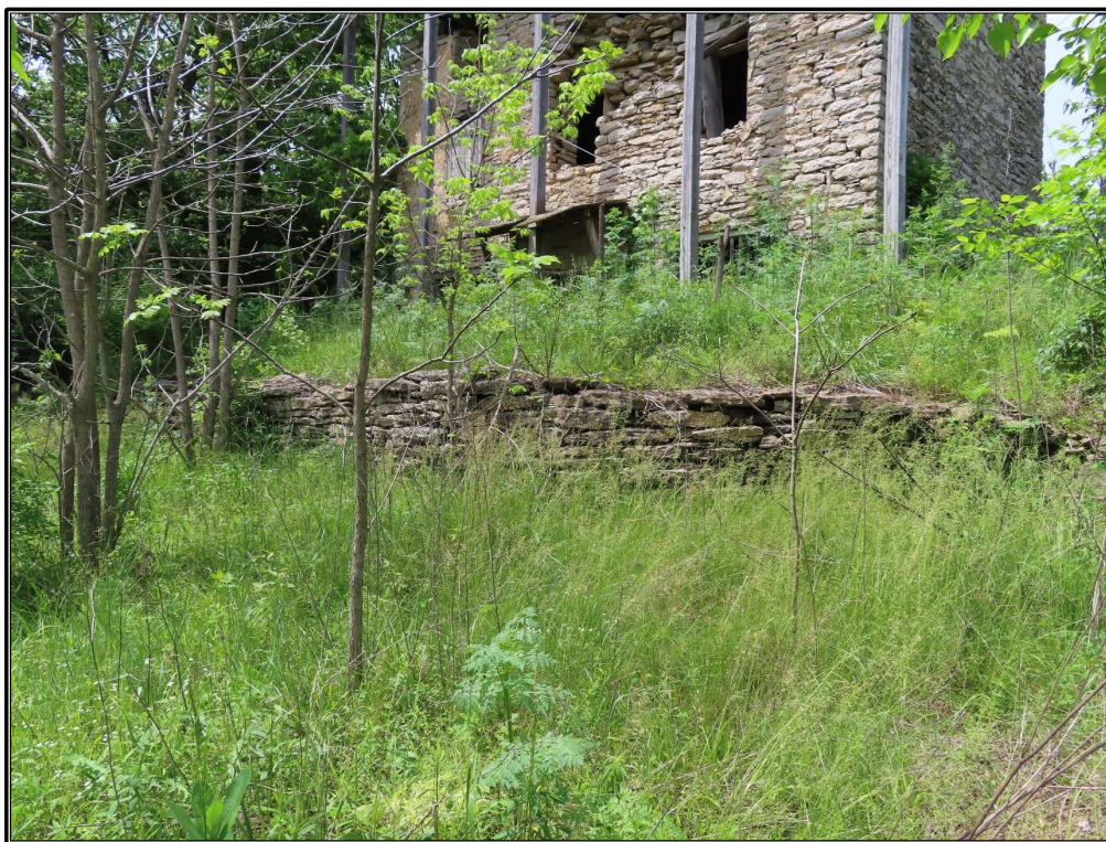
Figure 99. Site 8 (SC 174): View of the retaining wall (Resource C), looking northwest.
