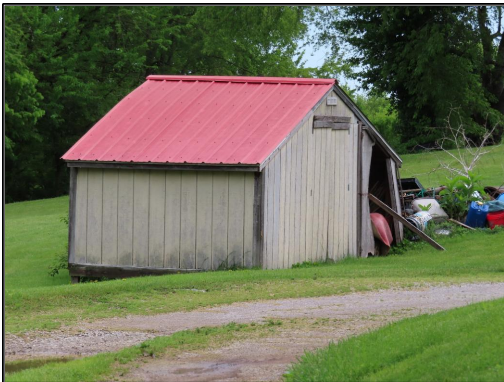
Figure 85. Site 7 (SC 813): Southwest and southeast elevations of the shed (Resource A), looking north-northeast.
