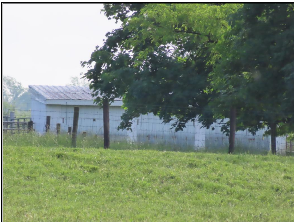
Figure 28. Site 1 (SC 808): Southwest and southeast elevations of the shelter (Resource K), looking northeast.
