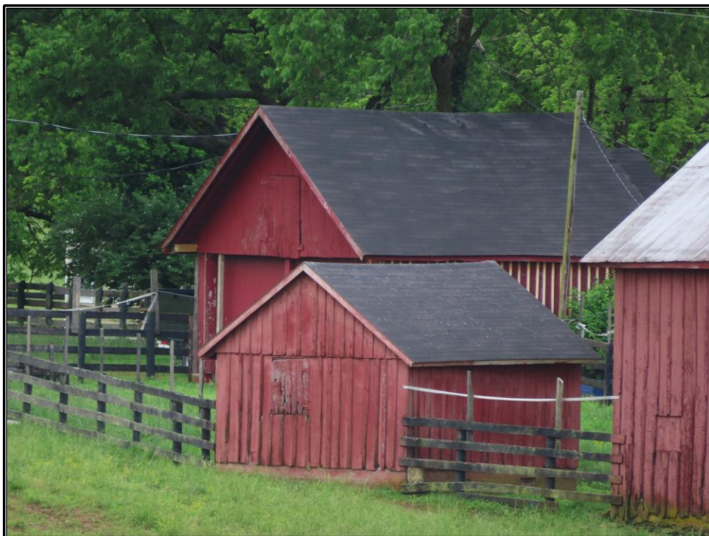
Figure 134. Site 10 (SC 150): Northwest and southwest elevations of the garage (Resource E) and the shed (Resource G), looking east-southeast.
