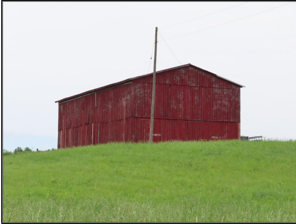
Figure 155. Site 10 (SC 150): South and west elevations of the barn (Resource X), looking northeast.
