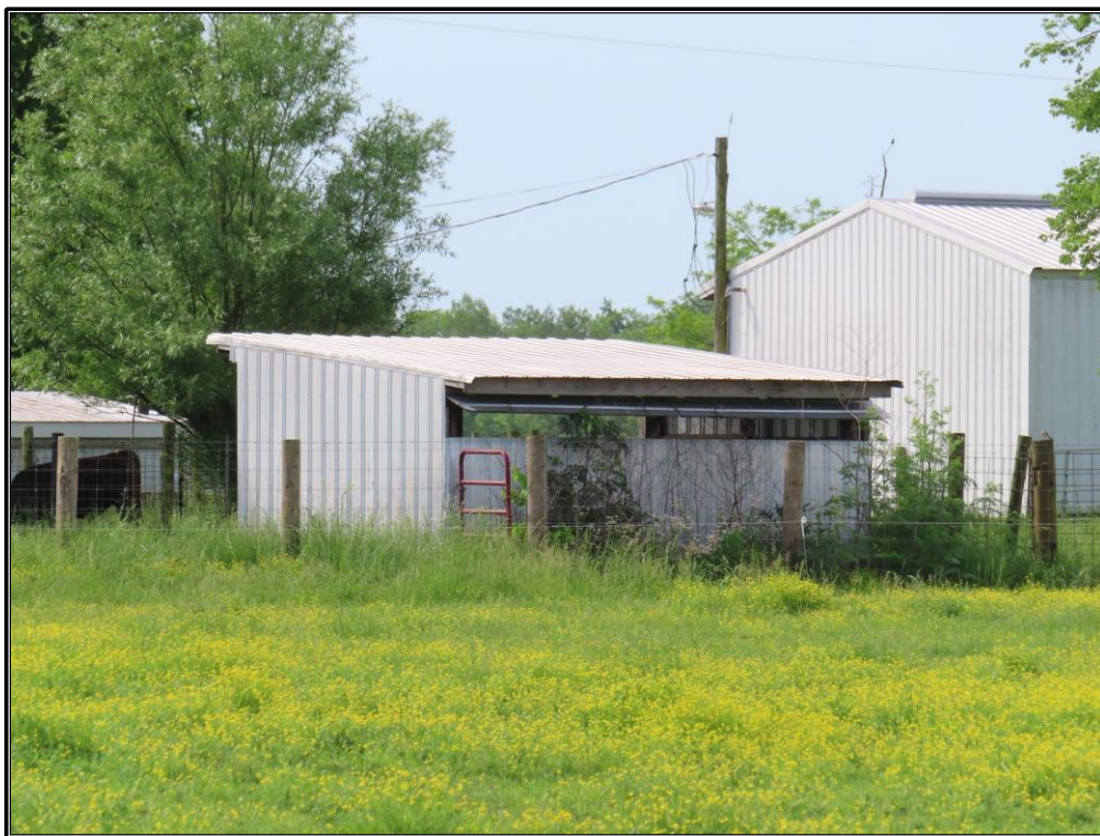
Figure 25. Site 1 (SC 808): Northwest and northeast elevations of the shelter (Resource H), looking south-southeast.
