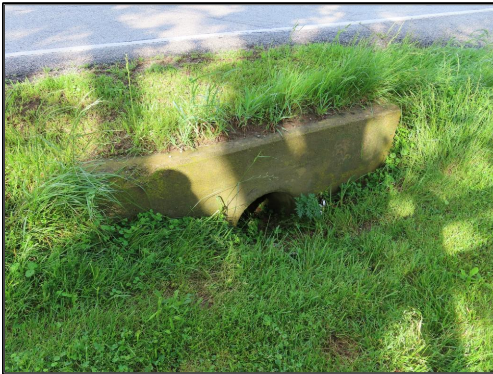
Figure 175. Site A (SC 815): Northeast elevation of Site A, looking south.
