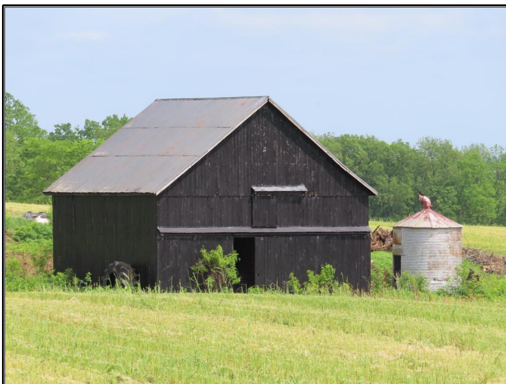
Figure 37. Site 3 (SC 173): West and north elevations of the barn (Resource A) and view of the grain bin (Resource B), looking southeast.
