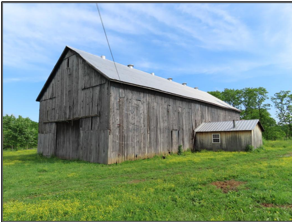
Figure 29. Site 2 (SC 813): Southeast and southwest elevations of the tobacco barn, looking north.
