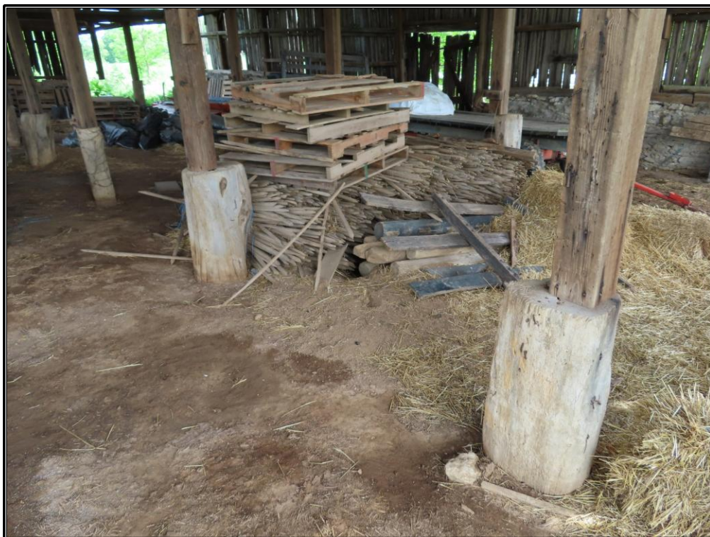
Figure 46. Site 3 (SC 173): Interior view of the barn (Resource D).
