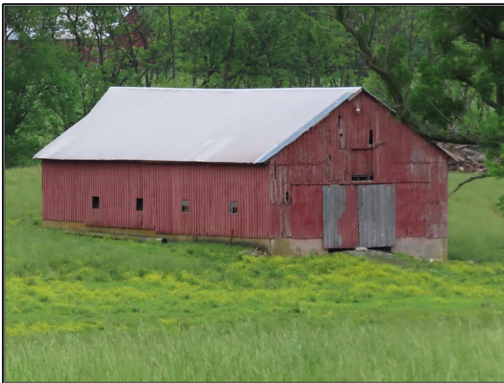
Figure 136. Site 10 (SC 150): Northwest and southwest elevations of the barn (Resource I), looking east-southeast.
