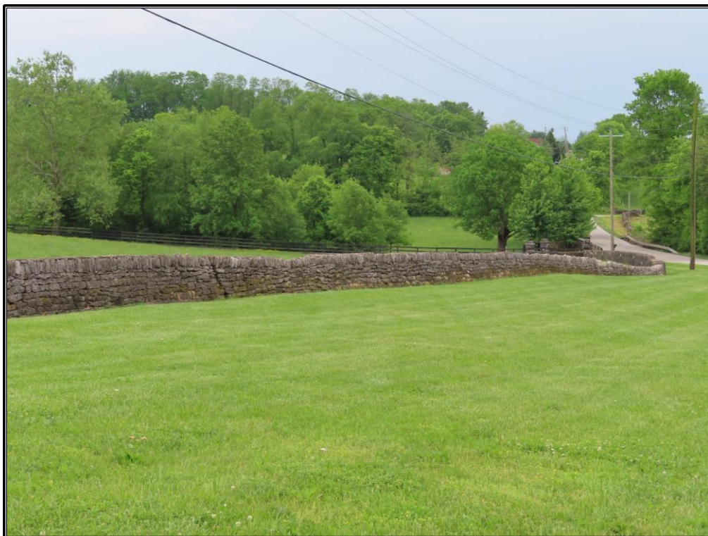
Figure 152. Site 10 (SC 150): View of the stone fence (Resource W), looking southeast.
