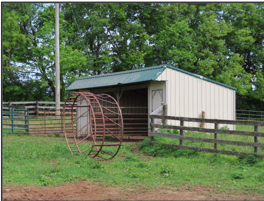
Figure 55. Site 3 (SC 173): North and west elevations of the livestock shelter (Resource I), looking southeast.
