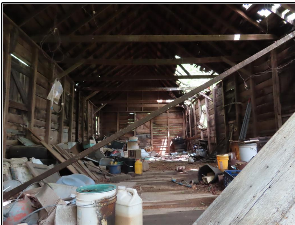
Figure 118. Site 8 (SC 174): Interior view of the north, east, and south elevations (Resource H), looking west.
