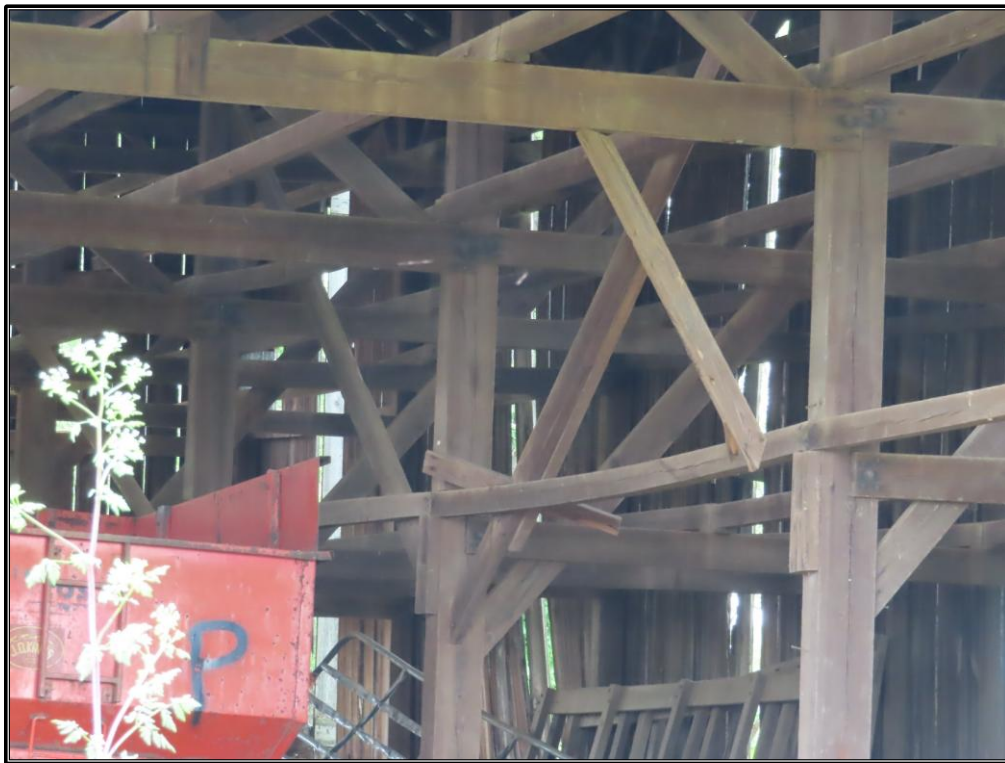
Figure 41. Site 3 (SC 173): Interior of the barn (Resource C).
