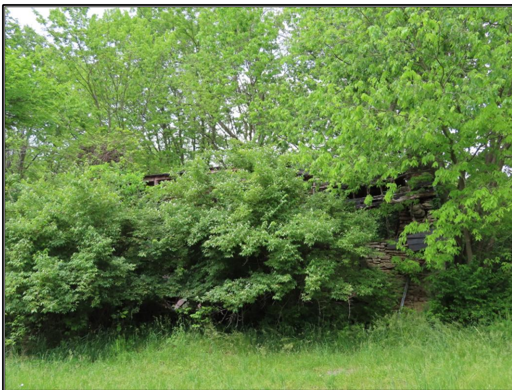
Figure 91. Site 8 (SC 174): Obscured view of the façade of the stone building (Resource A), looking north.
