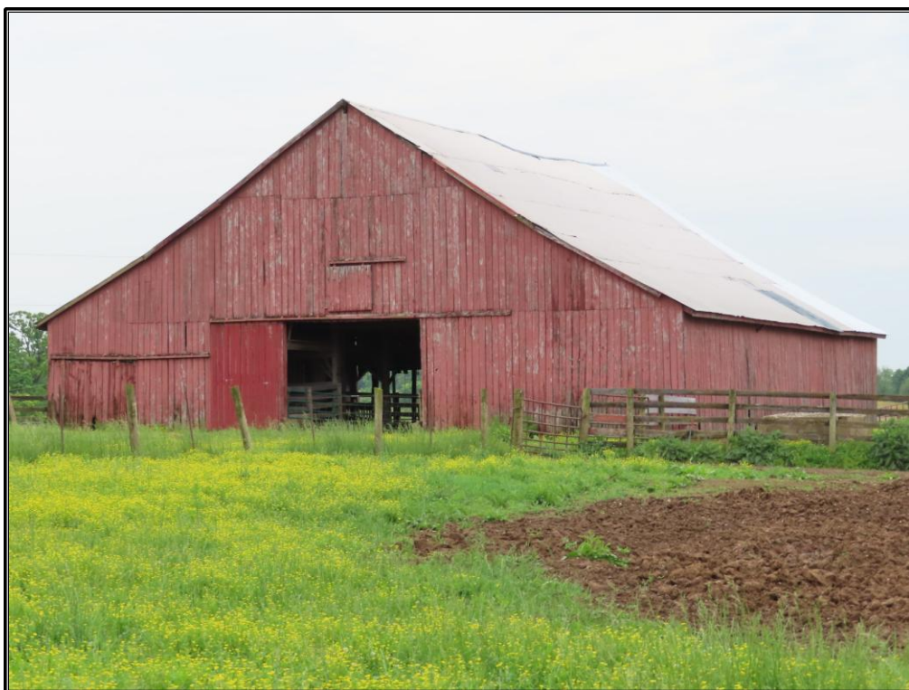
Figure 143. Site 10 (SC 150): Northwest and southwest elevations of the barn (Resource M), looking east.
