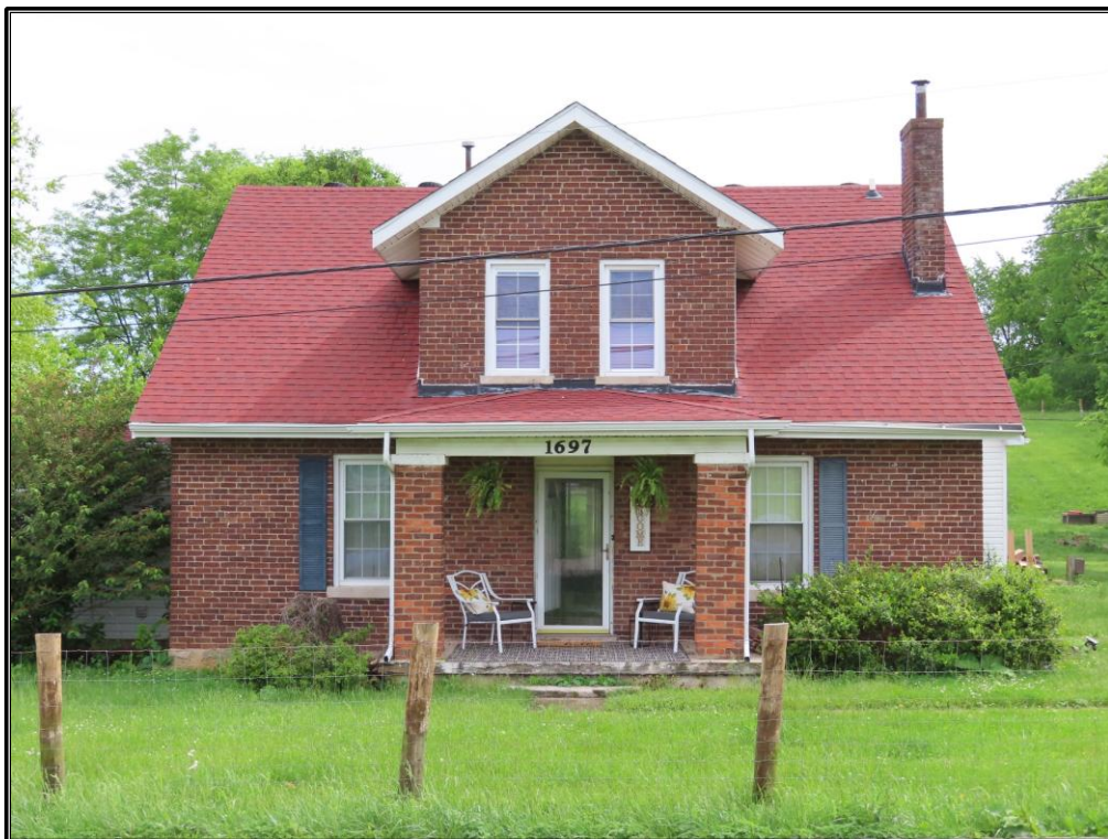
Figure 75. Site 5 (SC 811): Façade of the residence, looking northeast.
