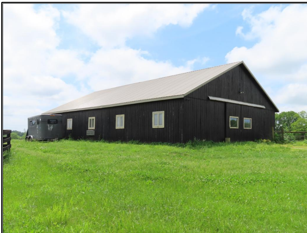
Figure 130. Site 9 (SC 814): North and east elevations of the barn (Resource B), looking southwest.
