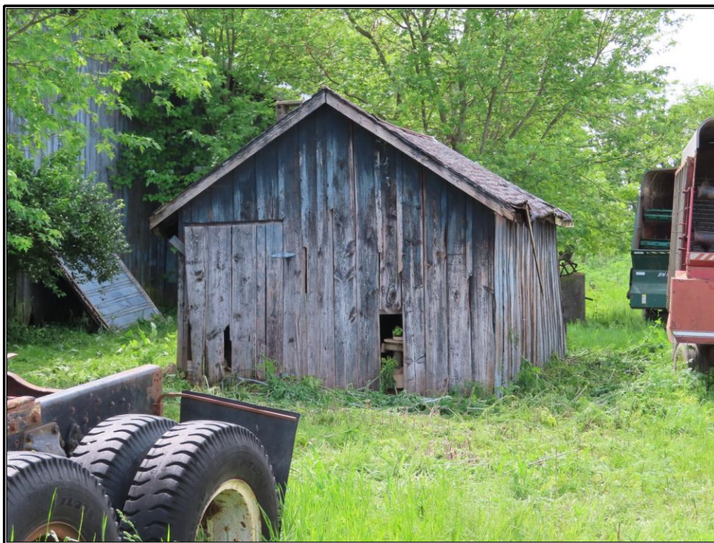
Figure 51. Site 3 (SC 173): East and north elevations of the shed (Resource F), looking west-southwest.
