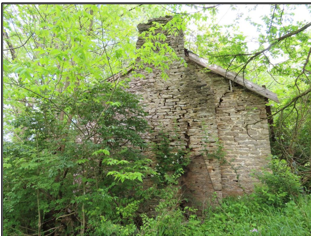
Figure 93. Site 8 (SC 174): West elevation of the stone building (Resource A), looking east.
