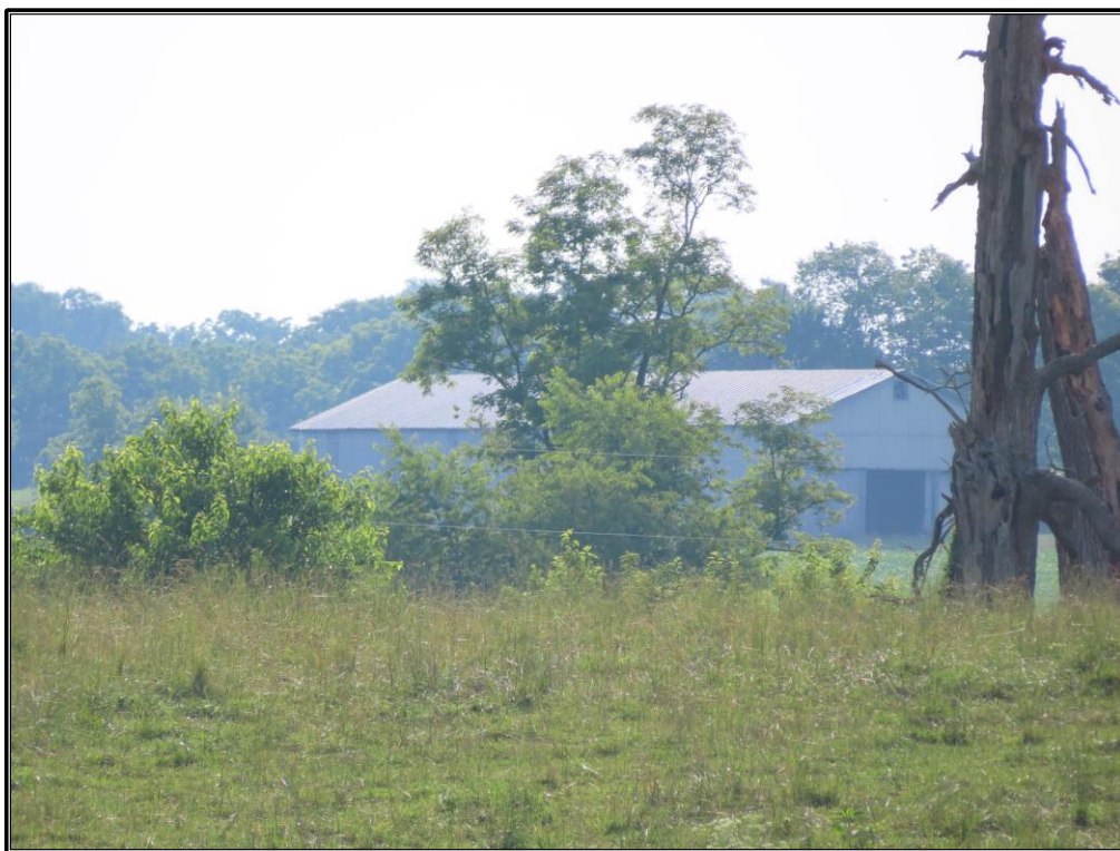
Figure 148. Site 10 (SC 150): Northeast and northwest elevations of the barn (Resource U), looking southeast.
