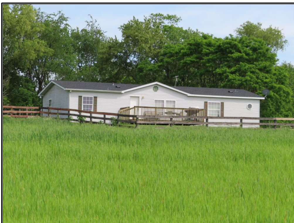
Figure 54. Site 3 (SC 173): Façade and north elevation of the manufactured home (Resource H), looking south-southeast.
