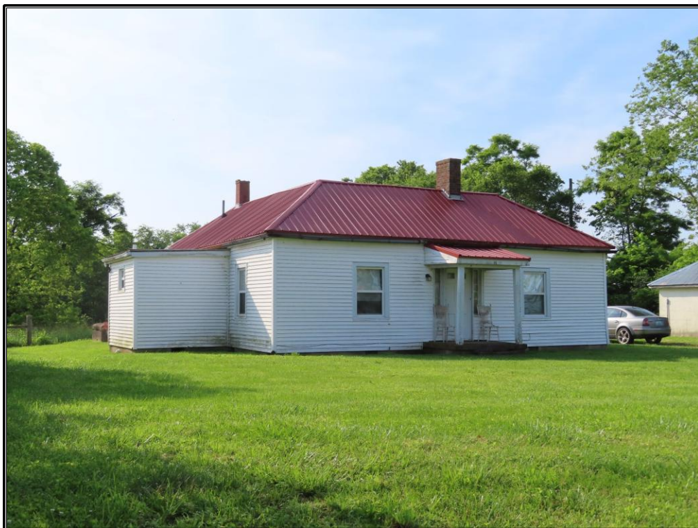
Figure 163. Site 10 (SC 693): Façade and north elevation of the residence (Resource AA), looking southeast.
