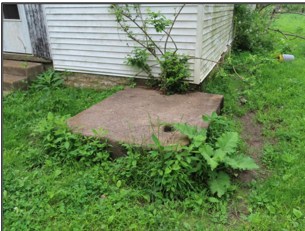
Figure 65. Site 3 (SC 173): View of the cistern (Resource P).
