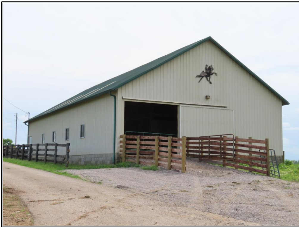
Figure 58. Site 3 (SC 173): North and east elevations of the barn (Resource L), looking southwest.
