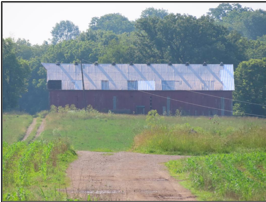
Figure 145. Site 10 (SC 150): Northwest elevation of the barn (Resource O), looking south-southeast.
