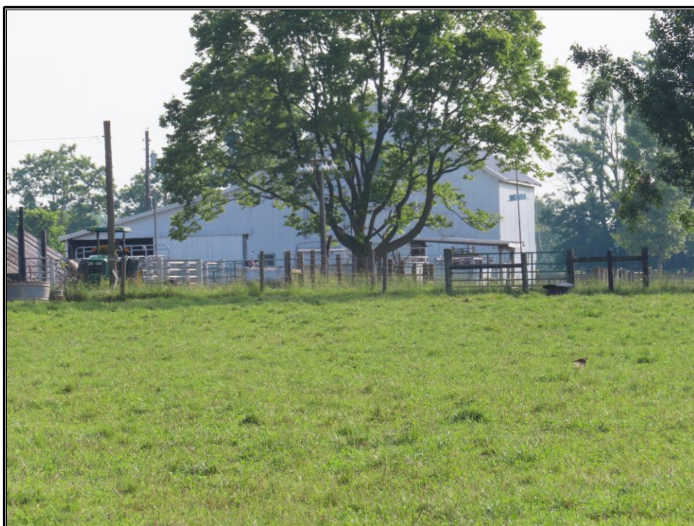
Figure 20. Site 1 (SC 808): View of the shelter (Resource C) and southeast and southwest elevations of the shelter (Resource F), looking north.
