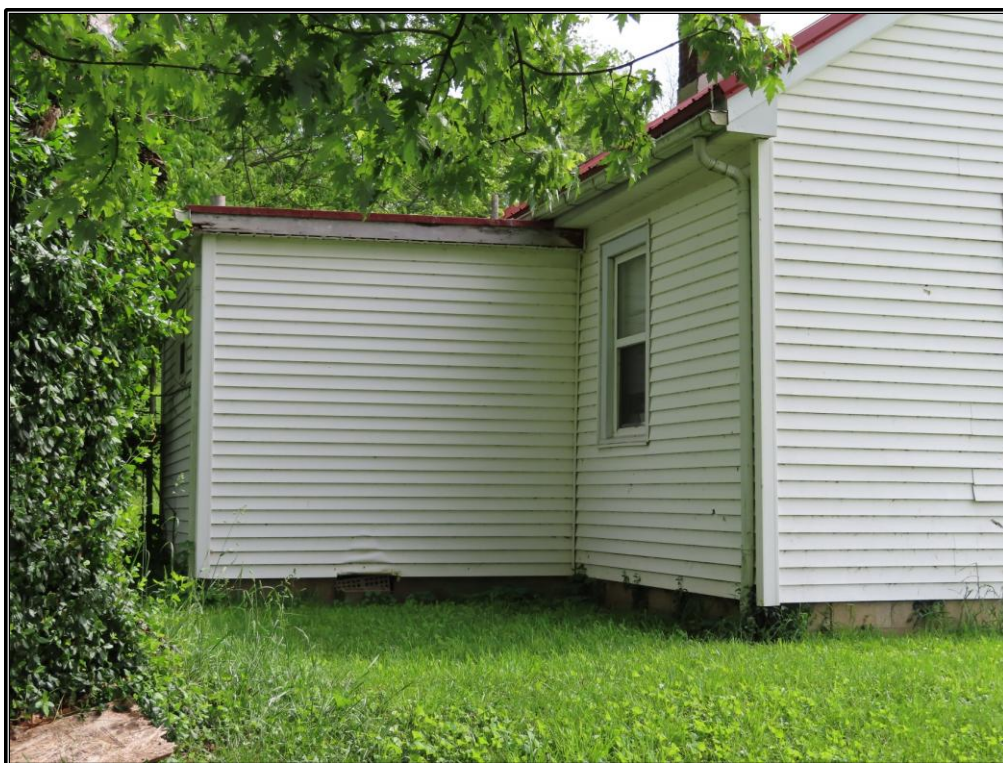
Figure 71. Site 4 (SC 810): Northwest and southwest elevations of the residence, looking east-northeast.
