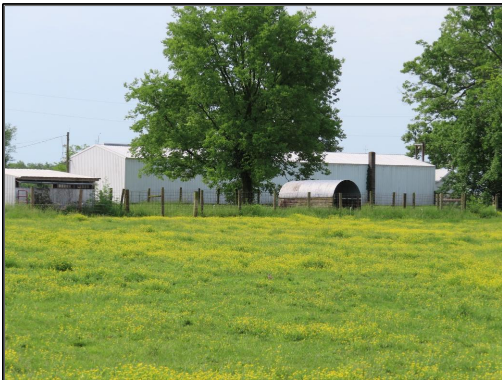
Figure 19. Site 1 (SC 808): Southwest and northwest elevations of the barn (Resource B), looking east-northeast.
