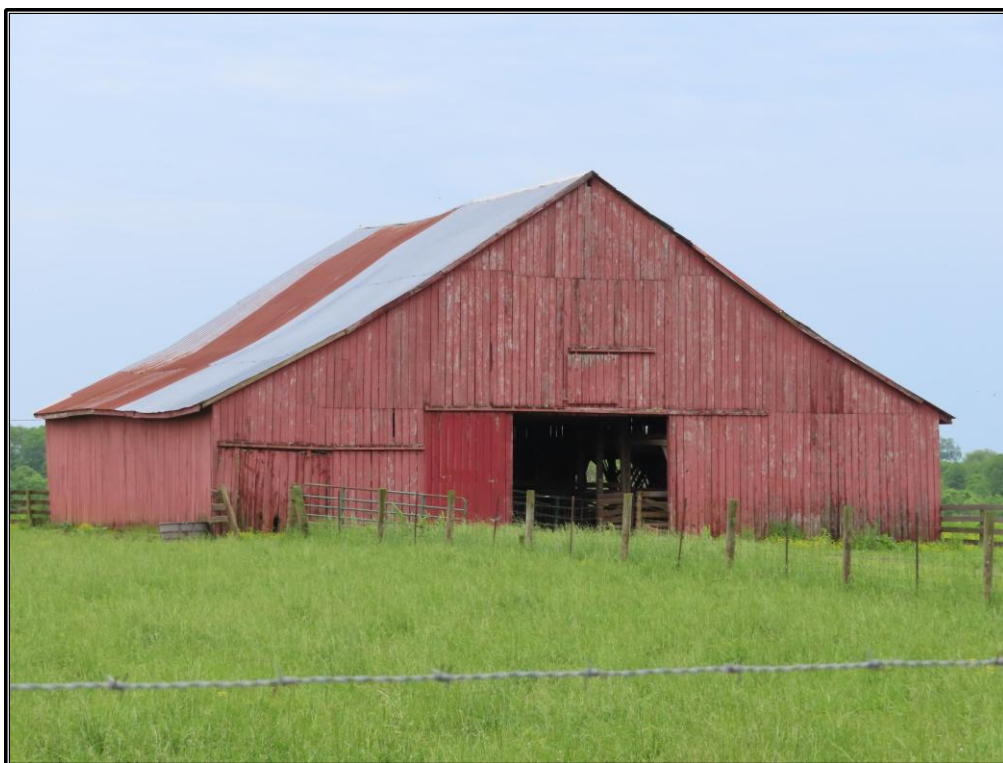
Figure 141. Site 10 (SC 150): Northwest and northeast elevations of the barn (Resource M), looking south.
