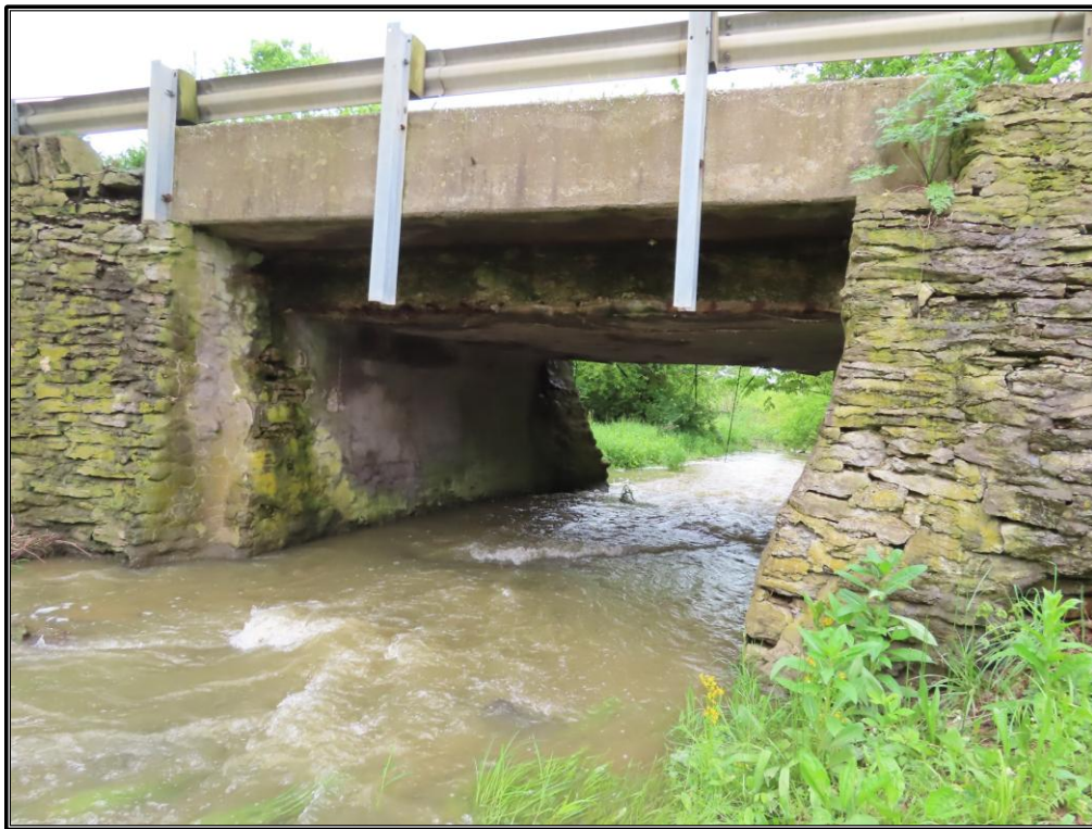
Figure 170. Site 11 (SC 817): View of the substructure and abutments, looking southwest.
