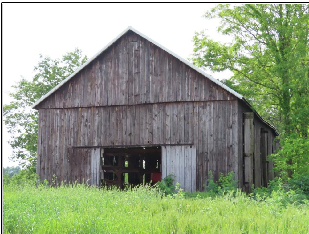
Figure 39. Site 3 (SC 173): East and north elevations of the barn (Resource C), looking west-southwest.
