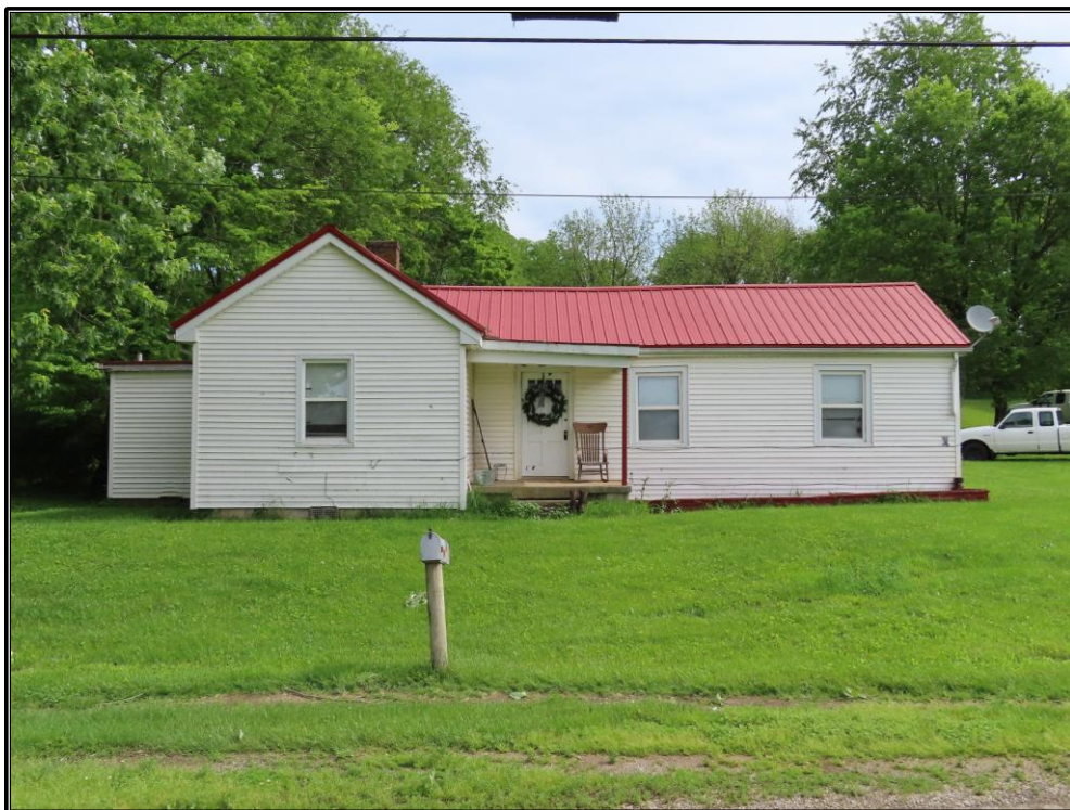
Figure 69. Site 4 (SC 810): Façade of the residence, looking northeast.
