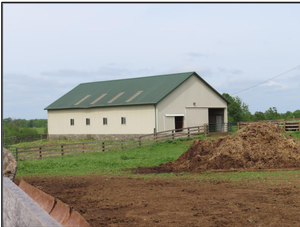
Figure 59. Site 3 (SC 173): South and west elevations of the barn (Resource L), looking northeast.
