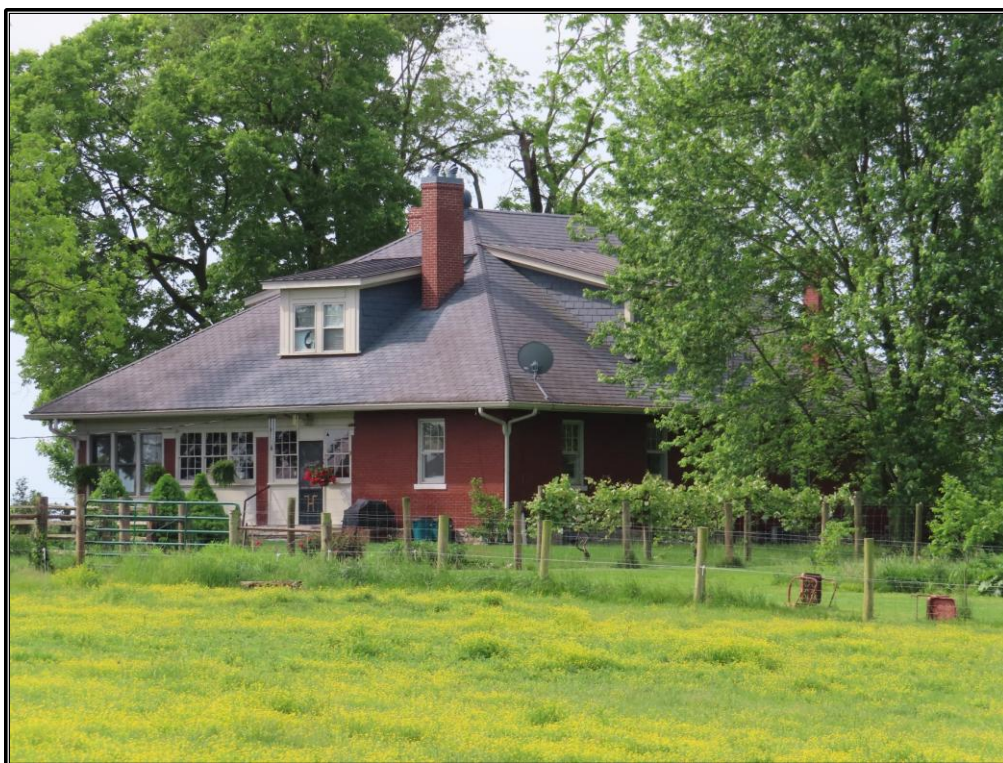
Figure 16. Site 1 (SC 808): Northeast (rear) and northwest elevations of the residence, looking south.
