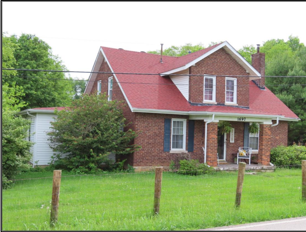
Figure 76. Site 5 (SC 811): Façade and northwest elevation of the residence, looking east.
