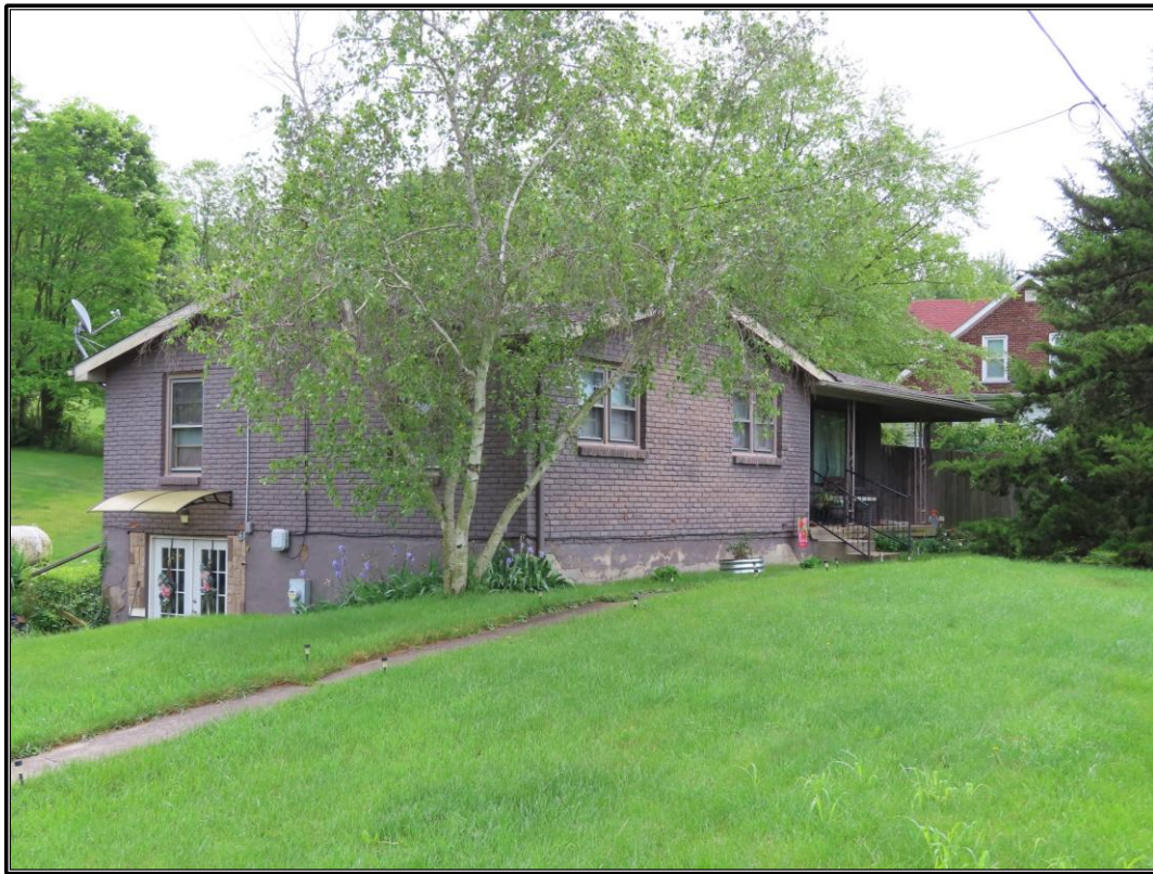
Figure 80. Site 6 (SC 812): Façade and northwest elevation of the residence, looking east.
