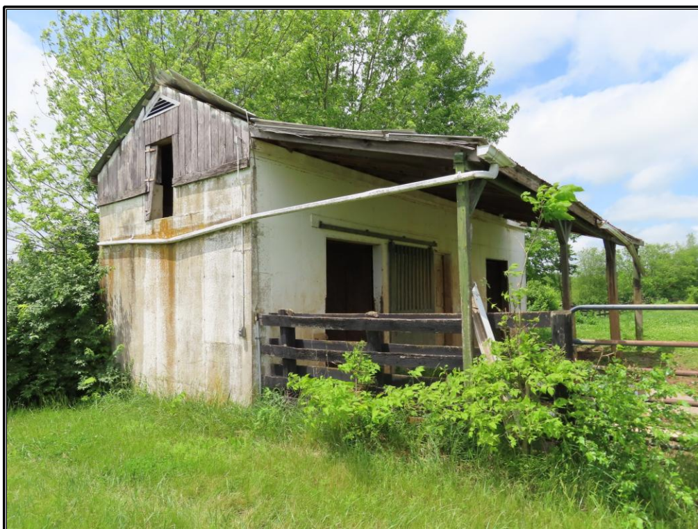
Figure 133. Site 9 (SC 814): East and south elevations of the stable (Resource D), looking northwest.
