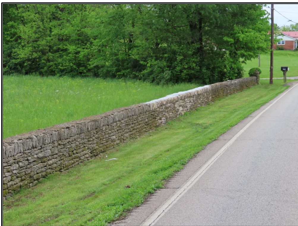
Figure 150. Site 10 (SC 150): View of the stone fence (Resource W), looking southeast.
