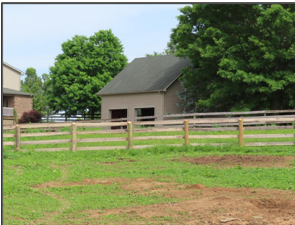
Figure 56. Site 3 (SC 173): Northwest and northeast elevations of the garage (Resource J), looking south.
