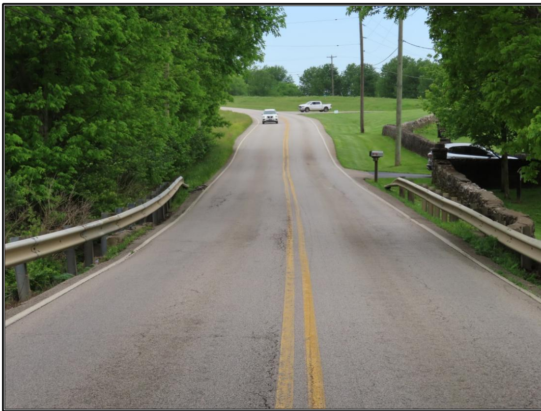
Figure 169. Site 11 (SC 817): View of the deck and railing, looking northwest.
