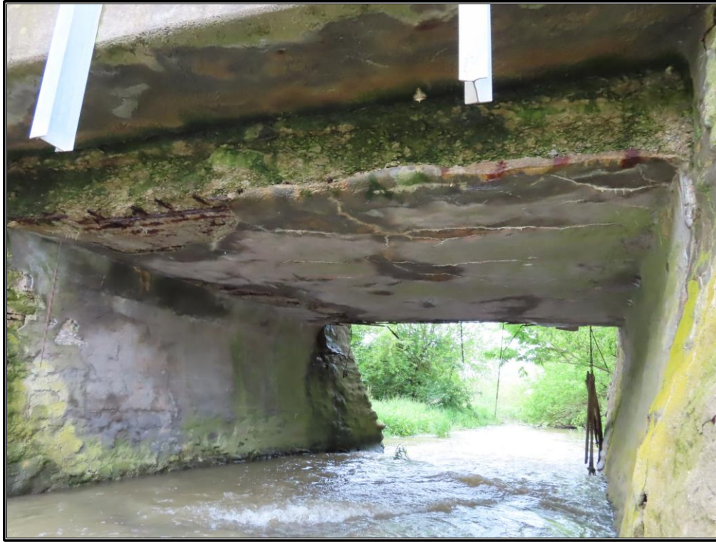
Figure 172. Site 11 (SC 817): Detail of the reinforced concrete deck.
