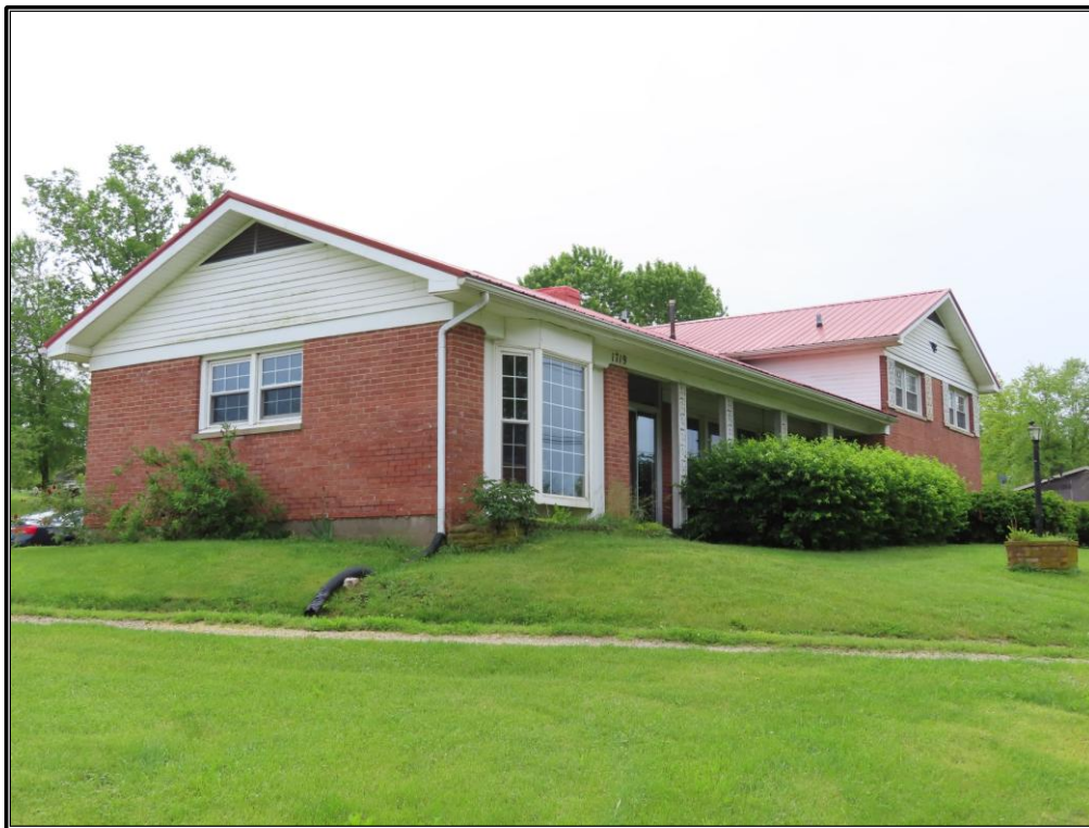
Figure 83. Site 7 (SC 813): Façade and northwest elevation of the residence, looking east.
