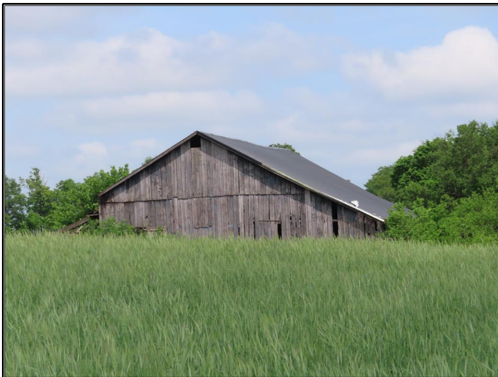
Figure 42. Site 3 (SC 173): West and north elevations of the barn (Resource D), looking southeast.
