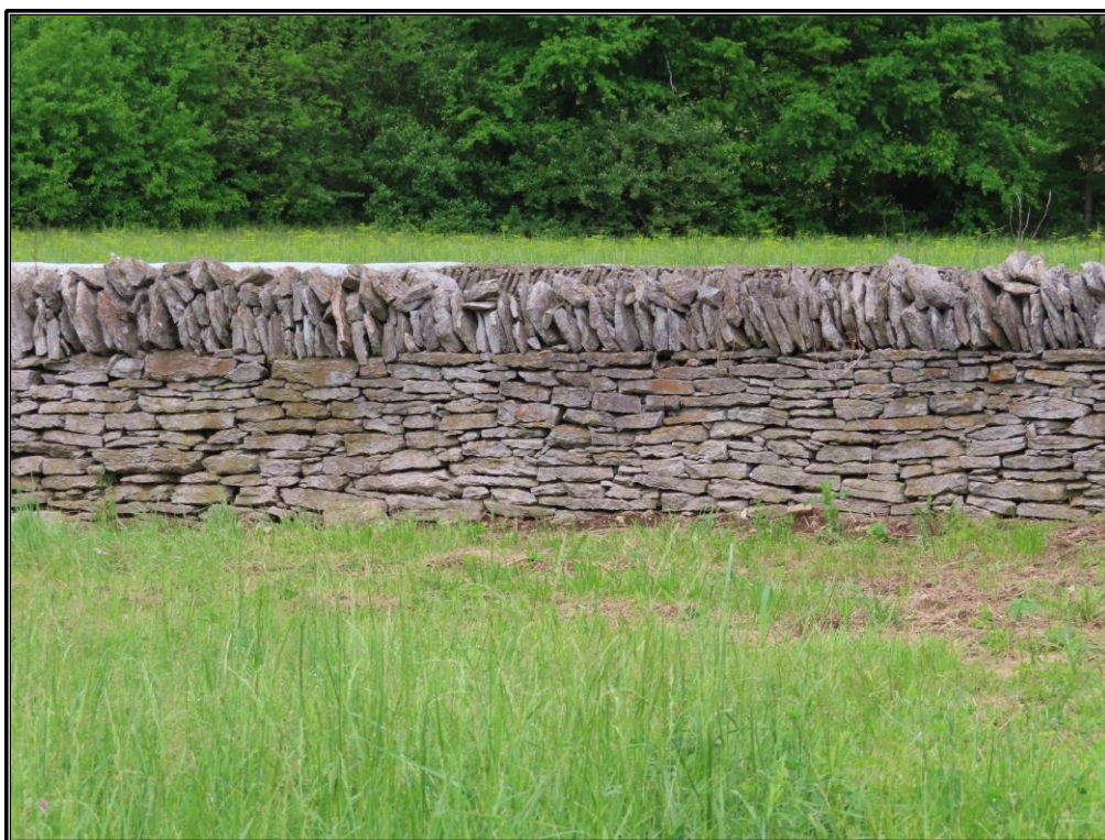
Figure 114. Site 8 (SC 174): Detail of the stone fence (Resource G).
