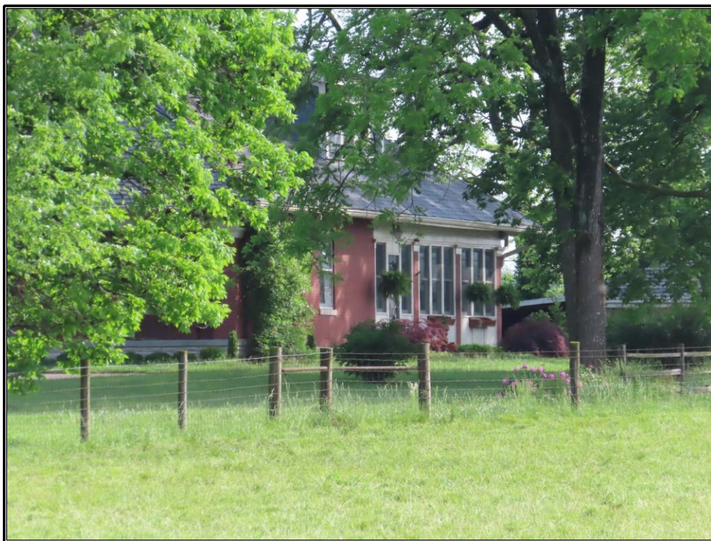
Figure 15. Site 1 (SC 808): Southeast elevation of the residence, looking north-northwest.
