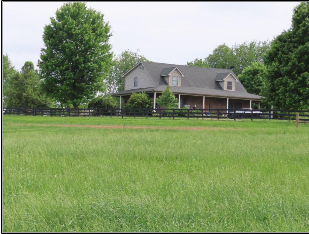
Figure 57. Site 3 (SC 173): Façade and northeast elevation of the modern residence (Resource K), looking south.
