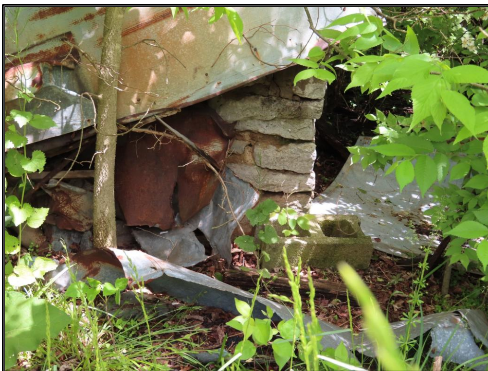
Figure 116. Site 8 (SC 174): Detail of a stone pier (Resource H).
