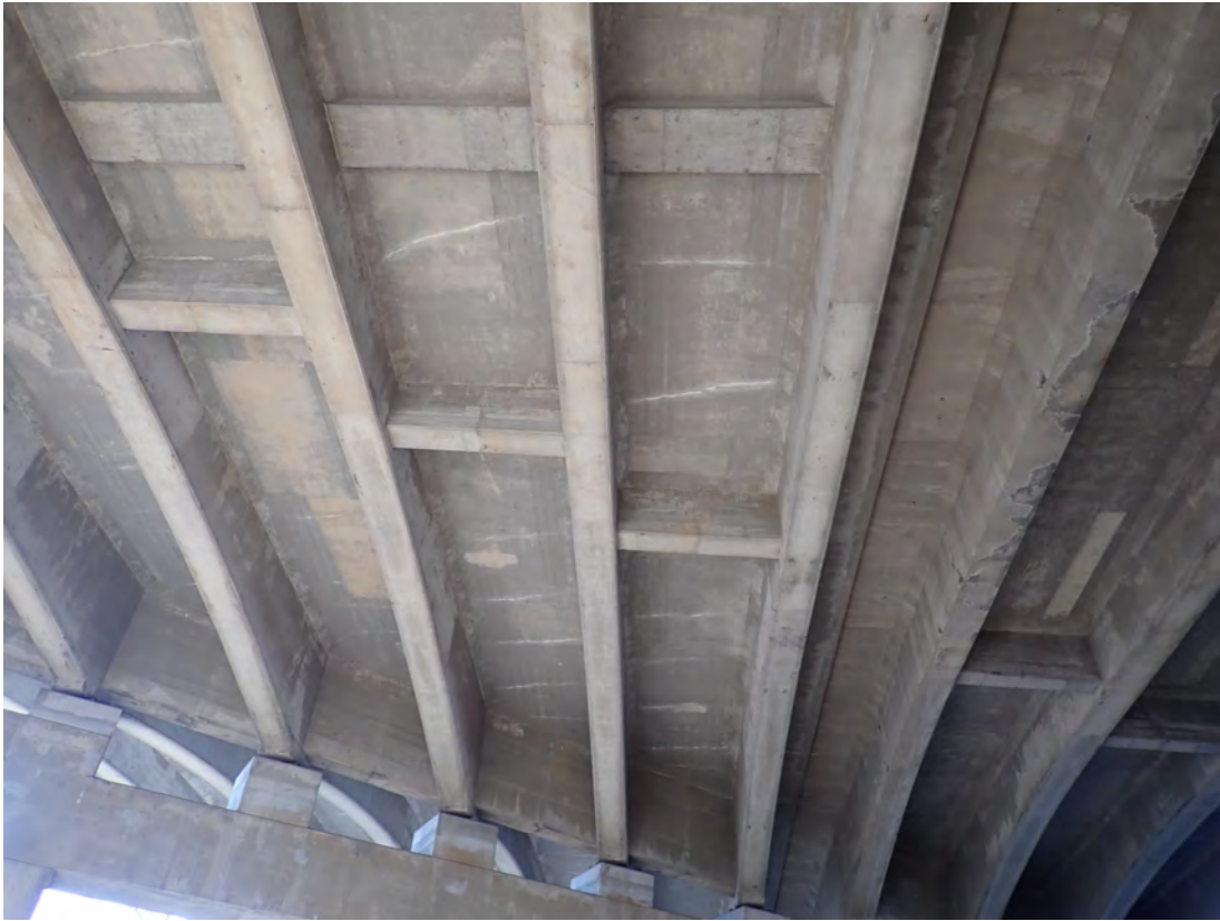
Span 5 deck soffit under EBL
