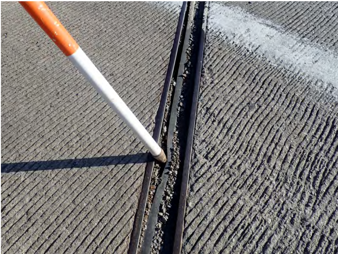
Closer view of compression joint seal over Pier 5 EBL
