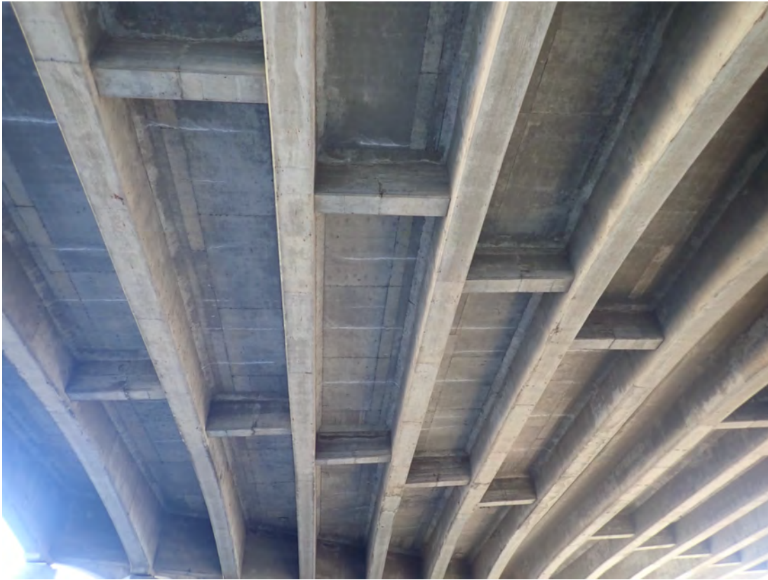
Span 6 deck soffit over WBL
