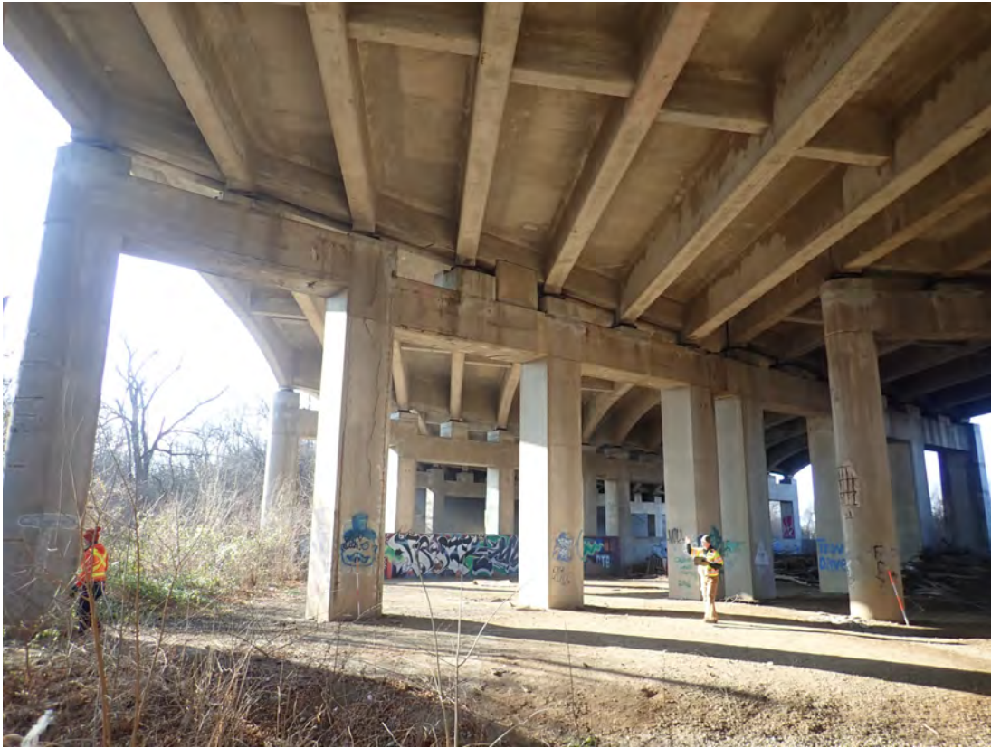
West face Pier 5
