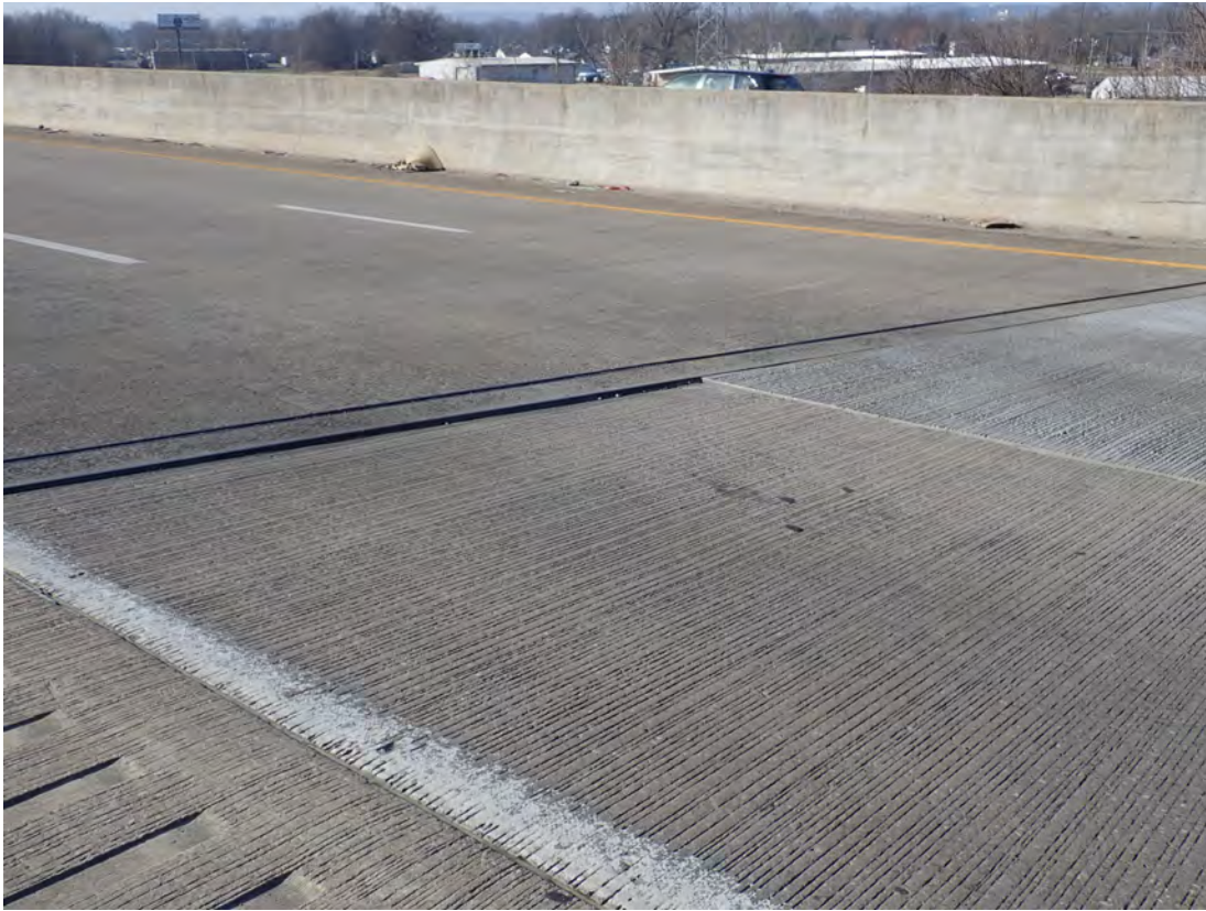
Abutment 1 WBL transition repair left one lane with transition unchanged
