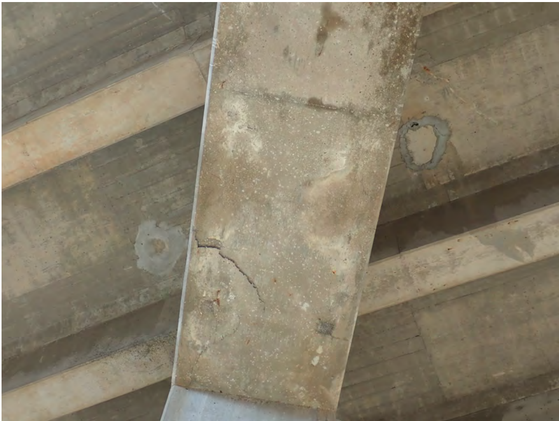
Deck soffit patching over Pier 5
