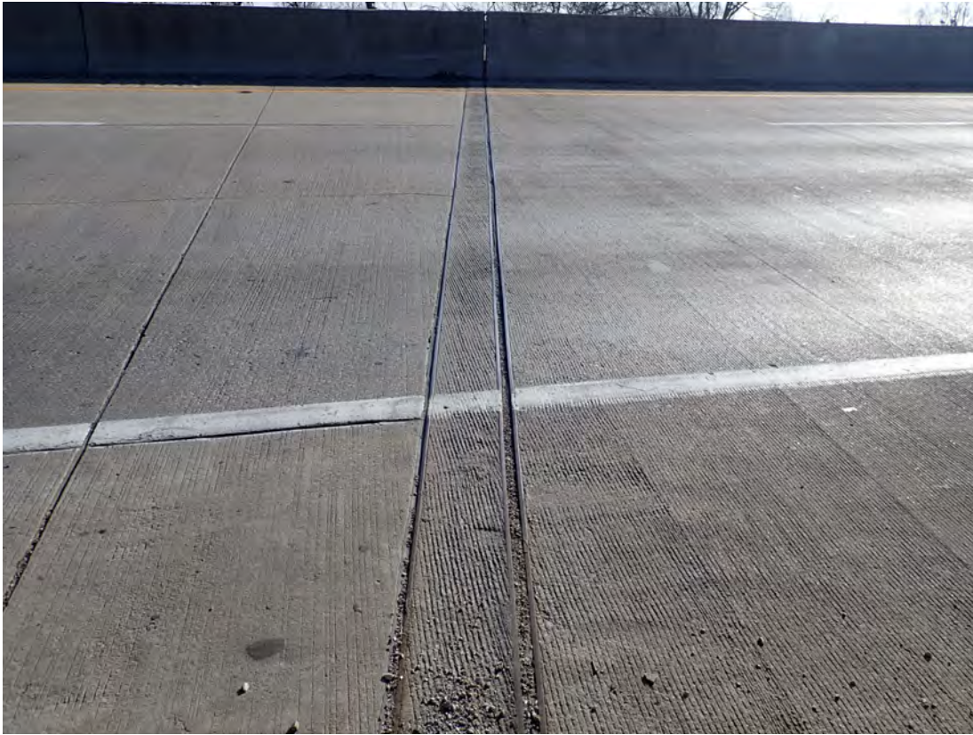
Compression joint seal over Abutment 1 EBL
