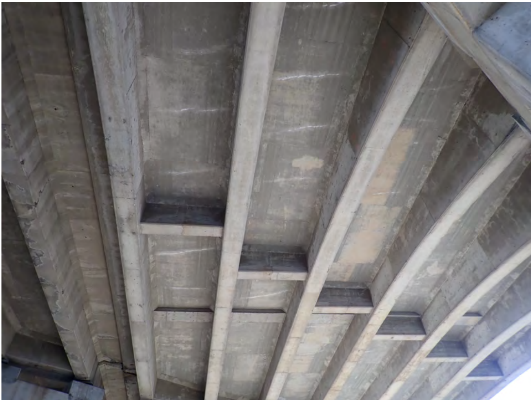
Span 5 deck soffit under WBL
