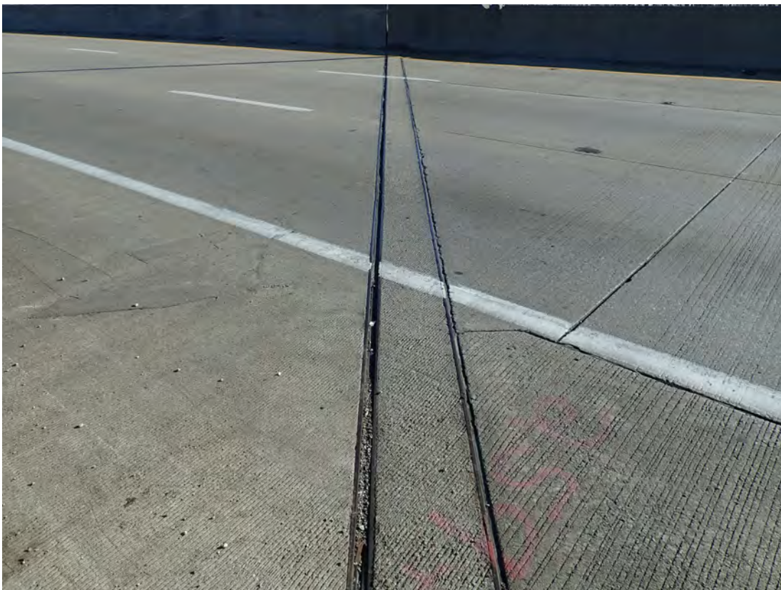
Compression joint seal over Abutment 8 EBL
