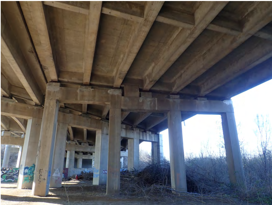
West face Pier 4
