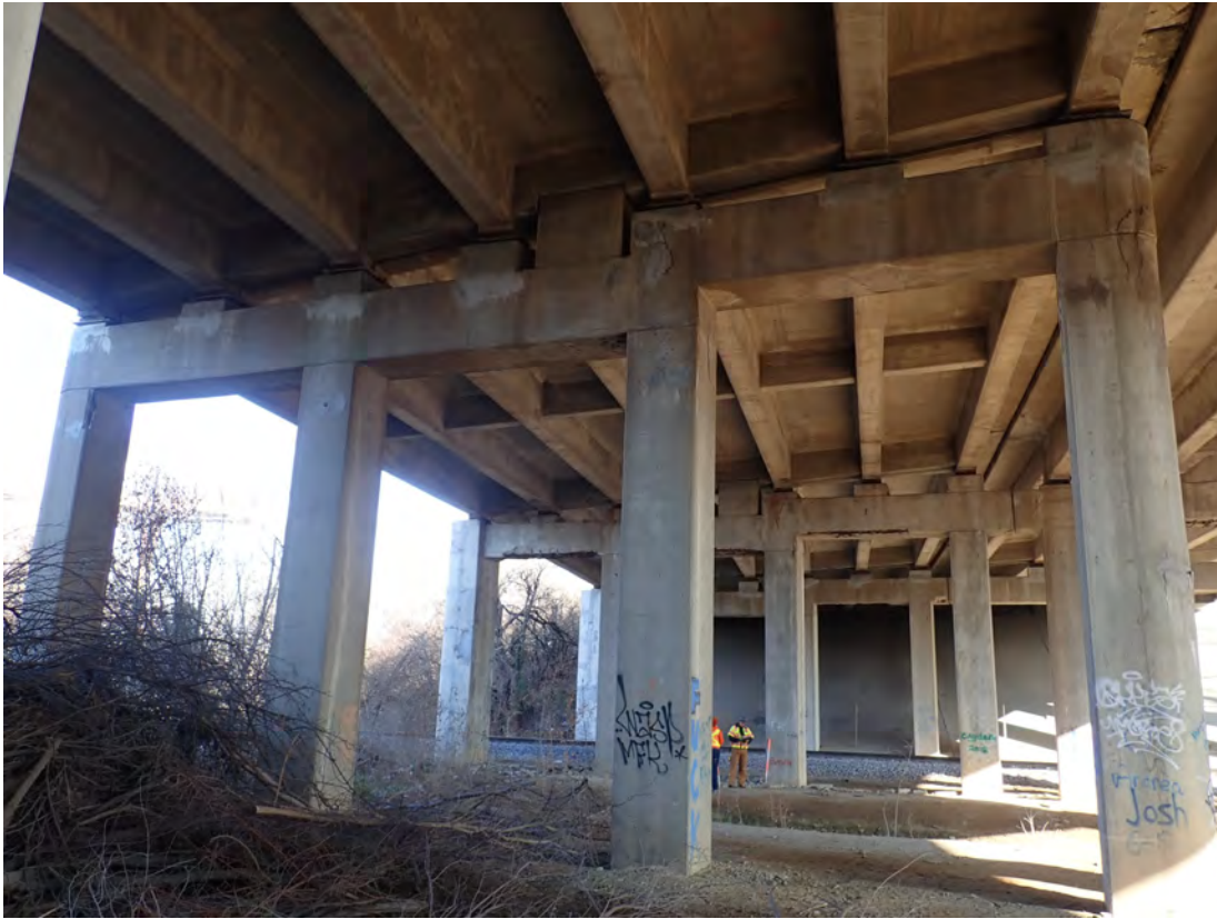
East face Pier 4
