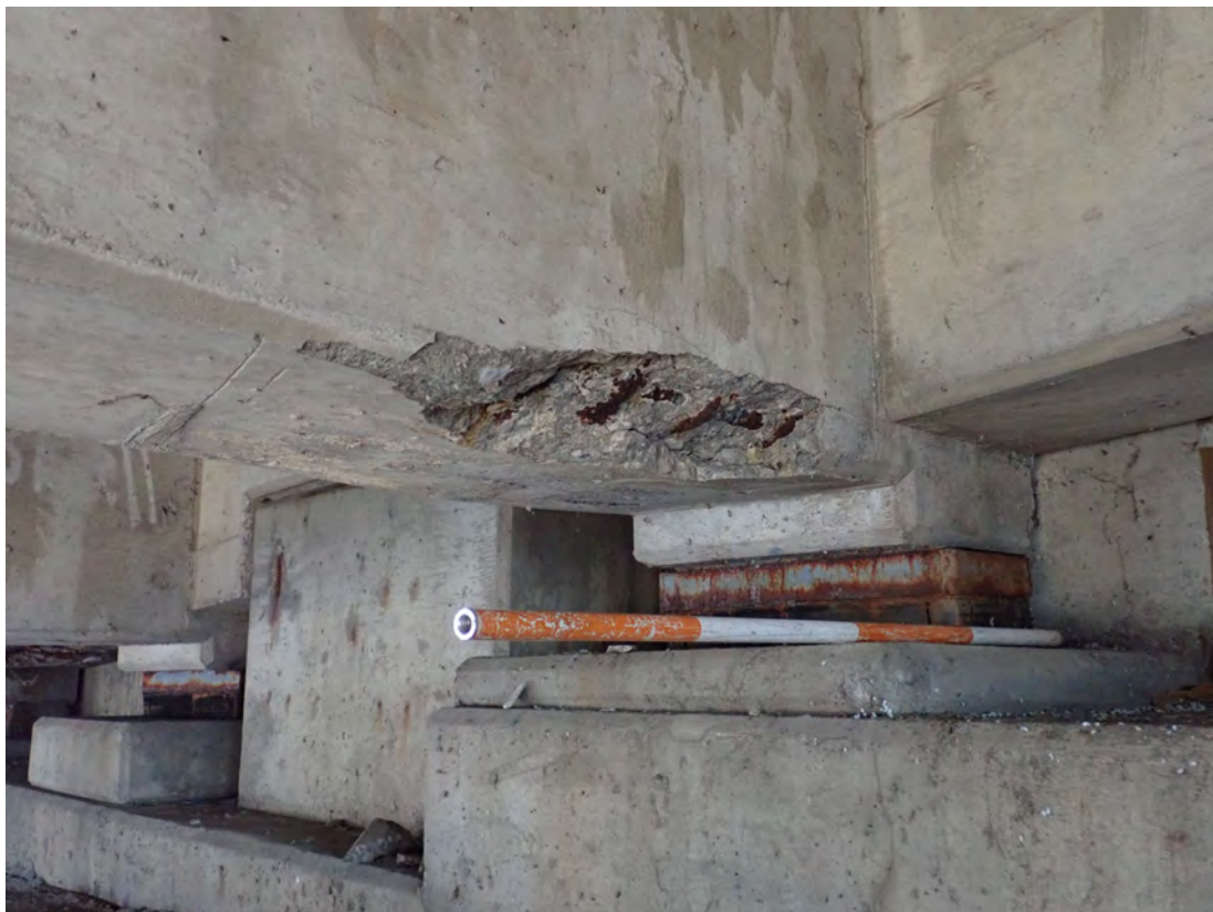
Closer view of Abutment 1-Girders 10
