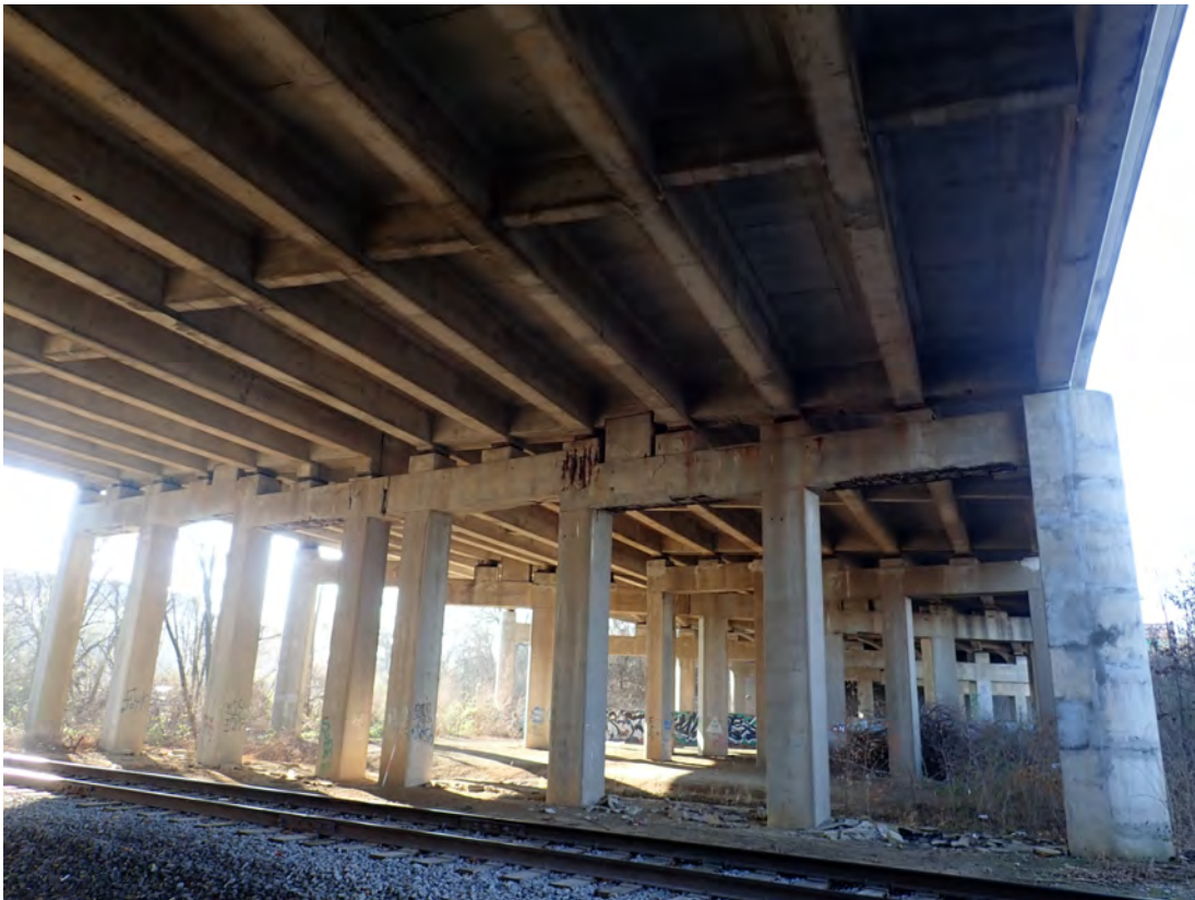
West face Pier 3
