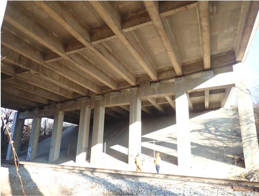
East face Pier 2
