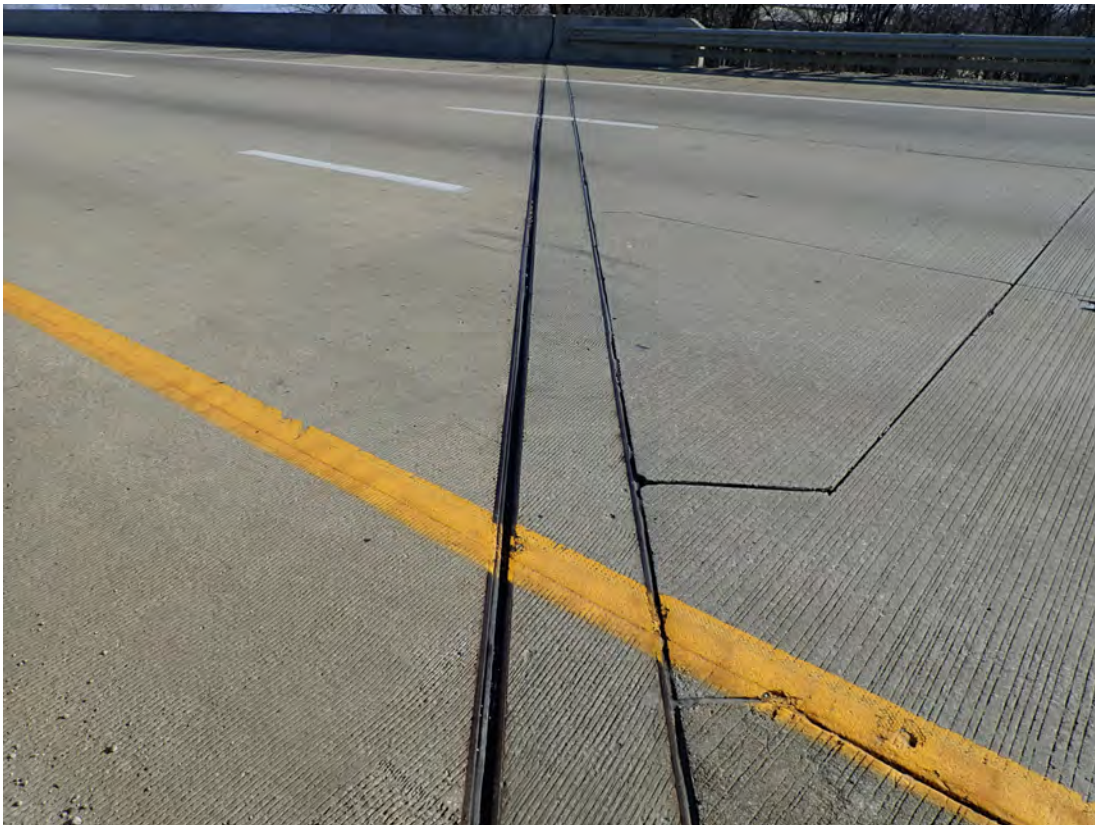
Compression joint seal over Abutment 8 WBL
