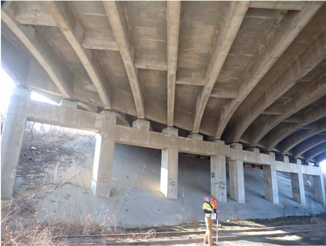
West face Pier 7
