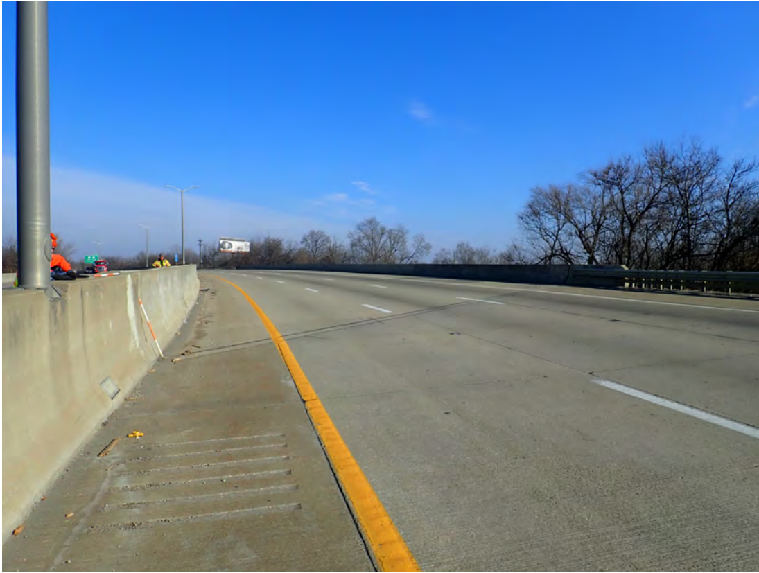
Looking west along I-264 WB toward Bells Lane/KY 2056 over P&L Railway
