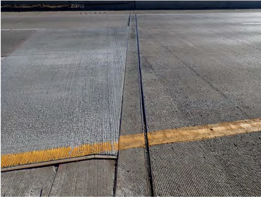
Compression joint seal over Abutment 1 WBL
