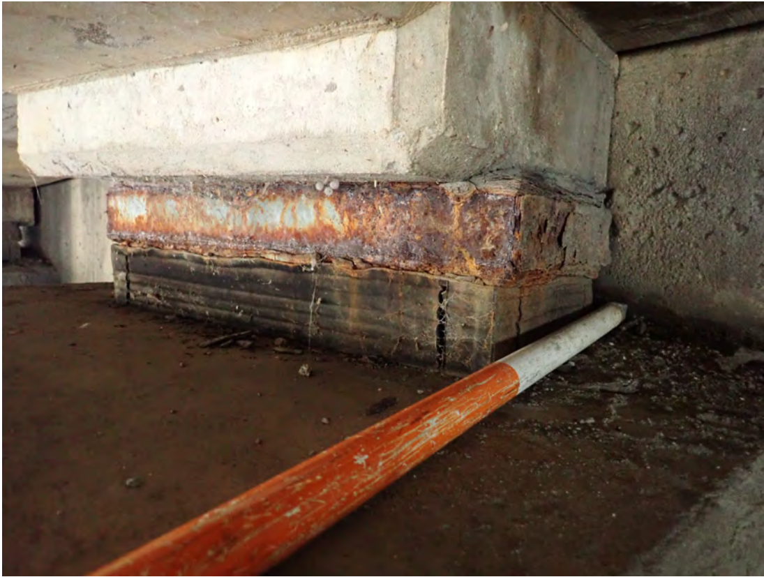
Typical bearing device condition at Abutment 1, showing Beam 12 device
