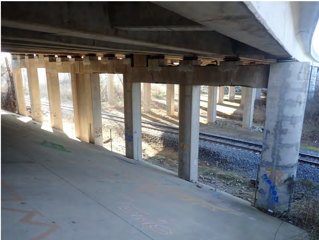
West face Pier 2
