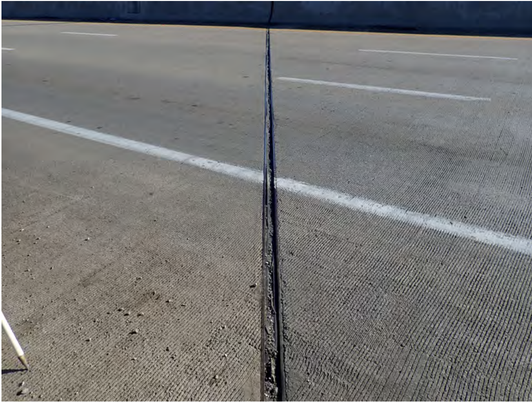
Compression joint seal over Pier 5 EBL
