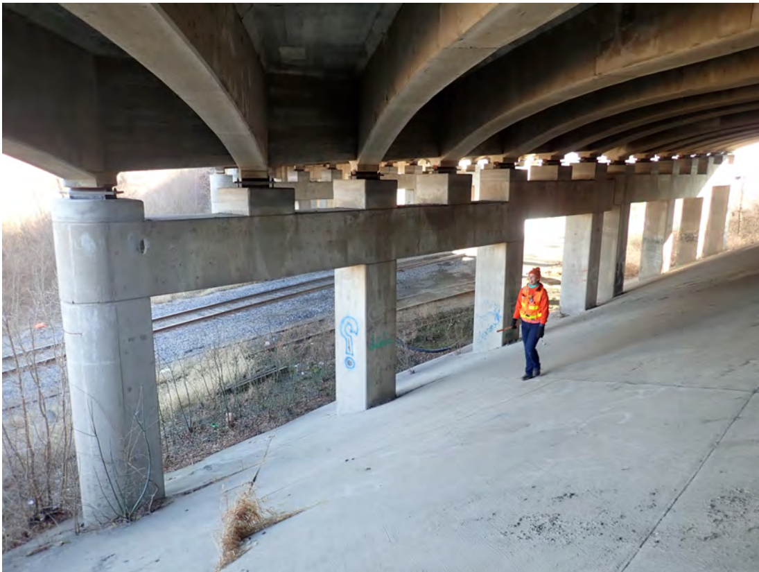
East face Pier 7
