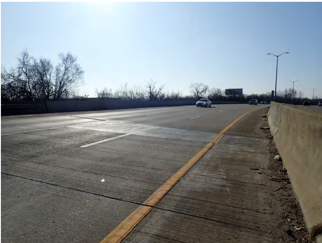
Looking east along I-264 WB toward Cane Run Road/KY 1934 over P&L Railway
