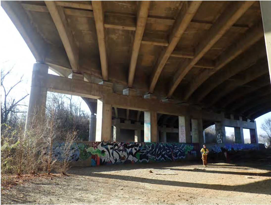
West face Pier 6
