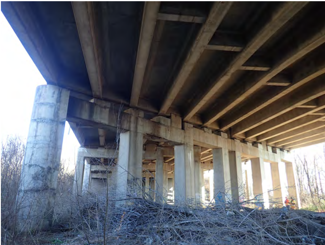
East face Pier 5 and debris pile under Span 5
