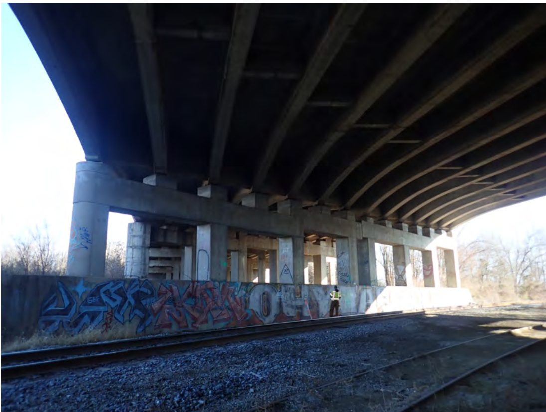
East face Pier 6
