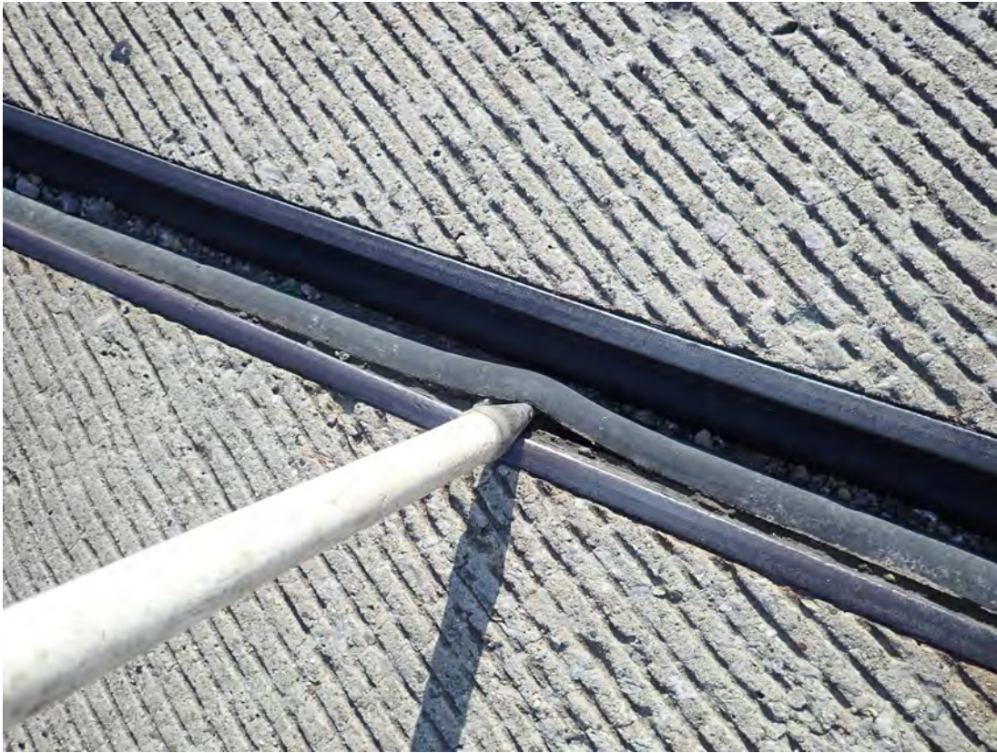
Closer view of compression joint seal over Pier 5 WBL
