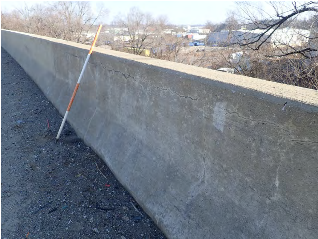
Typical condition of barrier wall
