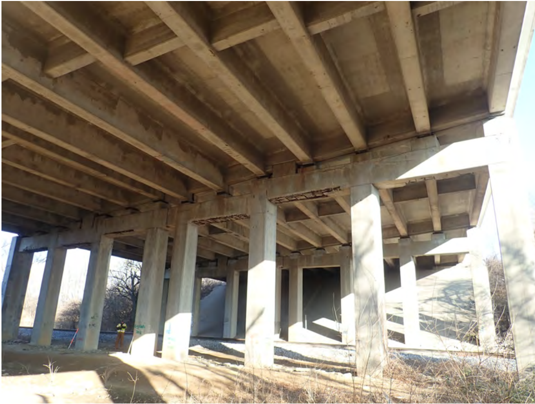
East face Pier 3
