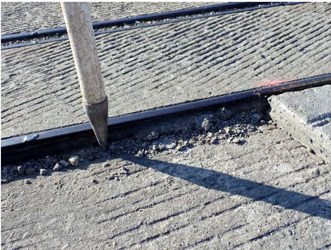
Closer view of transition at Abutment 1 WBL
