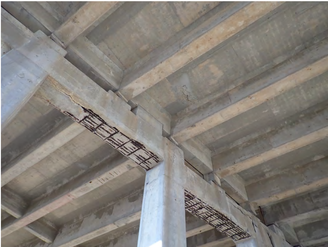
Bottom side of Cap 3 and deck soffit patching near pier
