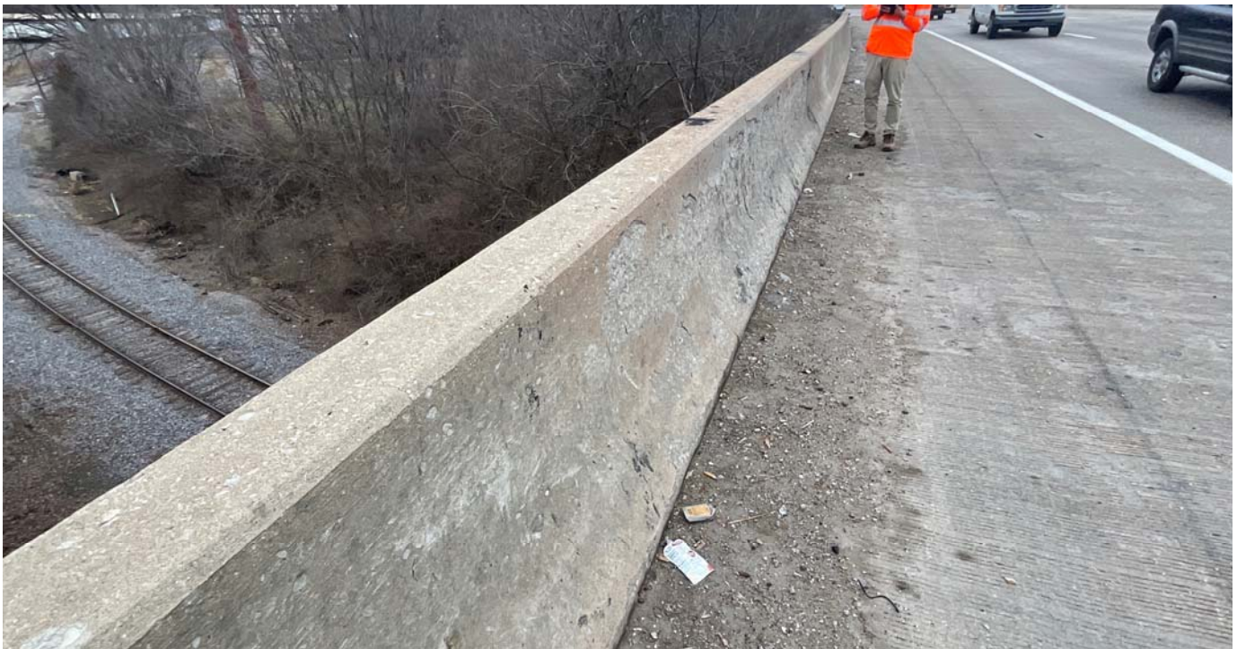
Barrier wall is scaled - EB barrier – Span 2
