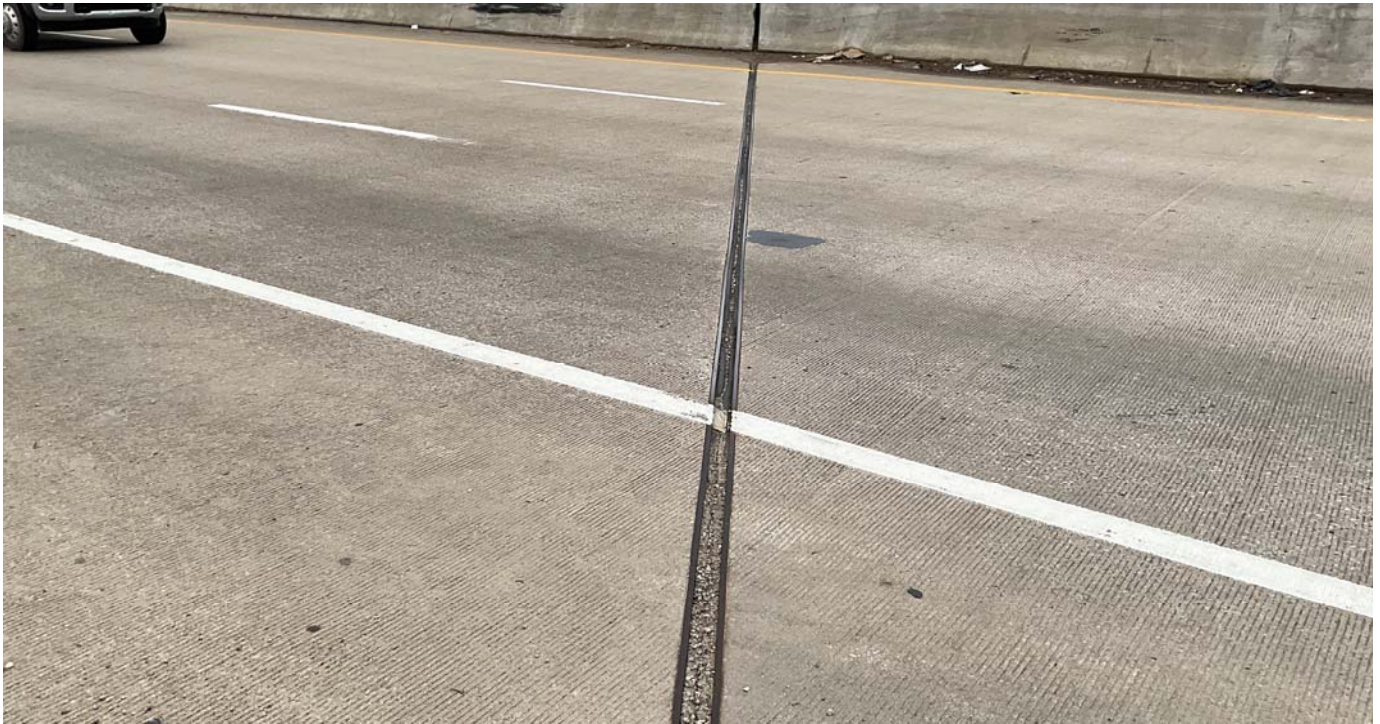
Joint at Pier 5
