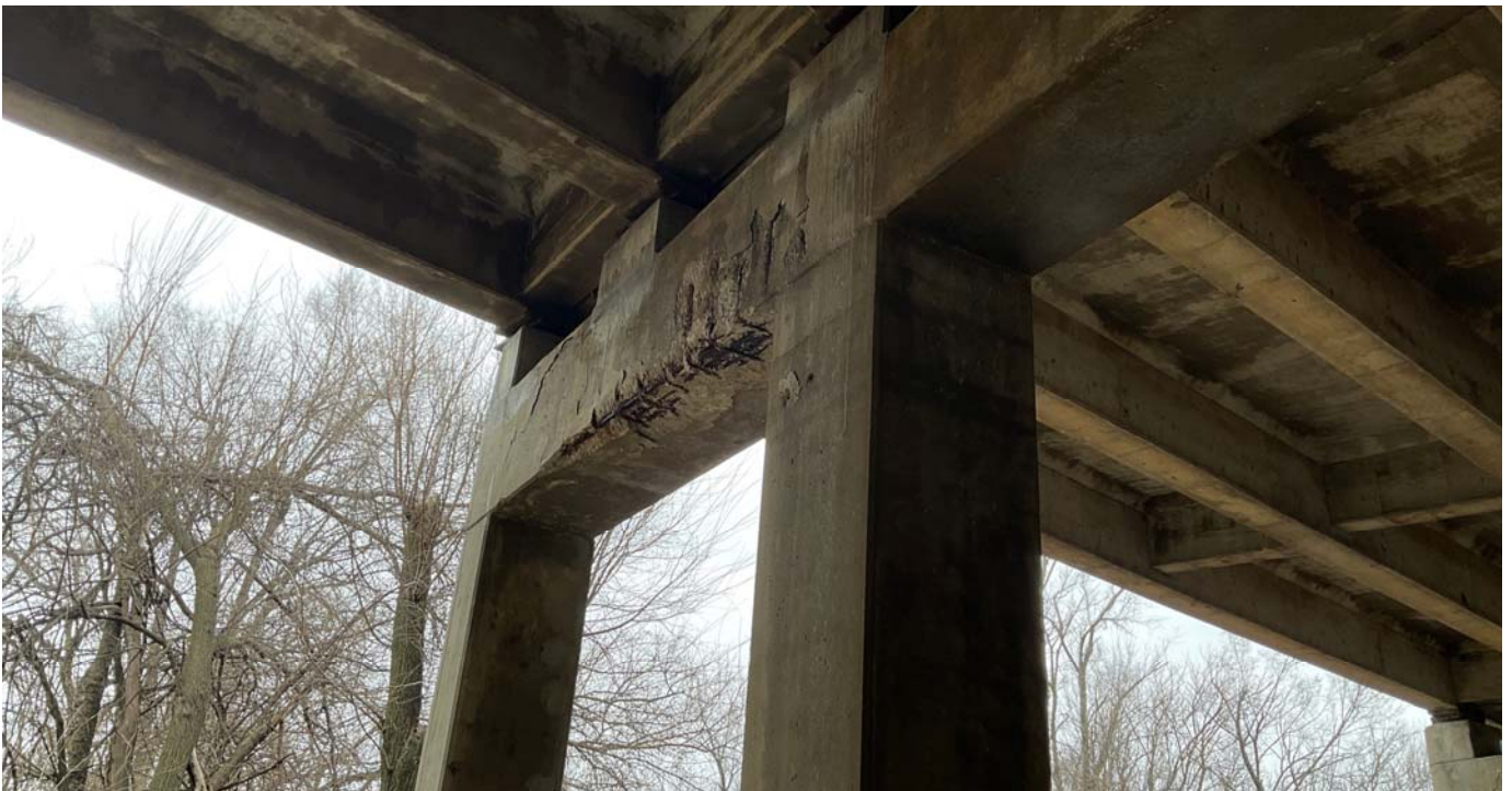
Pier 2 - north end
