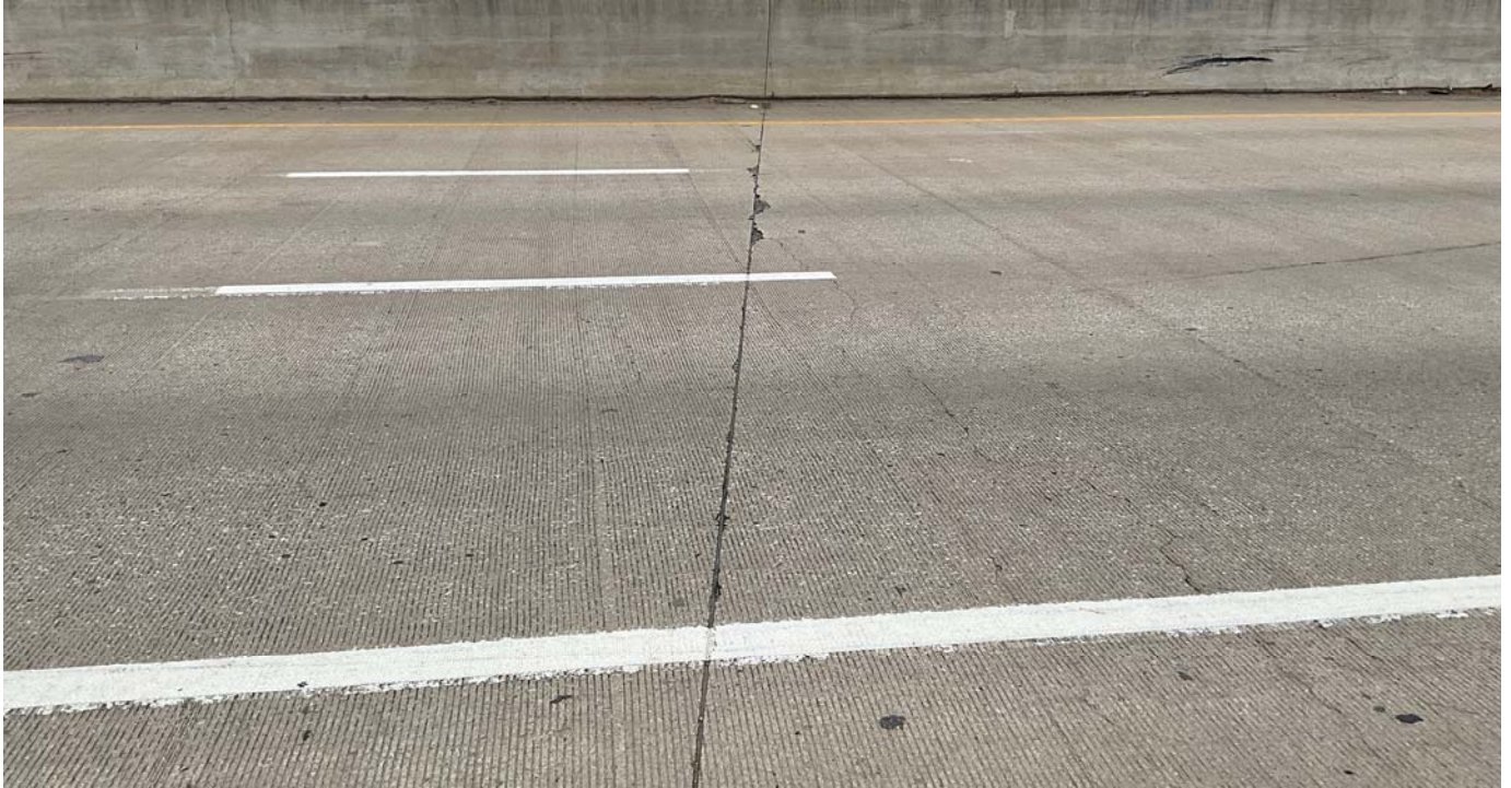
Joint at Pier 2
