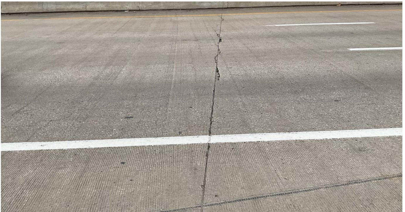
Joint at Pier 3
