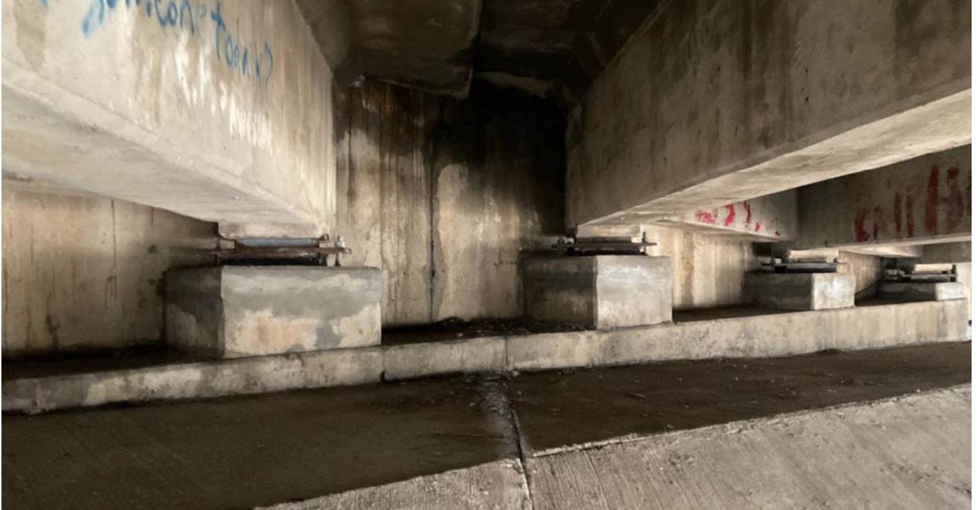
Typical bearing - Abutment 8
