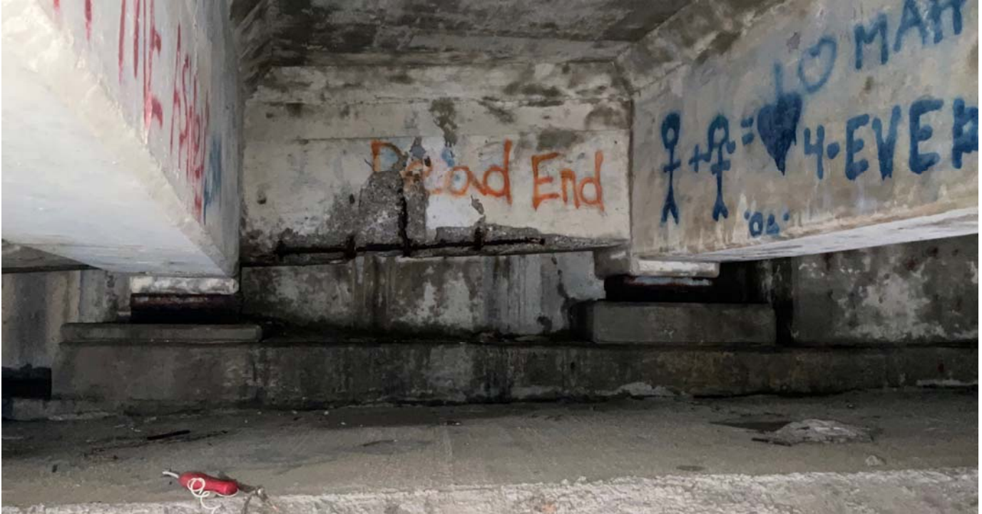
Diaphragm at Abutment 1 between Beams 11 and 12.
