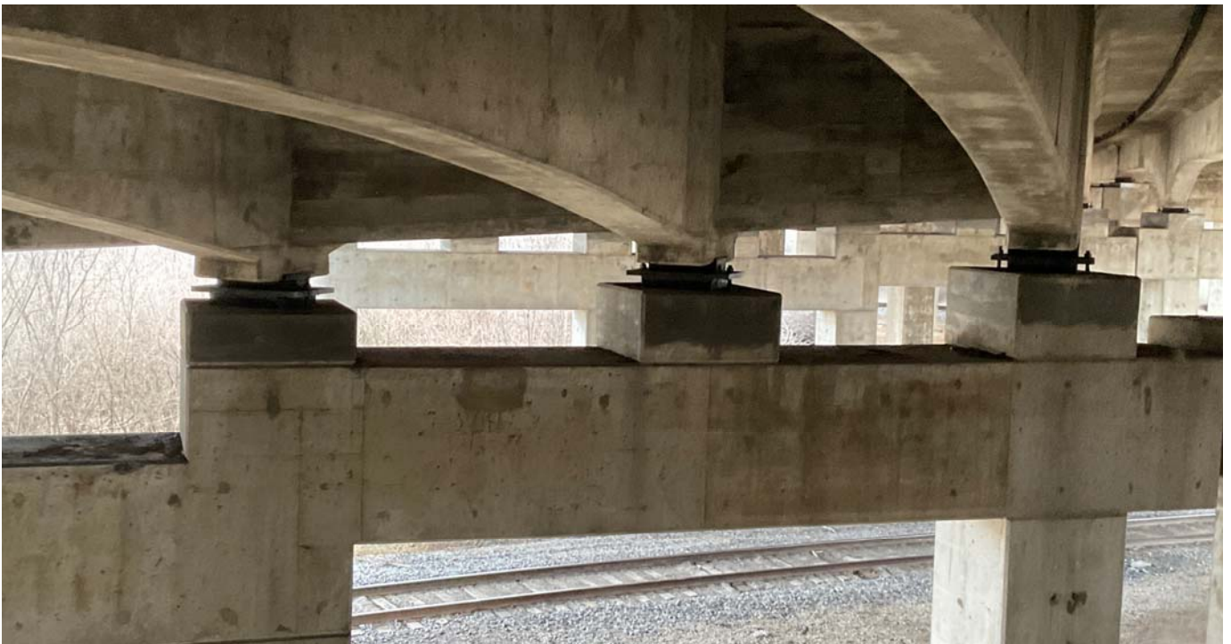
Typical bearing - Pier 7
