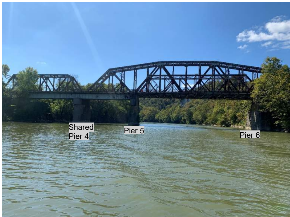
Photo 2 Overview of Bridge Looking Upstream
