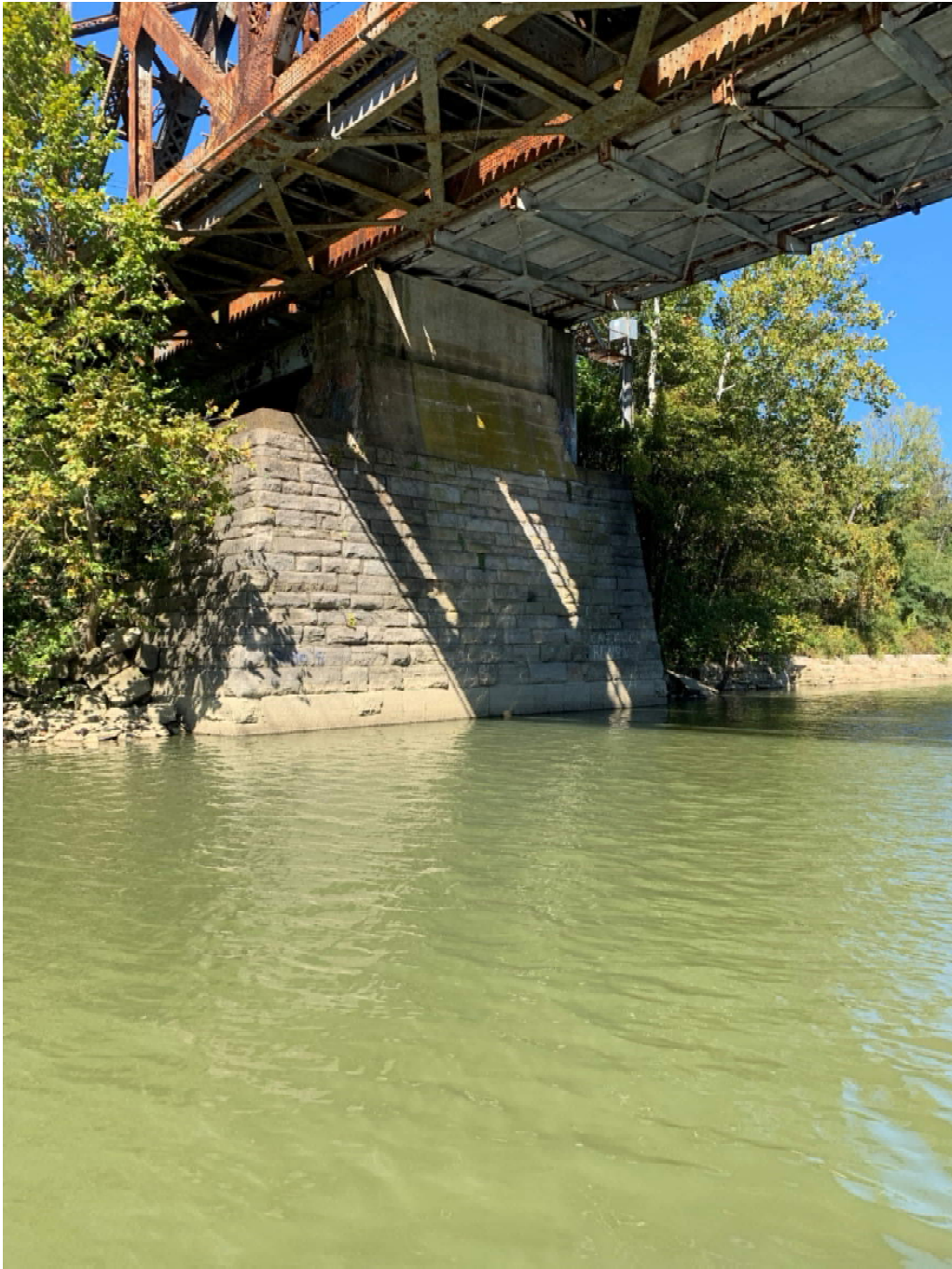
Photo 5 Pier 6 Looking West
