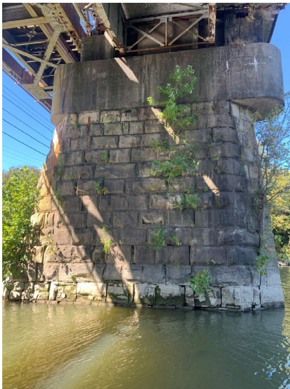
Photo 4 Pier 5 Looking West
