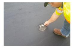
Excessive water in mix. Has a slick and smooth appearance. Debonding has occurred and is very slow to cure.
