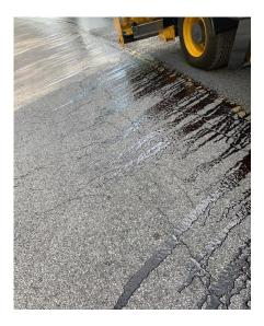
Emulsion shouldn't be running off roadway or into adjacent lane. If you see this you need to stop production. Check temperature of emulsion and/or sample for viscosity.
