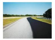
Fog seal on a chip seal. Improves appearance, locks in any remaining loose aggregate and improves visibility of striping.
