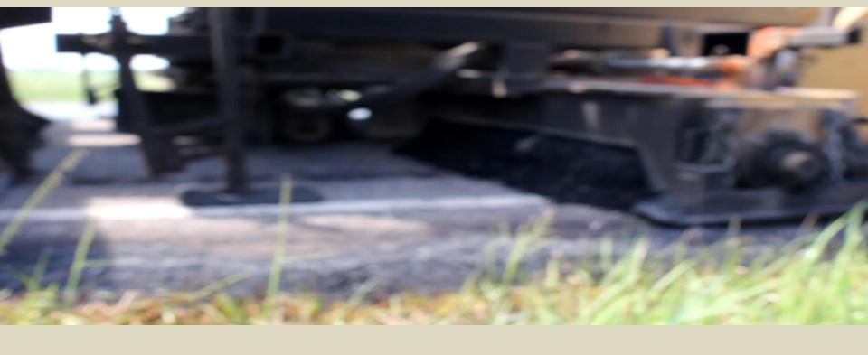
Next is the first milling heater which will continue to heat the roadway and remove the first lift of material and windrow it. Removing the material at ½" increments.
