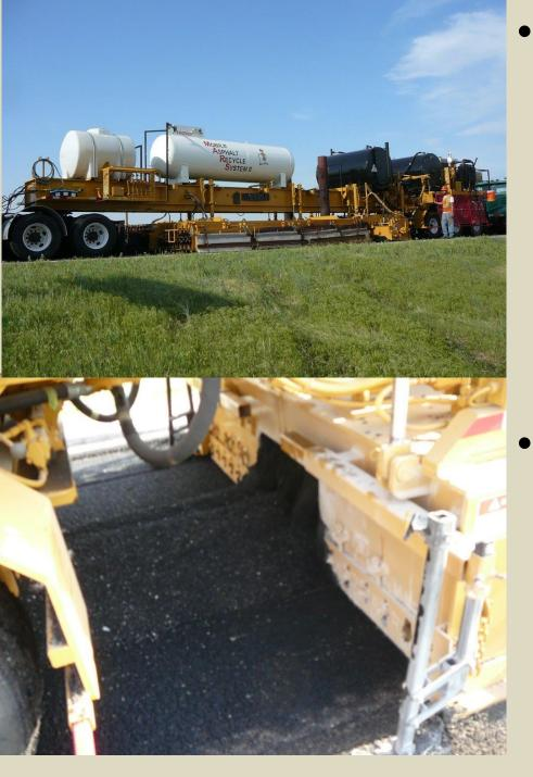
The last set of heating units is another tunnel heater followed by a milling heater with an emulsion system on board.
