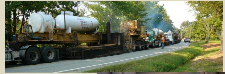
One to two more sets of Preheaters and Milling heaters with Tunnel ovens will be used to remove the existing asphalt in lifts to maintain heat.
