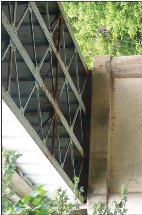
094B00003N ~ UNDERSIDE VIEW (Looking West)
