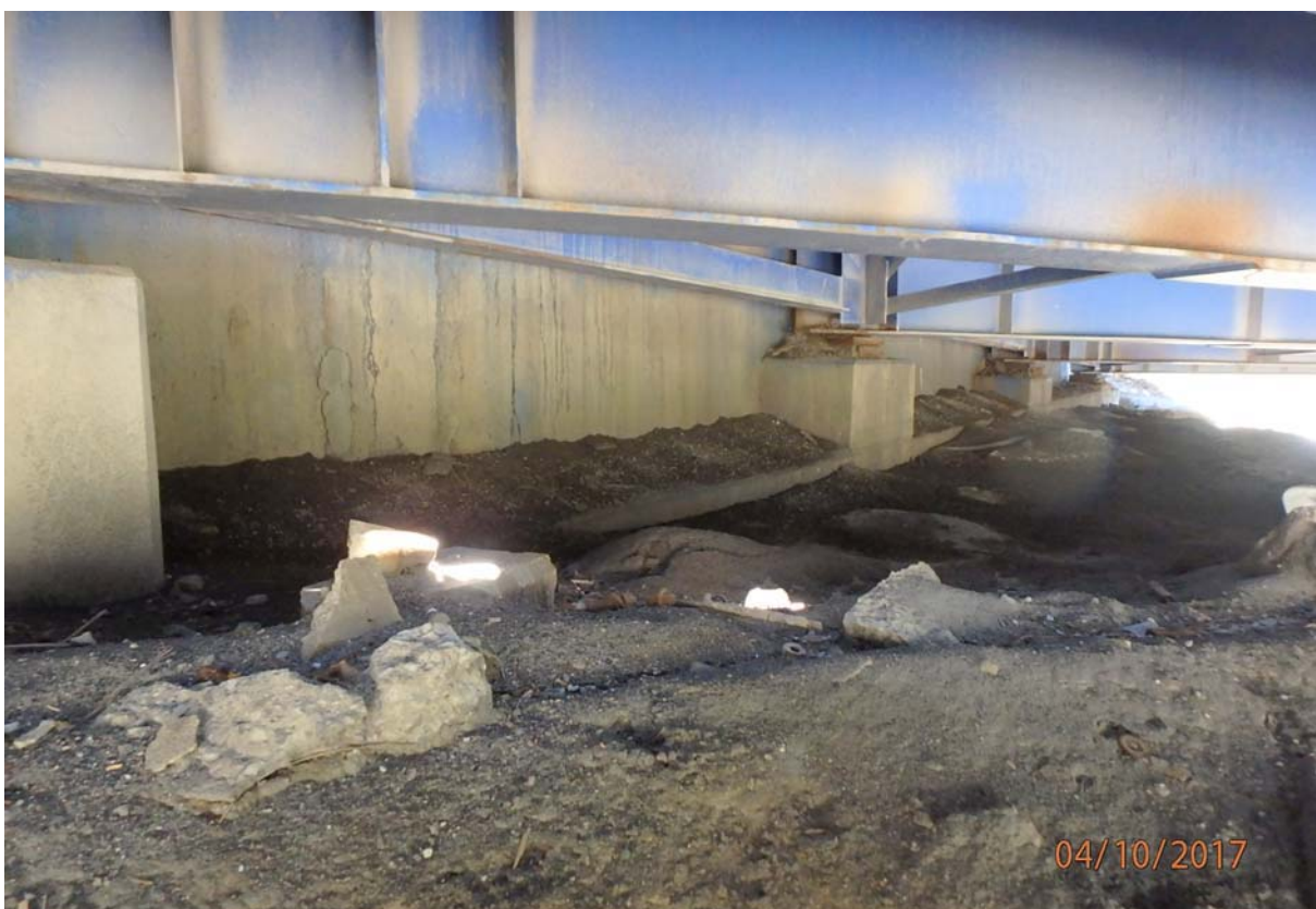
Abut 6 is in good condition.
