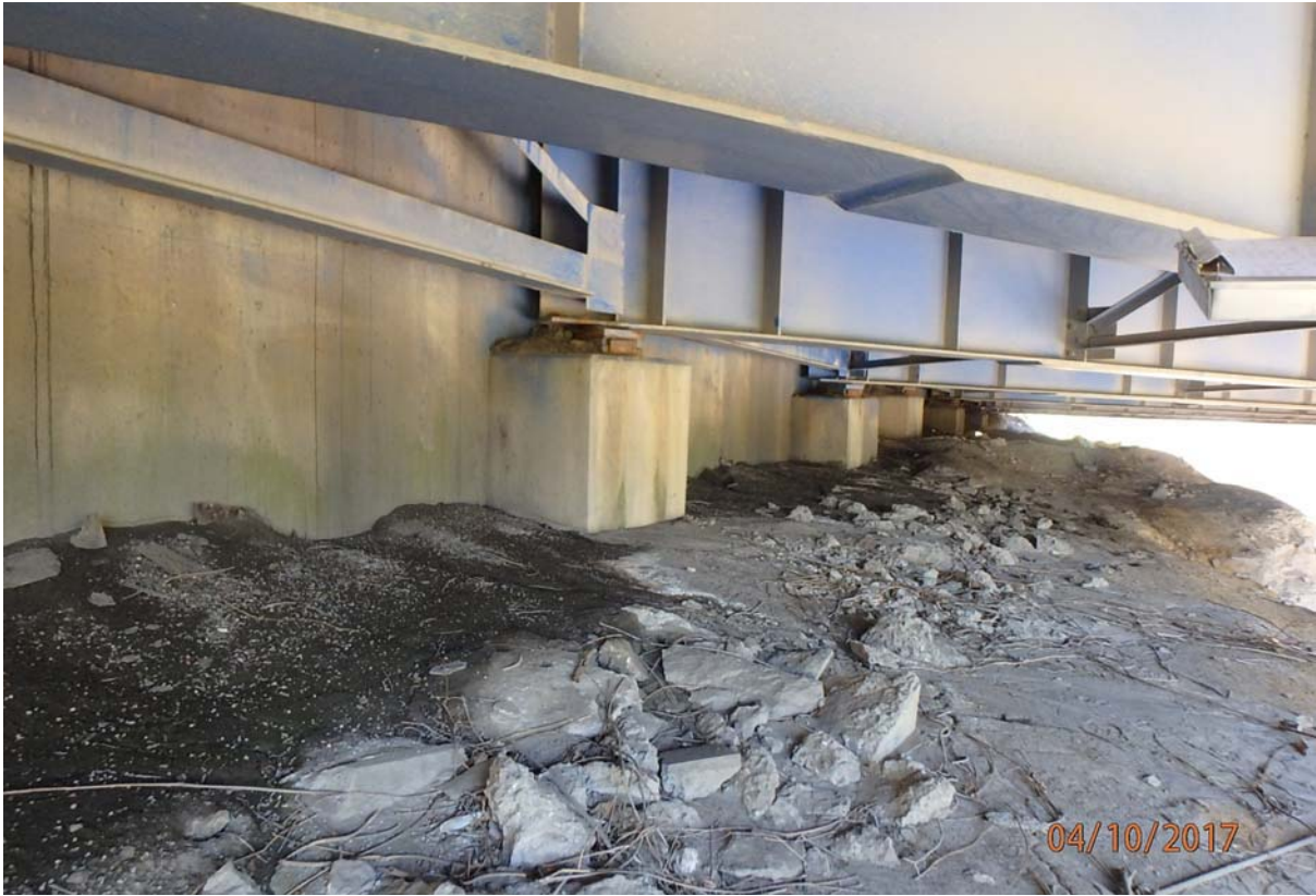
Abut 6 is in good condition
