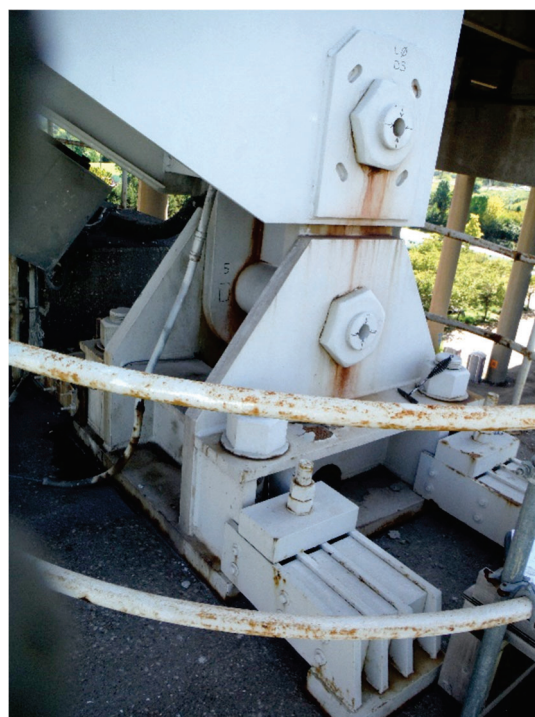
Figure 1 - DOWNSTREAM TRUSS BEARING AT PIER 1L
