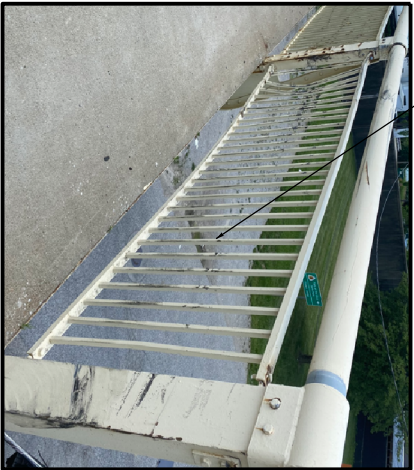
Replace Railing Panel
