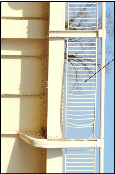
Replace Railing Panel
