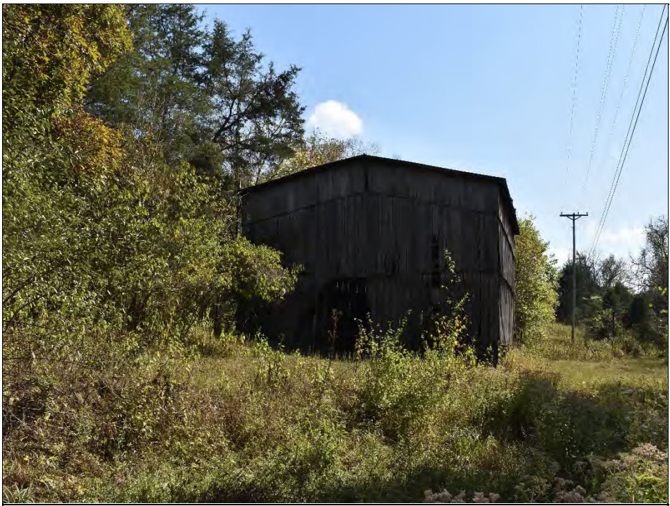
Photo 1: North elevation of barn at 0 McDonald Road.
