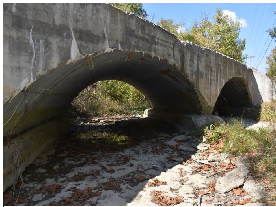
Photo 8: Upstream profile (west elevation) of Bridge No. 003B00041N.
