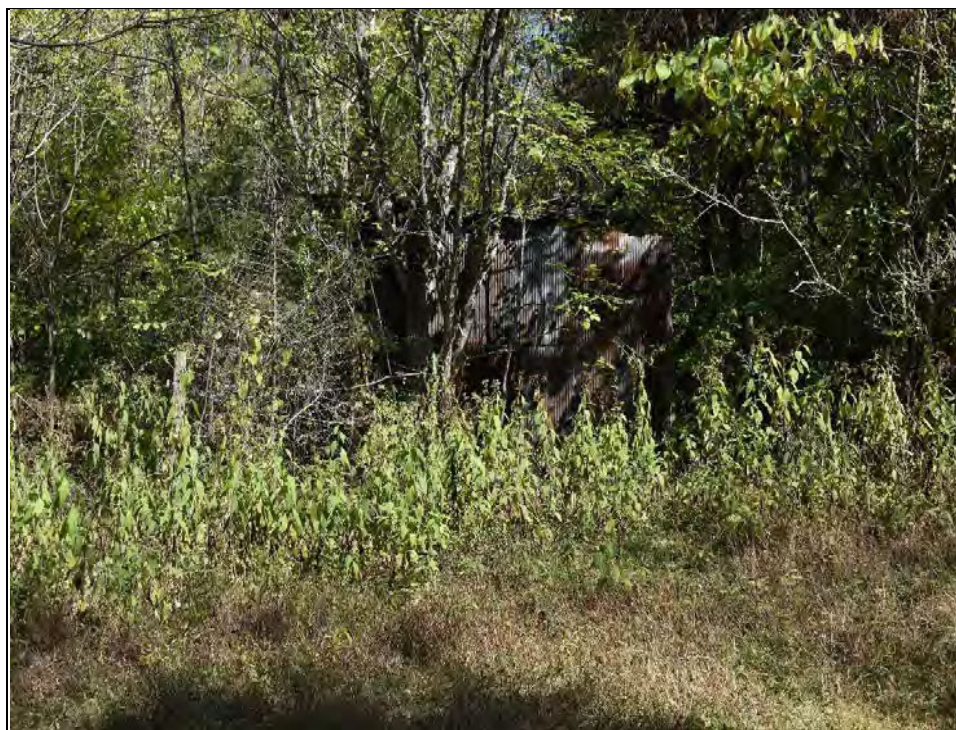
Photo 7: Facing east toward metal building.
