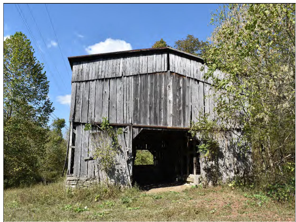
Photo 4: South elevation of barn at 0 McDonald Road.
