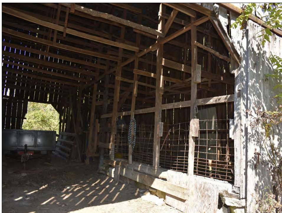
Photo 6: Interior pens on east wall of barn.
