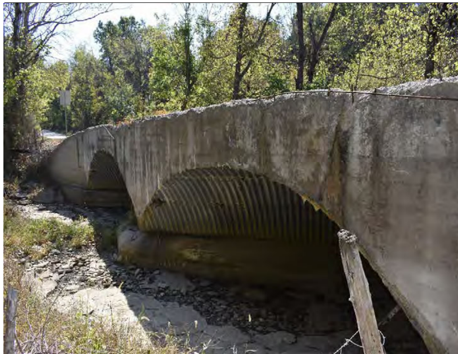
Photo 7: Downstream profile (east elevation) of Bridge No. 003B00041N.
