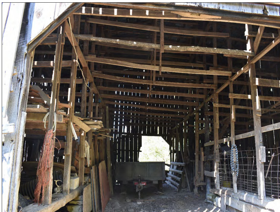
Photo 5: Facing north toward barn interior.
