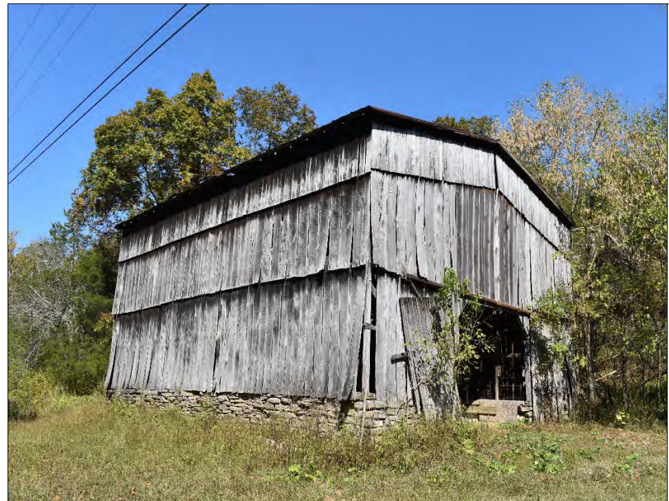
Photo 3: South and west elevations of barn at 0 McDonald Road.
