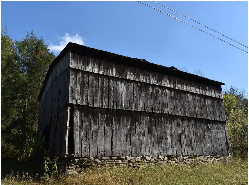
Photo 2: West elevation of barn at 0 McDonald Road.
