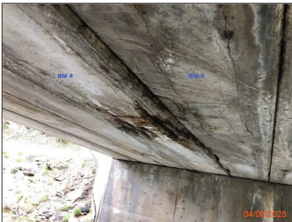
Figure 7. Evidence of failure to beams in Span 2. Image courtesy of the KYTC bridge inspection report for Bridge No. 007B00064N (BL-391).
