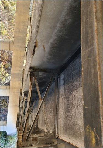
CROSSFRAME DAMAGE
