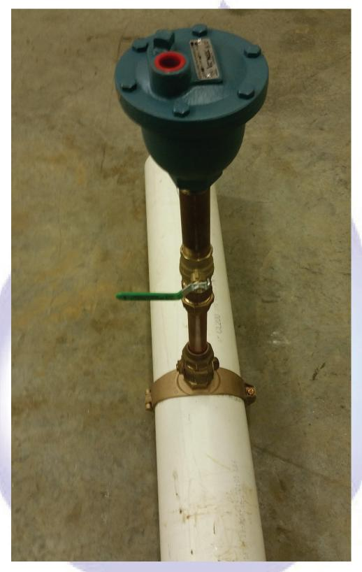
Air release Valve with Shut Off
