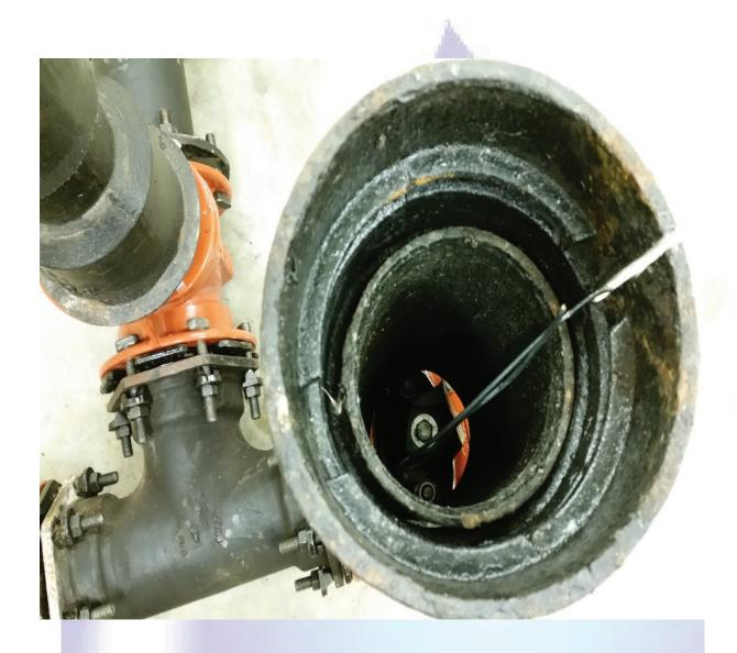
8 to 12in of tracer wire folded inside of valve box
