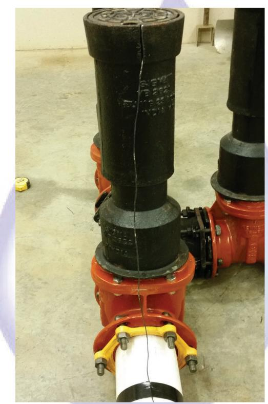
Taped 12in out from flange, tracer wire ran up outside of valve box
