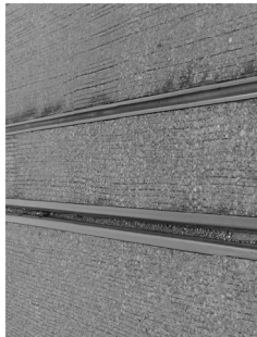
End Bent 2 Joints
