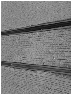
End Bent 1 Joints
