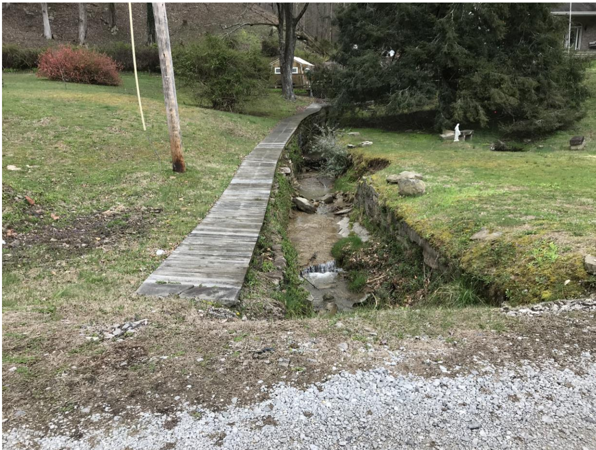
Mill Branch channel looking east
