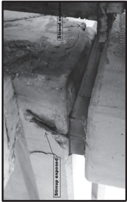
Pier 13, Span 12 Beam 1, 3, 4 & 5. 14'-0" Longitudinal U & 10' Vertical U.
