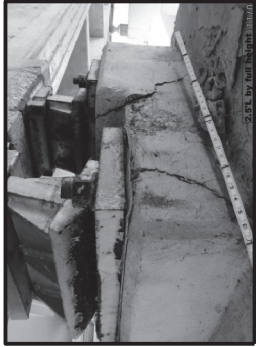
Pier 4: Span 3 ~ Beam 3. Span 4 ~ Beam 2. 9' Long Complete Wrap x 2.
