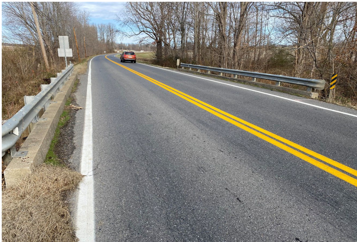
1 - IMG_2749 Bridge Surface - Facing N.JPG
