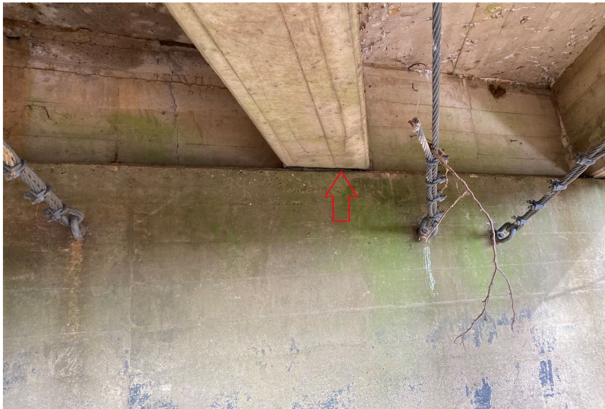
3 - IMG_2776 Horizontal Abutment Joint - Facing NE - Sample I-10128-1.JPG
