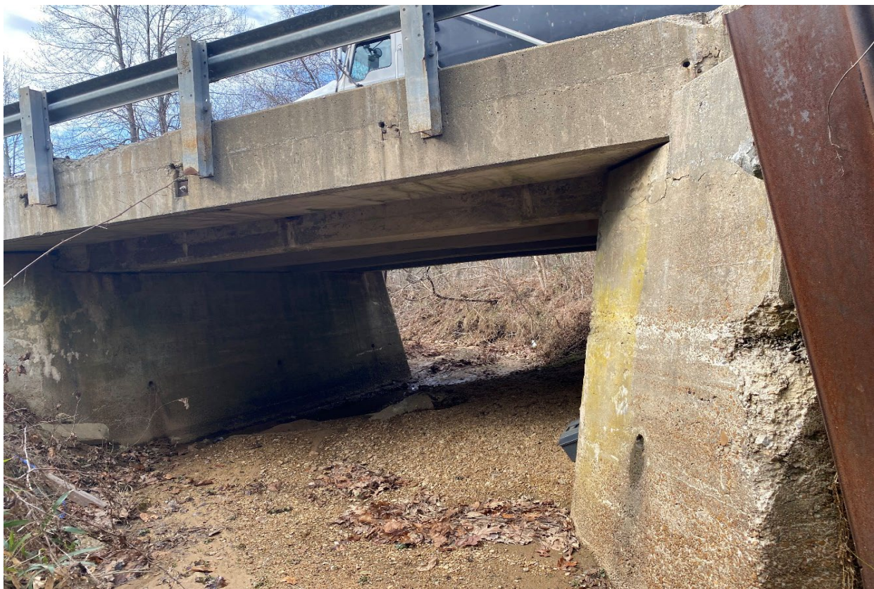
2 - IMG_2746 Bridge Below Deck - Facing W.JPG
