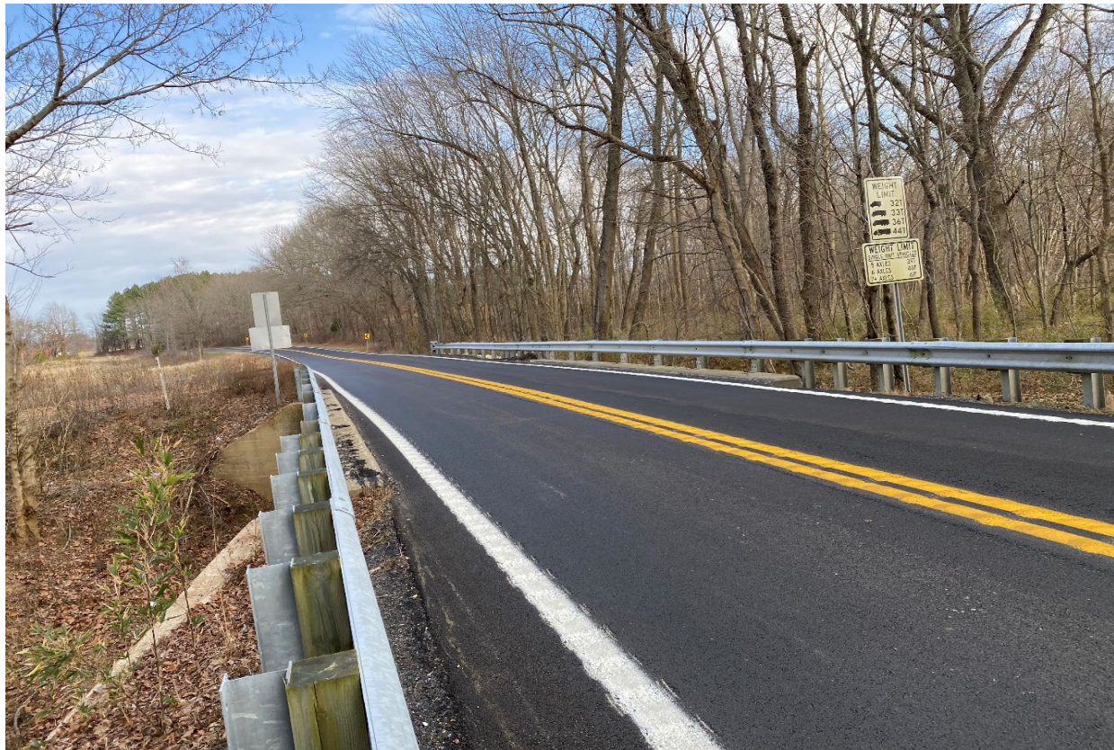
1 - IMG_2774 Bridge Surface - Facing NE.JPG
