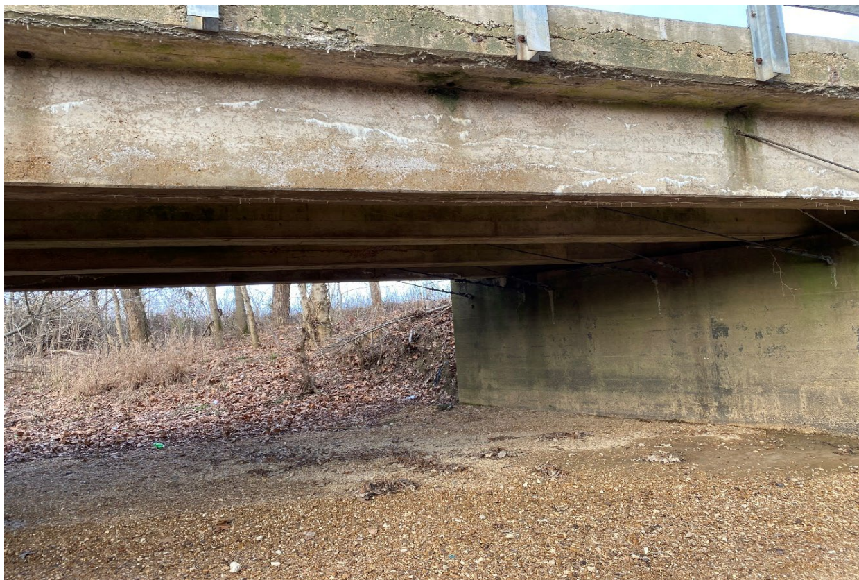
2 - IMG_2775 Bridge Below Deck - Facing N.JPG
