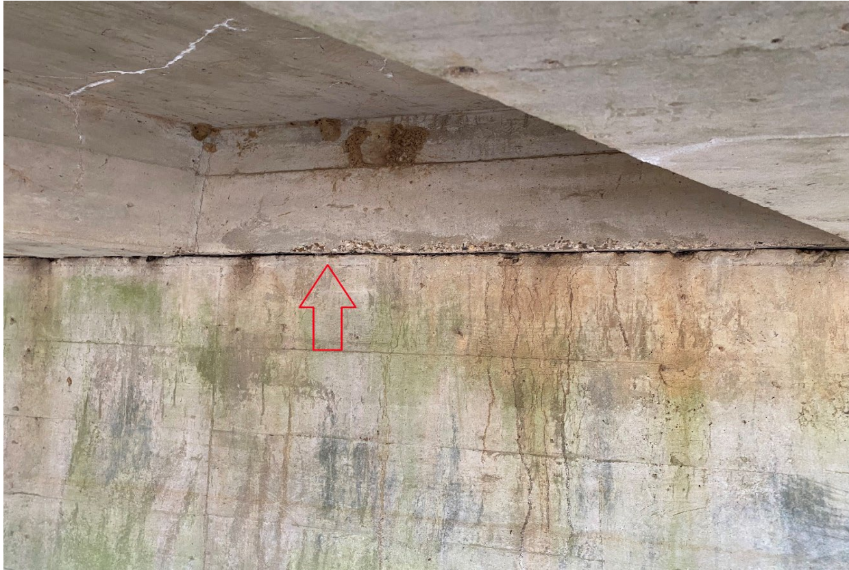
3 - IMG_2751 Abutment Joint - Facing S - Sample I-10104-1.JPG
