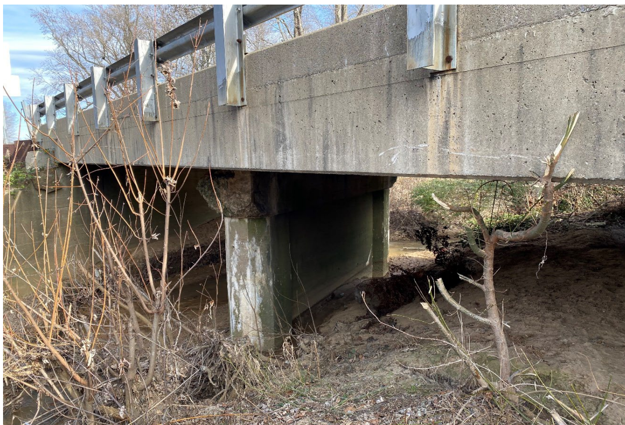
2 - IMG_2750 Bridge Below Deck - Facing N.JPG
