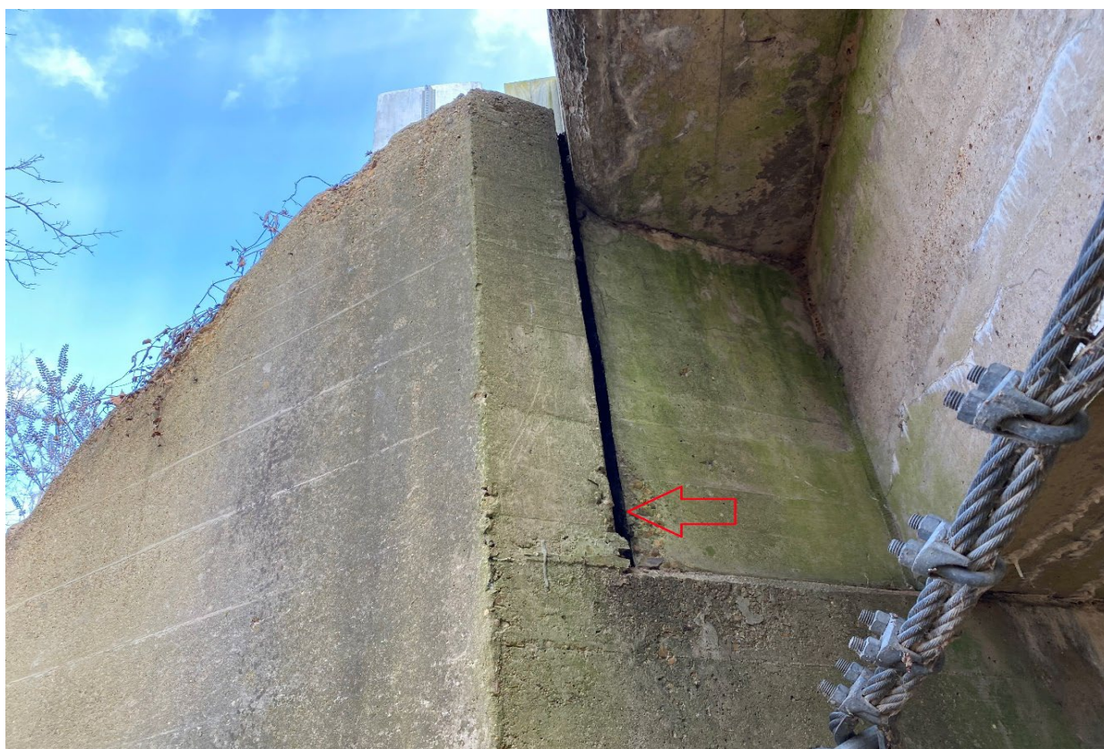
4 - IMG_2777 Vertical Abutment Joint - Facing NE - Sample I-10128-2.JPG
