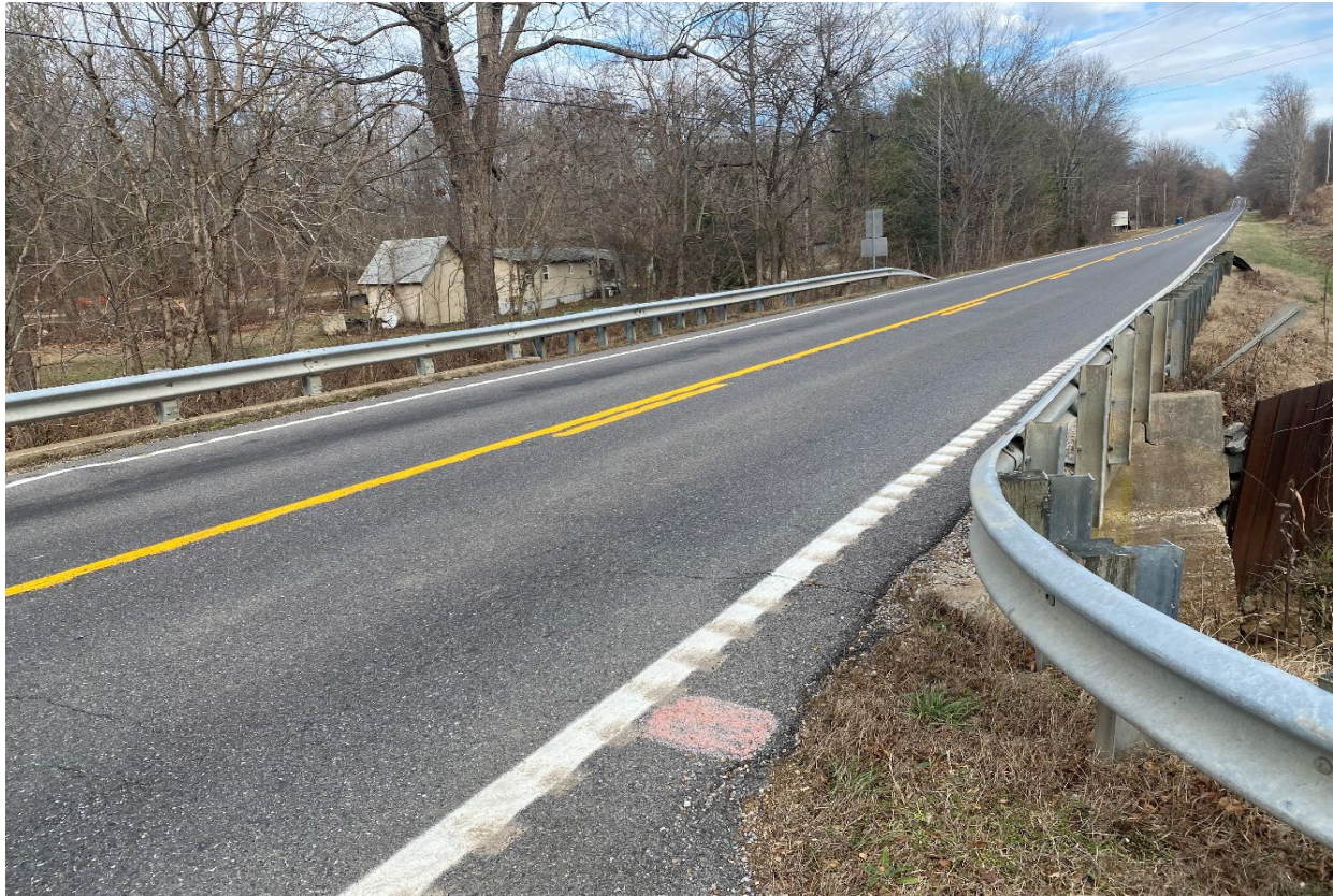
1 - IMG_2745 Bridge Surface - Facing N.JPG
