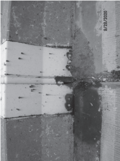
EXISTING EXPANSION JOINT STRIP SEAL AT PIER 8 BARRIER
