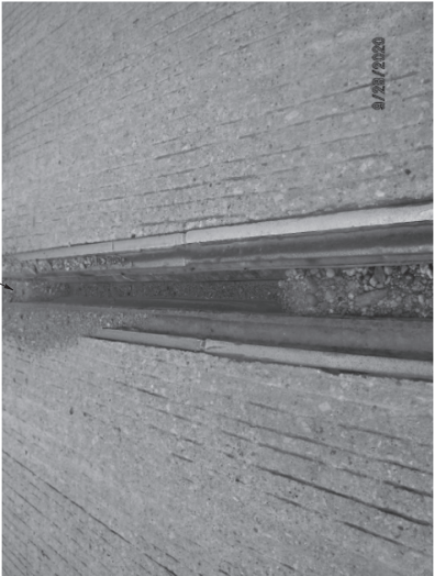
EXISTING EXPANSION JOINT STRIP SEAL AT PIER 8
