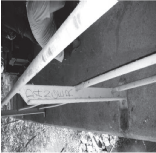
FAILED ANCHOR BOLTS AT SAFETY RAILING
