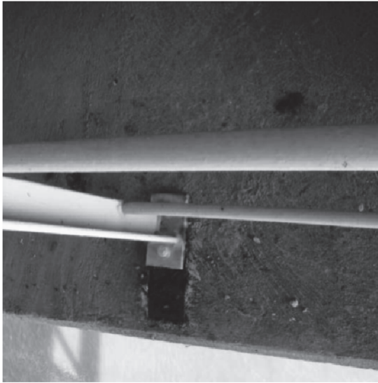
FAILED ANCHOR BOLTS AT SAFETY RAILING
