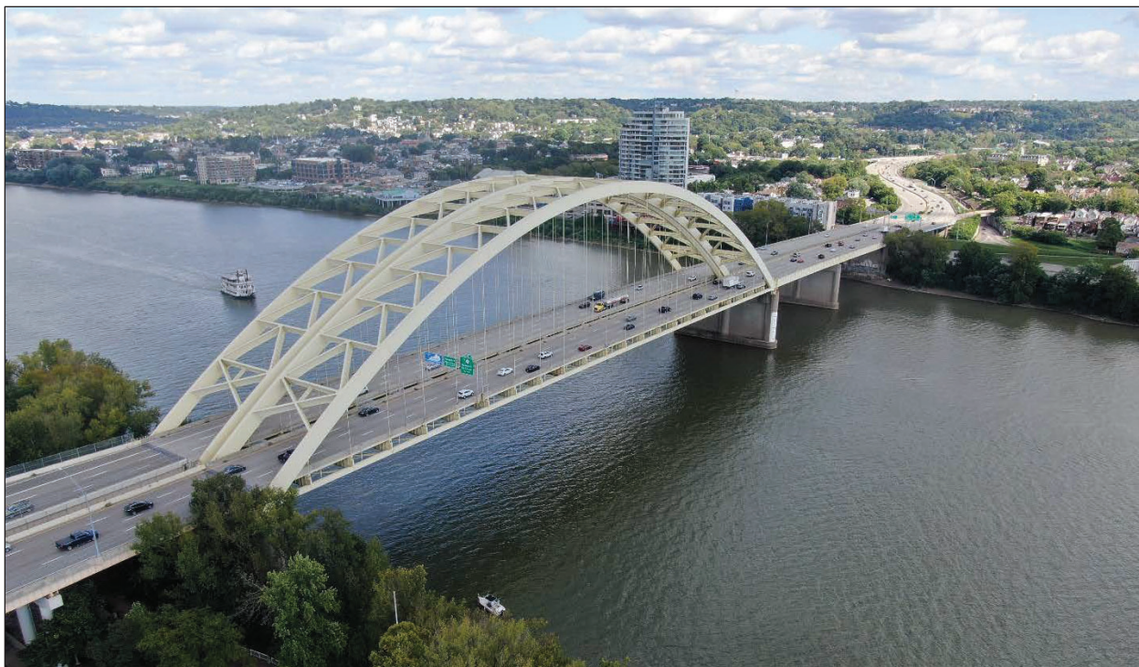
Figure 2. Project overview, showing the Daniel Carter Beard Bridge (DEBB), also known as the Big Mac Bridge, facing southeast. The DEBB is a twin span steel bowstring arch bridge which carries Interstate 471 across the Ohio River and was opened to traffic in 1976. The bridge is named for Daniel Carter Beard, founder of the Boy Scouts of America and Covington, Kentucky resident. Photograph by Palmer Engineering.
