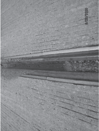
EXISTING EXPANSION JOINT STRIP SEAL AT PIER 8
