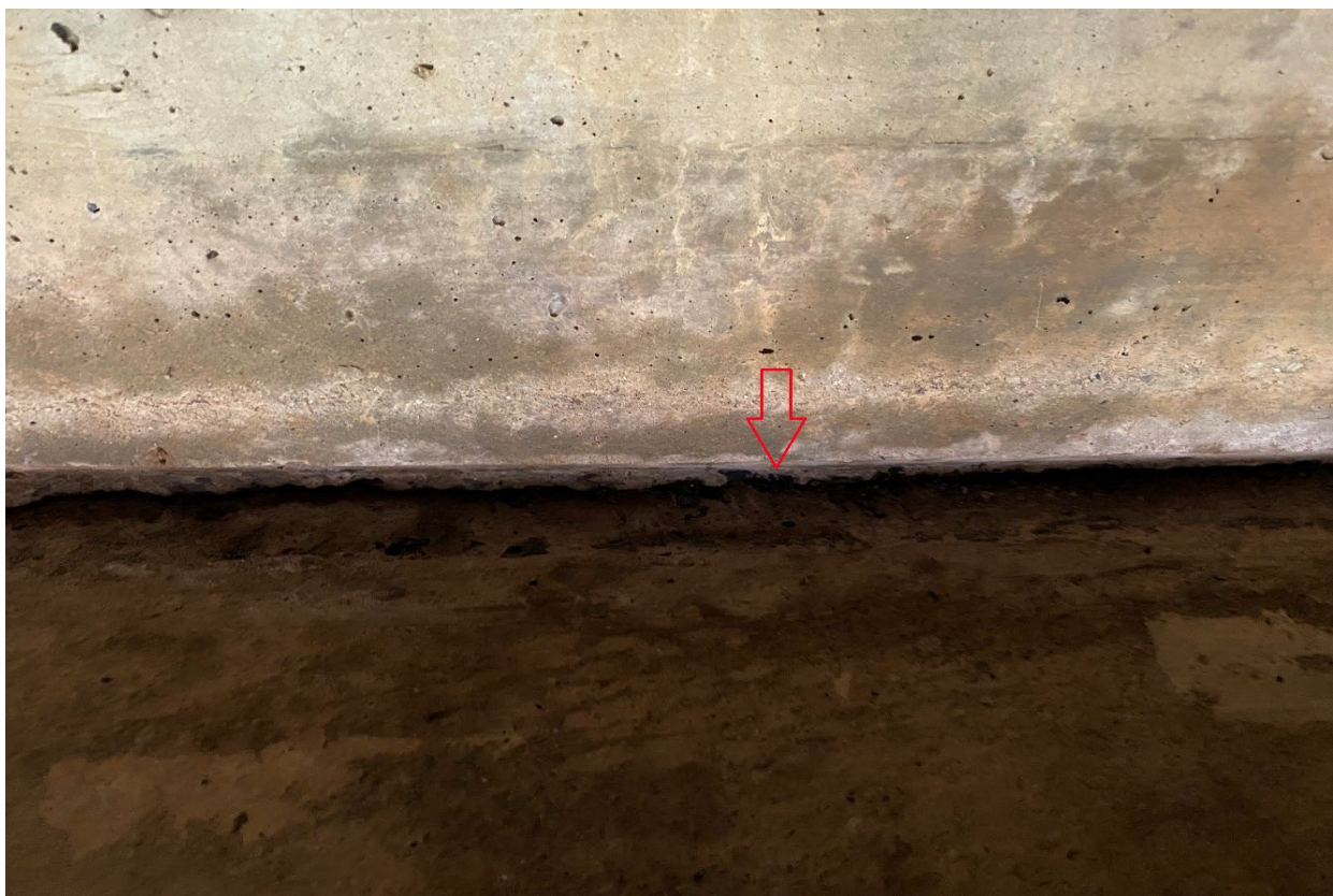
4 - IMG_2728 Horizontal Abutment Joint - Facing N - Sample I-10101-I.JPG
