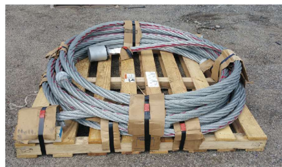
EXAMPLE SUSPENDER ROPE DELIVERED TO PROJECT SITE WITH RED STRIPE
