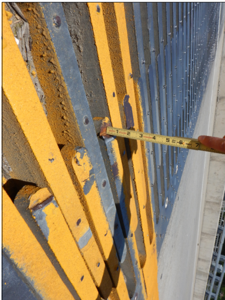
⑤ Damaged Finger Joint Repair Pier 6 Finger Joint: Grind the top of damaged fingers to provide smooth transition throughout joint prior to placing overlay.
