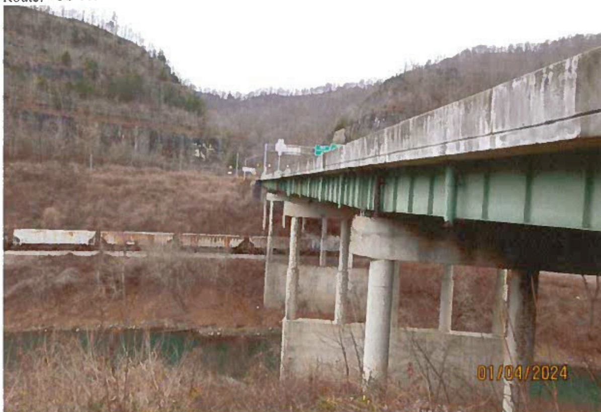
Downstream Profile looking from Abutment #1
